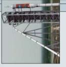
track to a safe area or bunker located inside the launch zone. A passive magnetic and friction braking system similar to those used on amusement-park on amusement-park rides decelerates the cabs. Total time from launchpad to bunker: about 88 seconds.
