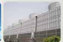
FIELD ERECTED, COUNTER FLOW, STEEL TOWER
