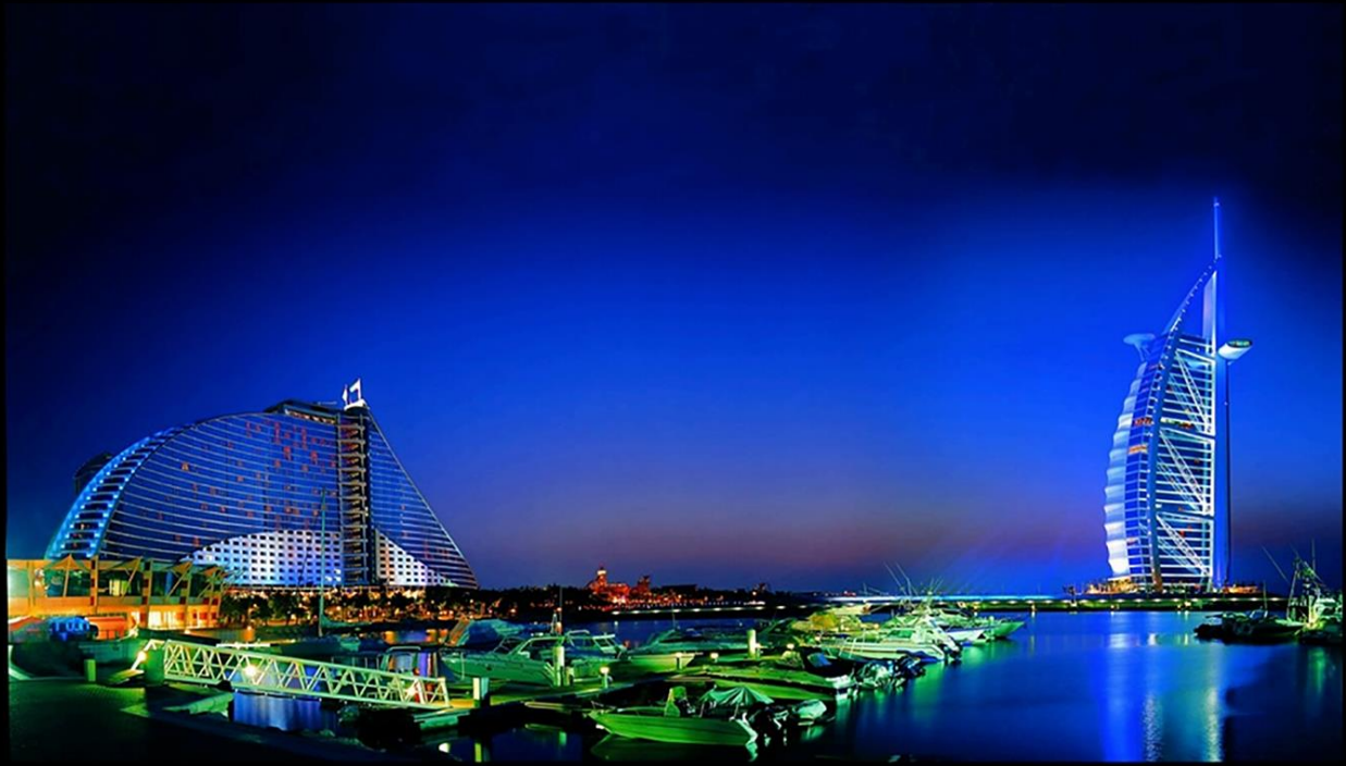
In 1993 Atkins was commissioned to design and construction manage the Jumeirah Beach Resort Development. They were asked to provide architectural design, structural engineering design, building service engineering design and civil engineering design. This slide show follows the Burj Al Arab from sketch to reality.
