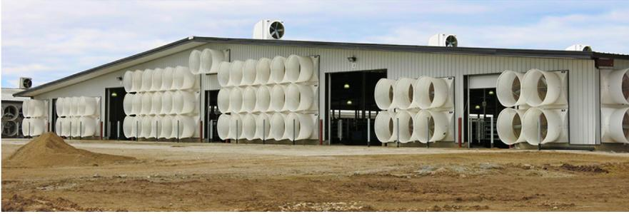
**Fig. 13.** A hybrid ventilation system with fans at the end-wall for summer ventilation and cupola fans for winter ventilation.
