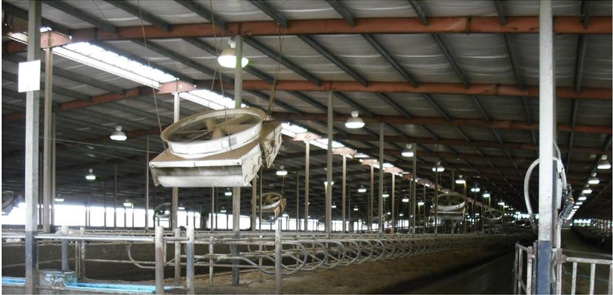
**Fig. 9.** Hybrid-ventilated barn with cyclone fans over the stalls to provide fast-moving air in the stall microenvironment and a closed ridge with a cupola system.
