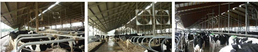
**Fig. 8.** Natural ventilation barns equipped with a panel fan every support post (*left*), 2 panel fans side by side over head-to-head stalls and a panel fan over single-row stalls every other support post (*middle*), and alternating fans every other support post over head-to-head stalls (*right*).
