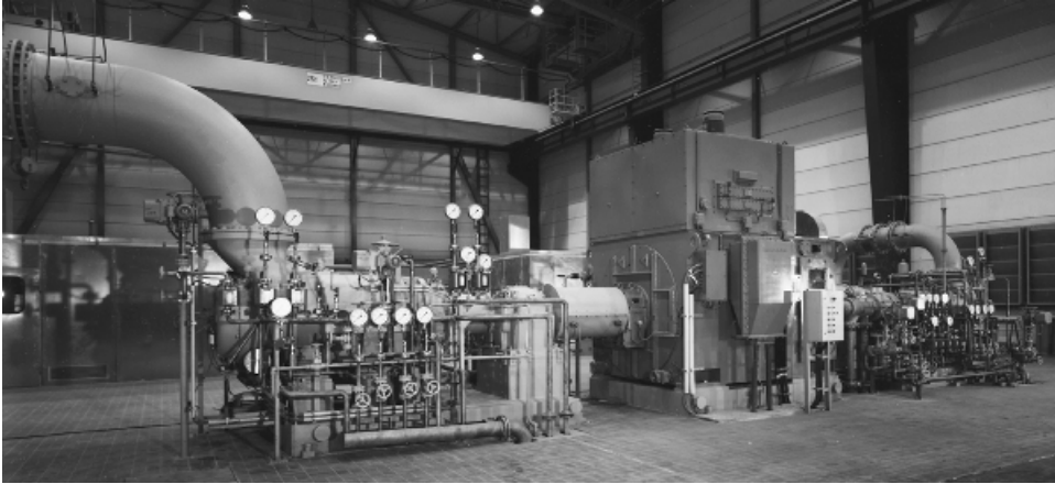
FIGURE 9.16 Large (approximately 7000 hp) rotary screw compressor installation at a German coal gasification plant. ( Aerzener Maschinenfabrik, Aerzen, Germany )
