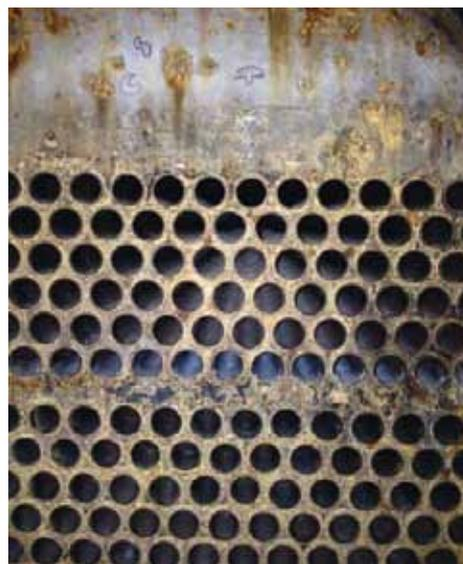
This Chiller is connected to a Cooling Tower which is exposed to lots of air borne contamination from surrounding farms.
