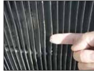
Silica is not removed by hosing, but can be pealed off with a nail.
