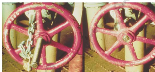
Color Plate 28 OS&Y Indicating Valves. (See Exhibit 13.7)
