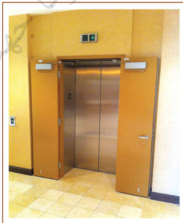
Exhibit 7.157 Permitted doors at entrance to elevator.
