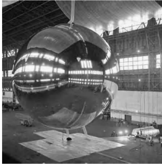
Figure 7.6 Echo 1 (1960) undergoing inflation tests. Courtesy of NASA.
