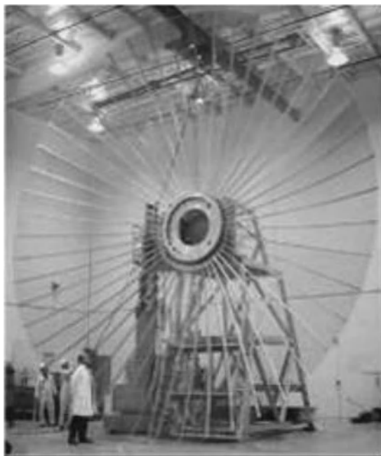
Figure 7.24 Lockheed wrap-rib antenna for NASA's ATS-6 (1974). Courtesy of NASA.
