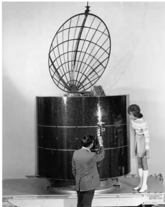
Figure 7.46 Telesat’s Anik A1 (1972) with first shaped beam antenna. Source unknown.
