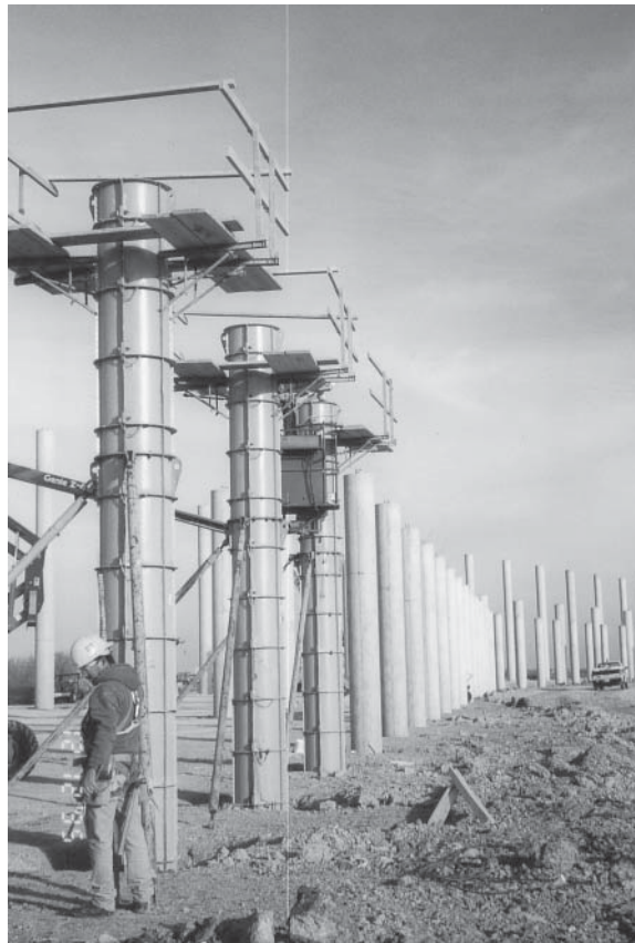
Round forms for grandstand support columns at the Texas Motor Speedway, Fort Worth, Texas.
