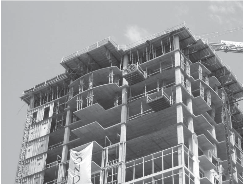
Flat Plate Construction—Pharr Road Condominiums, Atlanta, Georgia.
