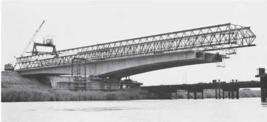
Prestressed concrete segmental bridge over the River Trent near Scunthorpe, Lincolnshire, England.
