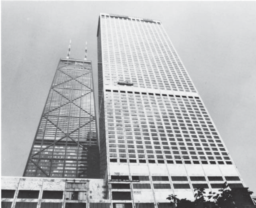
Water Tower Place, Chicago, Illinois, tallest reinforced concrete building in the United States (74 stories, 859 ft).
