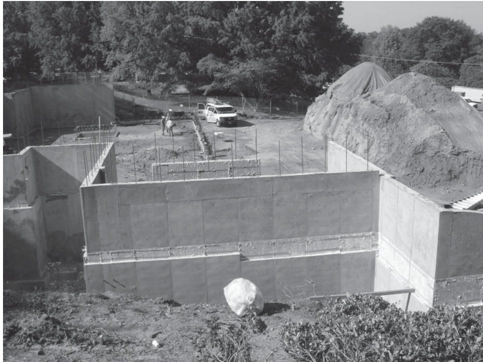
Retaining wall with stepped wall thickness.
