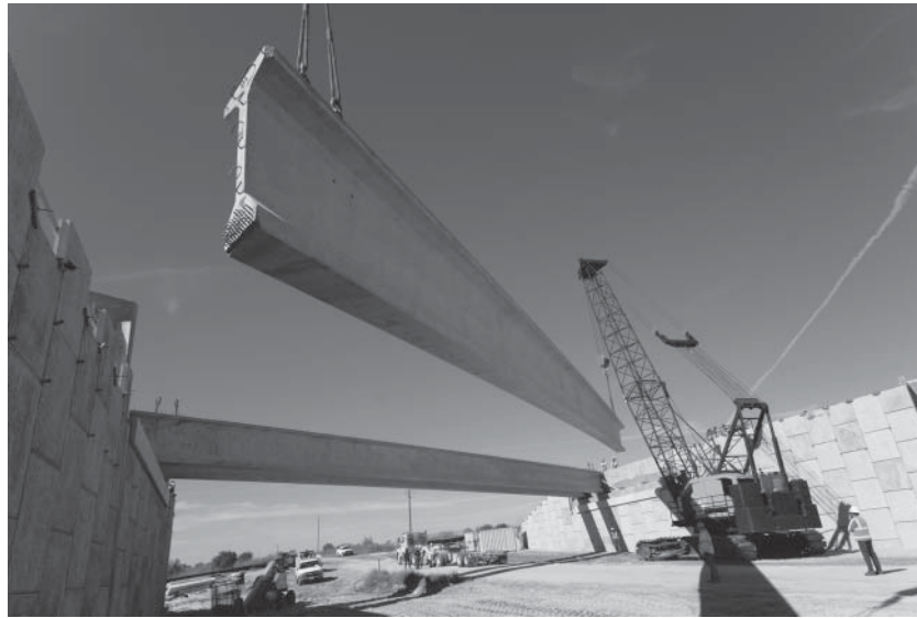
Prestressed bridge girders during erection.
