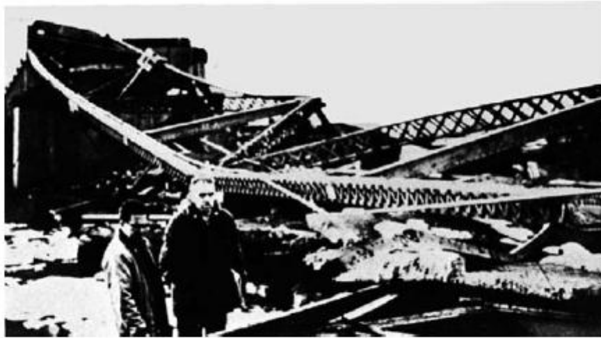
Fig. 1.3 On December 15, 1967, the Silver Bridge connecting Ohio and West Virginia over the Ohio River collapsed, and 46 people lost their lives. The cause of the collapse was stress-corrosion cracking [3]
