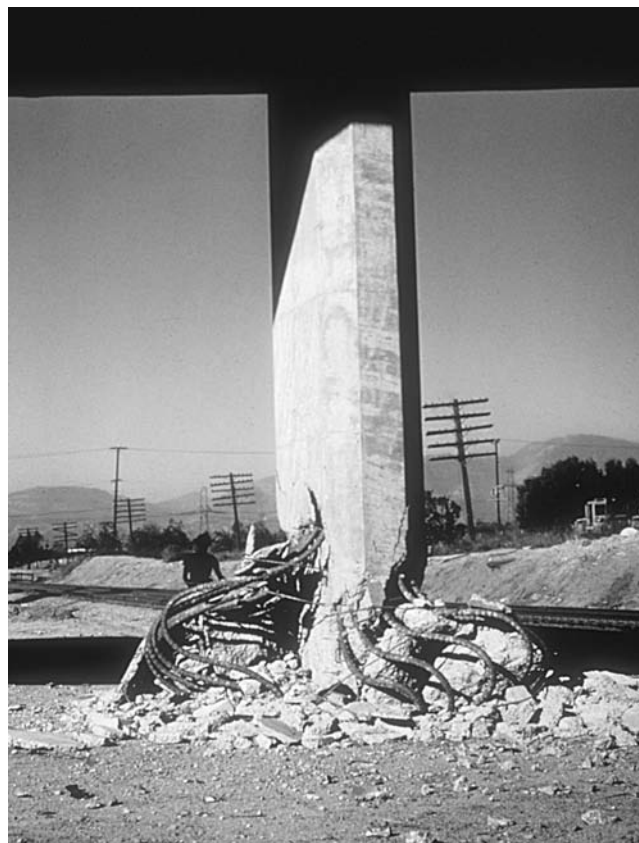
Crushing of the base of a column in an overpass during the 1971 San Fernando earthquake. The damage done to the column is characteristic of that done by a Rayleigh wave. The motion of the ground is like an ocean wave. The return upward motion causes the crushing because it is held in place by the overpass. (Courtesy of the USGS)
