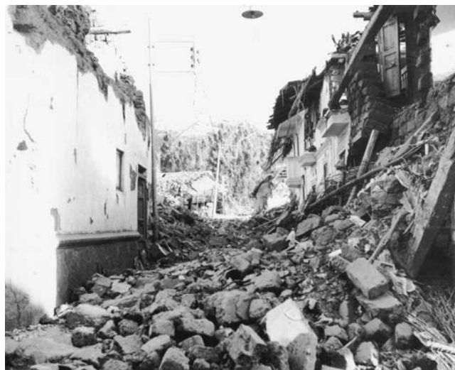
Massive destruction of adobe houses in the town of Huez during the 1970 earthquake, by far Peru's worst natural disaster (Courtesy of the USGS)
