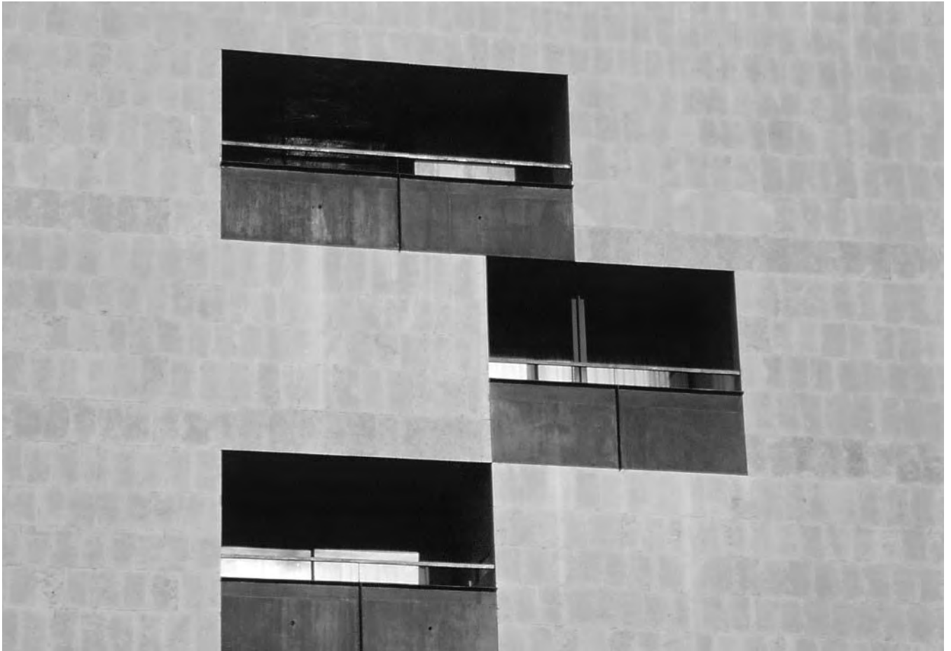
6.10 Alejandro de la Sota, Civil Government building, detail, Tarragona, 1961.
