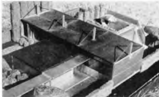
Prefabricated "one plus two" expandable dwellings of Diatom construction.
