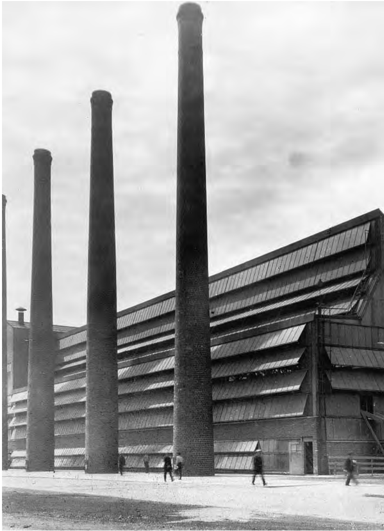
1.1 Albert Kahn, Ford Motor Company, glass plant, Detroit, 1922.
