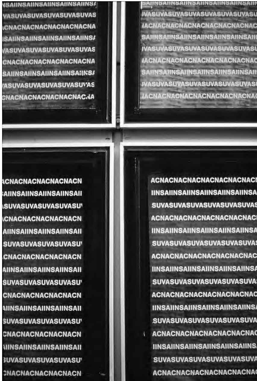
P.6 Herzog and de Meuron, Suva Building, Basel, 1993.
