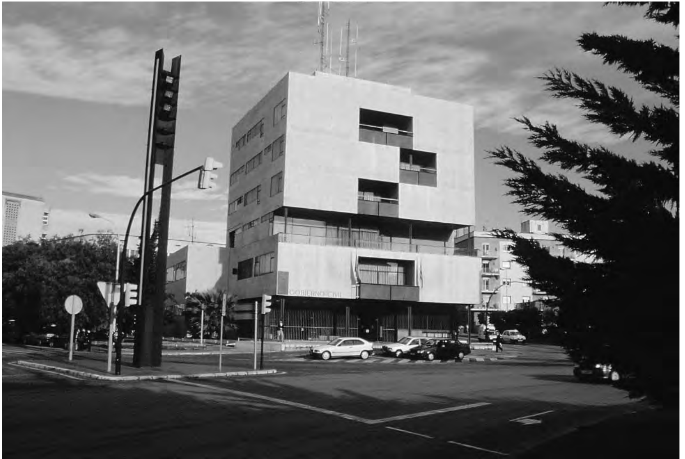
6.9 Alejandro de la Sota, Civil Government building, Tarragona, 1961.
