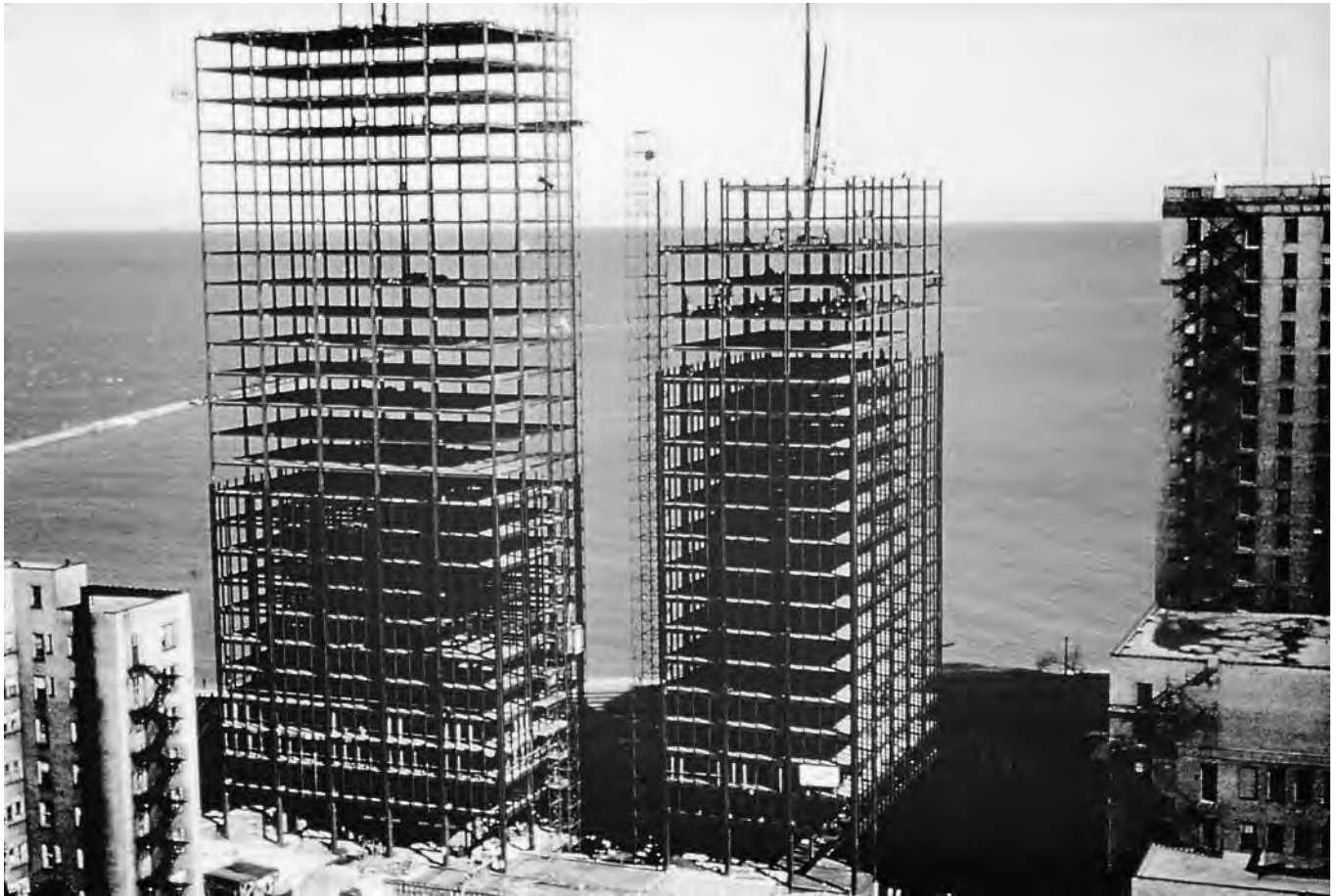
4.14 Ludwig Mies van der Rohe, Lake Shore Drive apartments, under construction, Chicago, 1950.
