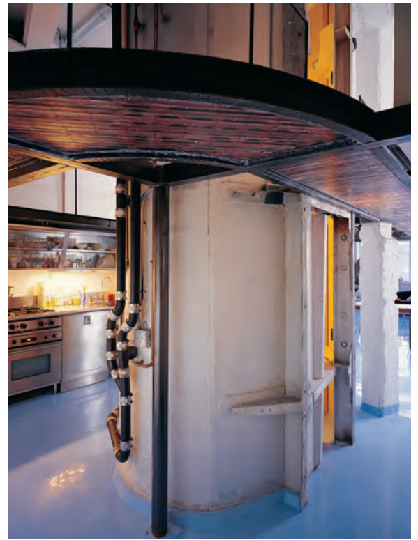
LOT/EK, Morton Residence, New York, 1999. A used petroleum trailer tank was hoisted into this loft, then cut in two sections, one placed vertically and fitted out as a bathroom with a bright yellow interior. The twin section is converted into a sleeping chamber.
