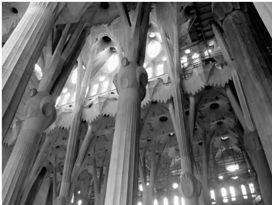
Figure 6.55. Some of the vaults of La Sagrada Família. Photo by Sarika Bedi
