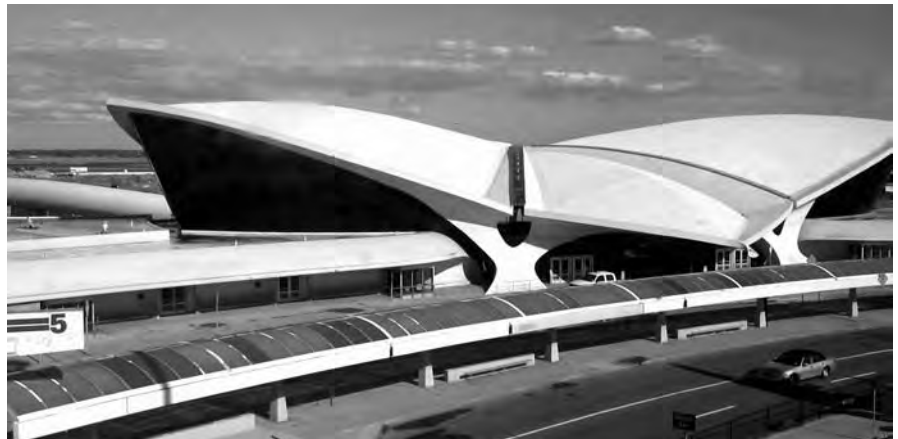
Figure 7.29. Saarinen's terminal at JFK showing three of the four vaults and two of the Y-shaped columns. Photo by Pheezy
