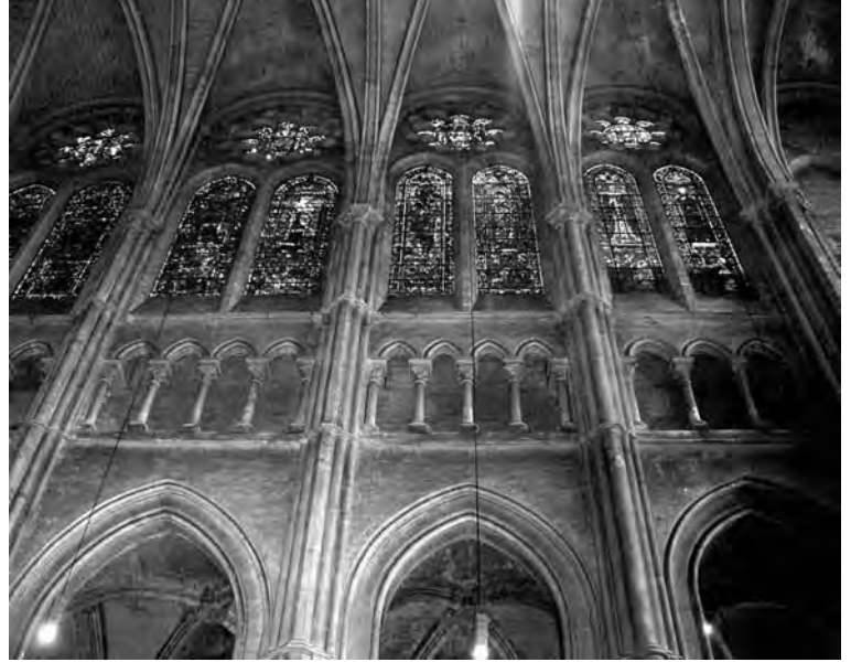
Figure 3.22. Sets of three converging ribs along with supporting columns. Photo by BjörnT
