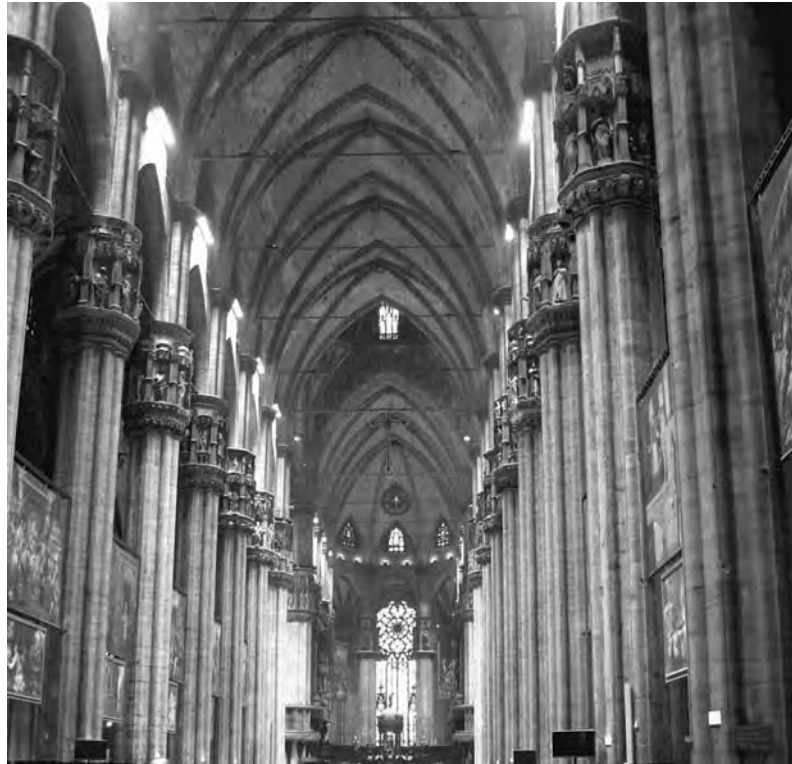
Figure 3.29. Some of the main piers of the nave with capitals and iron binding rods, and Gothic vaulting of the Milan Cathedral. Photo by Giovanni Dall'Orto
