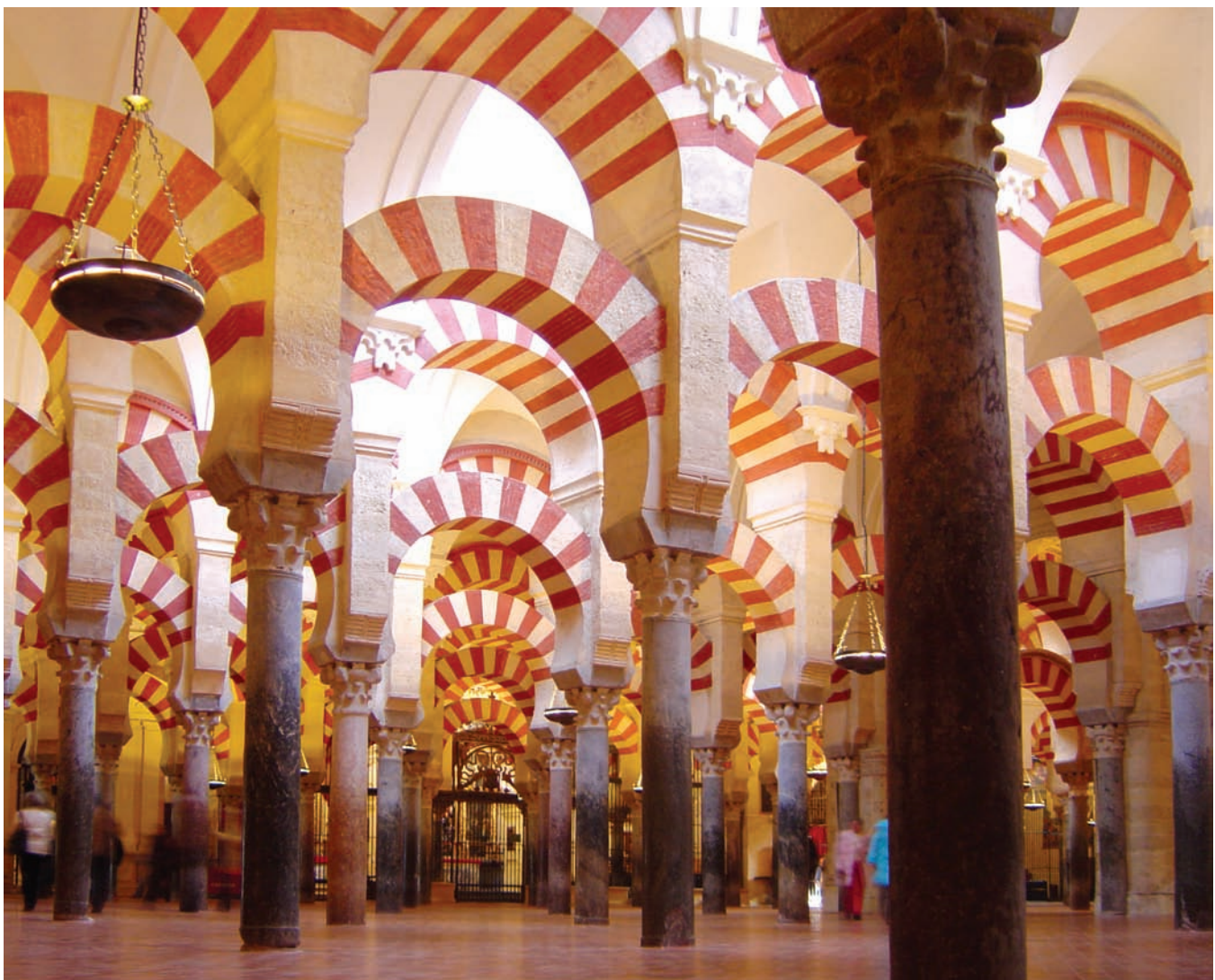
Plate 8. Rows of double arches define the vast prayer hall of the Great Mosque of Córdoba. Photo by Timor Espallargas
