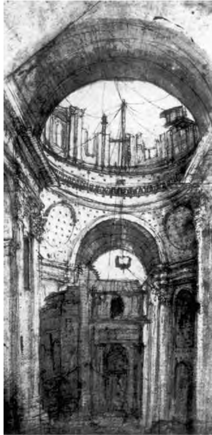
Figure 5.36. Giovanni Antonio Dosio, Michelangelo's drum under construction around 1562. (The structure Bramante built to protect the altar can be seen under the arching vault). From Charles B. McClendon, "The History of the Site of St. Peter's Basilica, Rome," Perspecta , vol. 25, 1989
