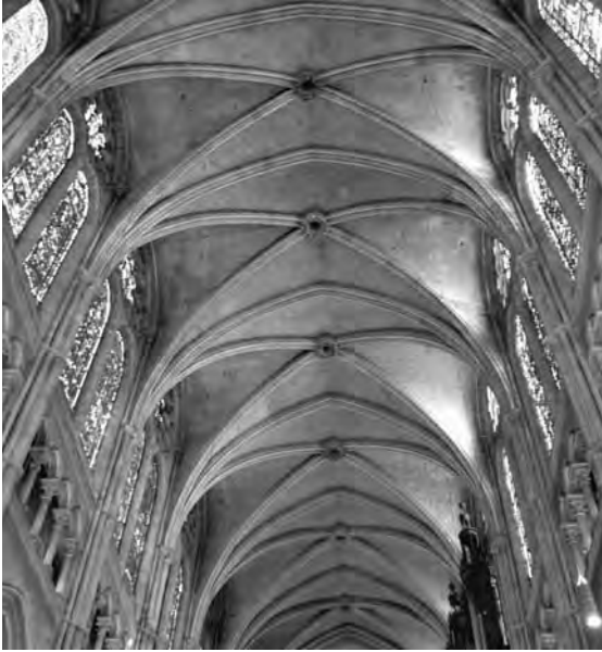
Figure 3.21. Ribbed vaults over several bays in the ceiling of a Gothic cathedral. Photo by Magali Ferare
