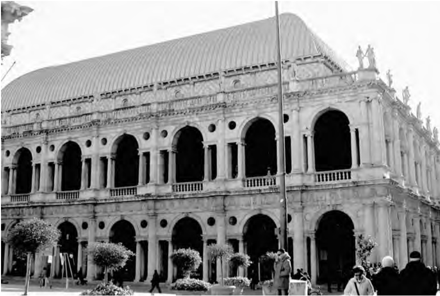
Figure 5.14. Palladio's shell for the basilica of Vicenza, a medieval market and council hall, 1549. Photo by GvF
