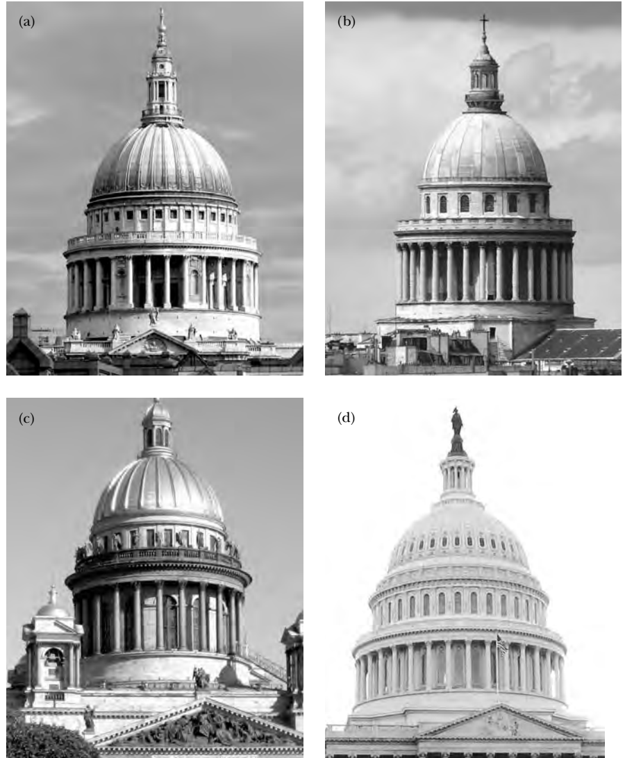
Figure 6.1. The domes of (a) St. Paul's in London (1705–1708) photo by Bernard Gagnon, (b) the Panthéon in Paris (1775–1781) photo by Siren-Com, (c) St. Isaac's in Saint Petersburg (1840–1842), (d) the Capitol Building in Washington (1856–1864), photo by Túrelío
