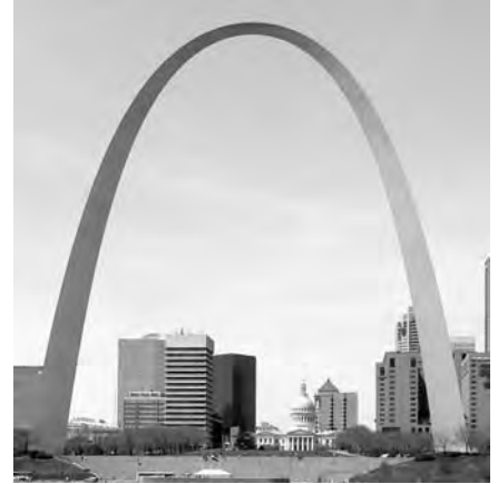
Figure 7.20. The Gateway Arch in St. Louis. Photo by Bev Sykes
