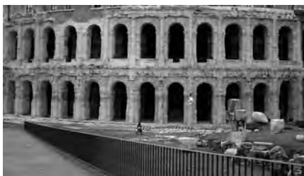
Figure 2.36. Remaining wall structure of the Theater of Marcellus, Rome. Photo by Joris van Rooden
