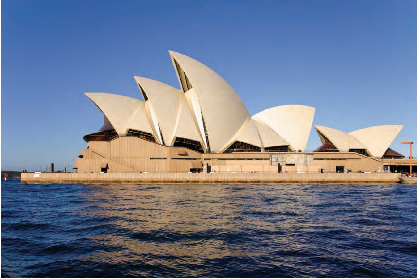
Plate 24. Shell and podium structure of the Sydney Opera complex. Photo by Matthew Field
