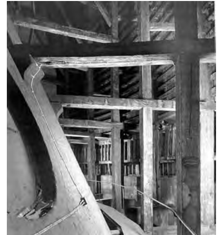
Figure 6.3. Inner timber structure resting on the brick cone in support of the outer dome. Conway Library, The Courtauld Institute of Art, London. Photo by A. F. Kersting
