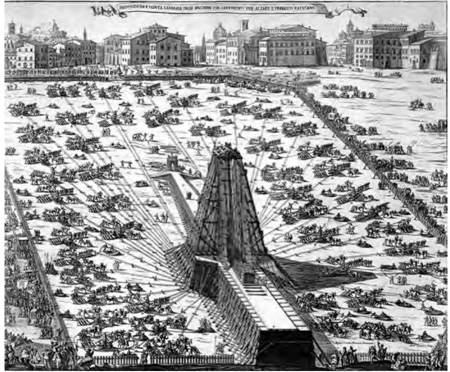
Figure 5.70. Natale Bonifacio, illustration for Domenico Fontana's manuscript Della Transportatione dell' Obelisco Vaticano , 1590. Marquand Library of Art and Archaeology, Princeton University Library
