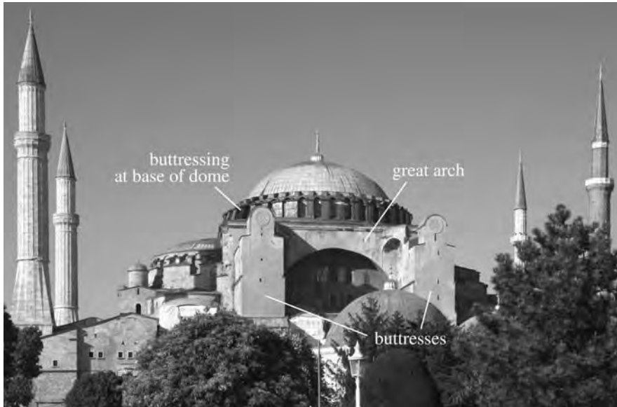
Figure 3.5. Today's Hagia Sophia from the south. The four spires are minarets added after the conversion of the church to a mosque. Photo by Terry Donofrio
