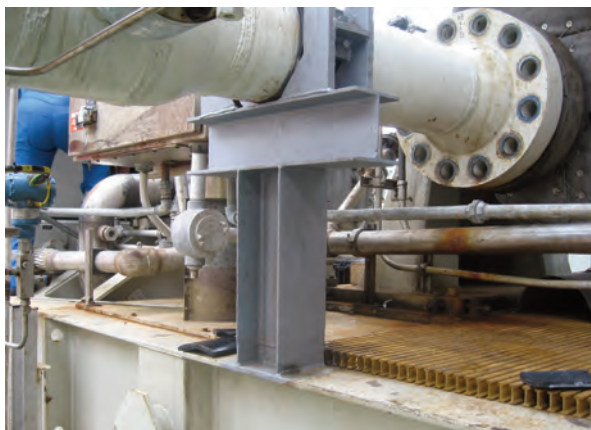
Figure 18. Check for Pipe Strain.
