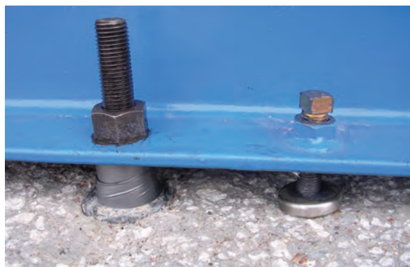
Figure 6. Anchor Bolts and Leveling Jackscrew.
