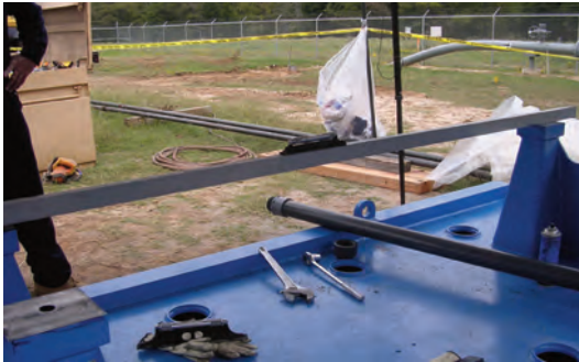
Figure 9. Base with Straightedge and Machinist Level.
