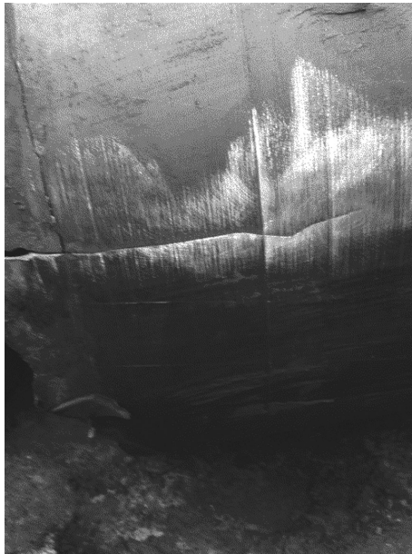
FIGURE 15.8 Longitudinal crack propagating and ending at the end plate.
