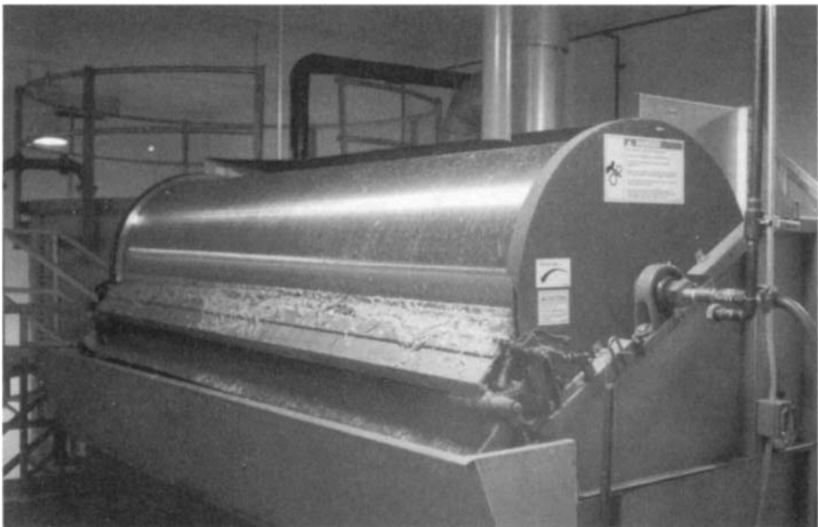
Figure 7-66 Rotating cylindrical screen (courtesy of Hycor).
