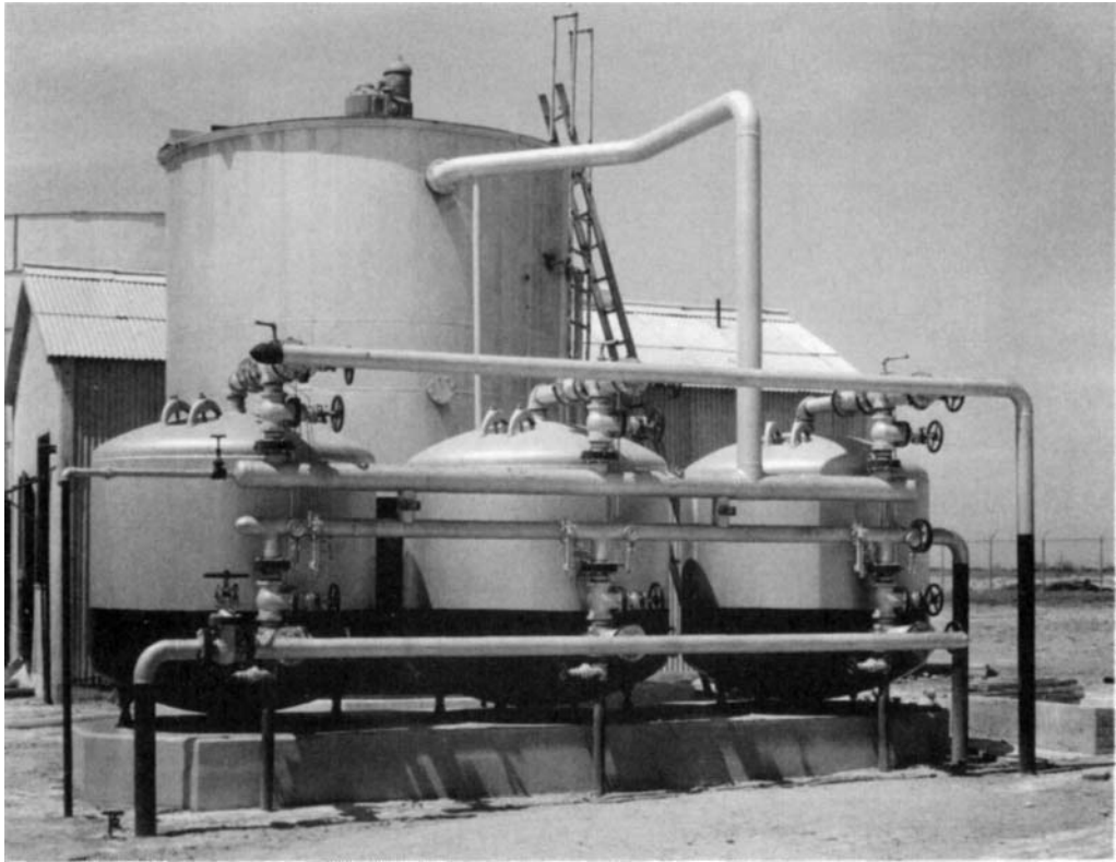
Figure 7-78 Pressure and vacuum filters. (a) Courtesy of IDI/Infilco Degremont, Inc.
