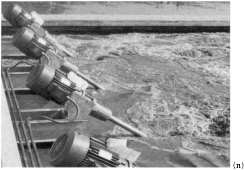
Figure 7-40 Alternative types of devices for aeration: (m) pontoon-mounted, aspirating aerator (courtesy of Eimco Process Equipment, a Baker Hughes Company); (n) fixed-mounted, aspirating aerator (courtesy of Eimco Process Equipment, a Baker Hughes Company).
