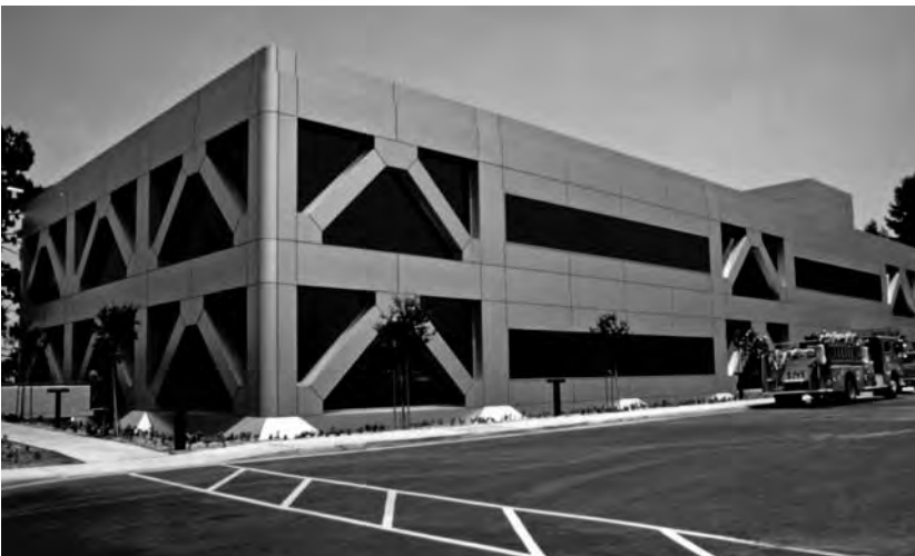
Figure 1.7 Fire Command and Control Facility, Los Angeles, California. Courtesy of James M. Kelly, NISEE Online Archive, University of California, Berkeley
