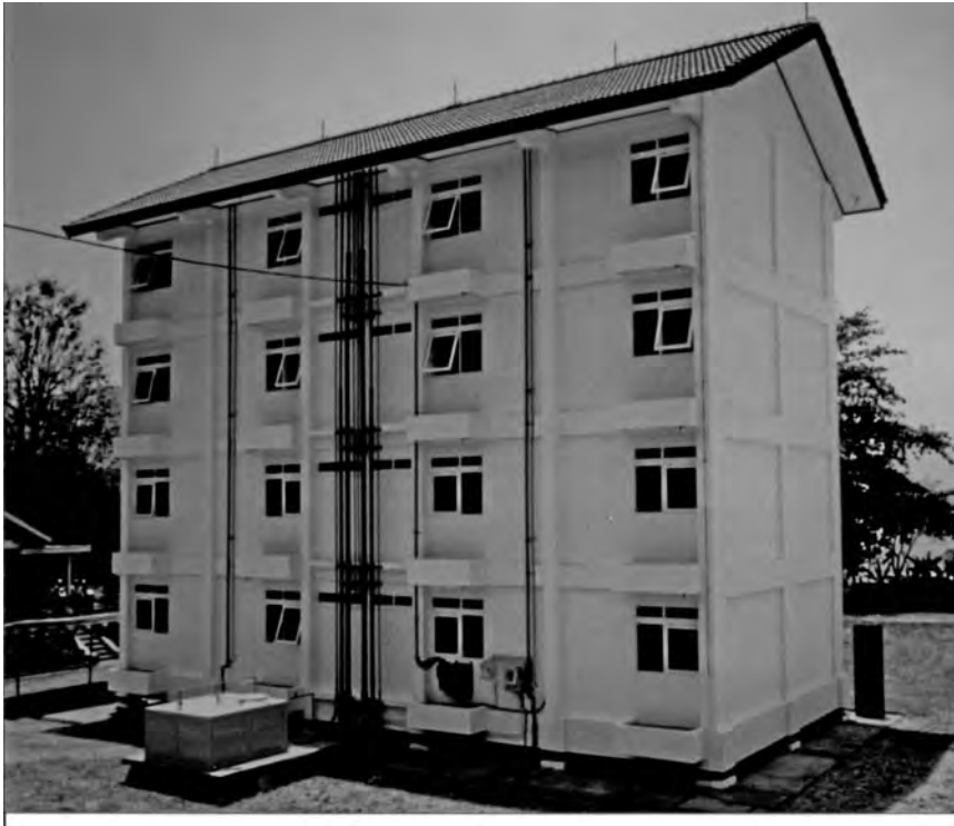
Figure 1.13 Demonstration building in Pelabuhan Ratu, West Java, Indonesia. Courtesy of James M. Kelly. University of California, Berkeley
