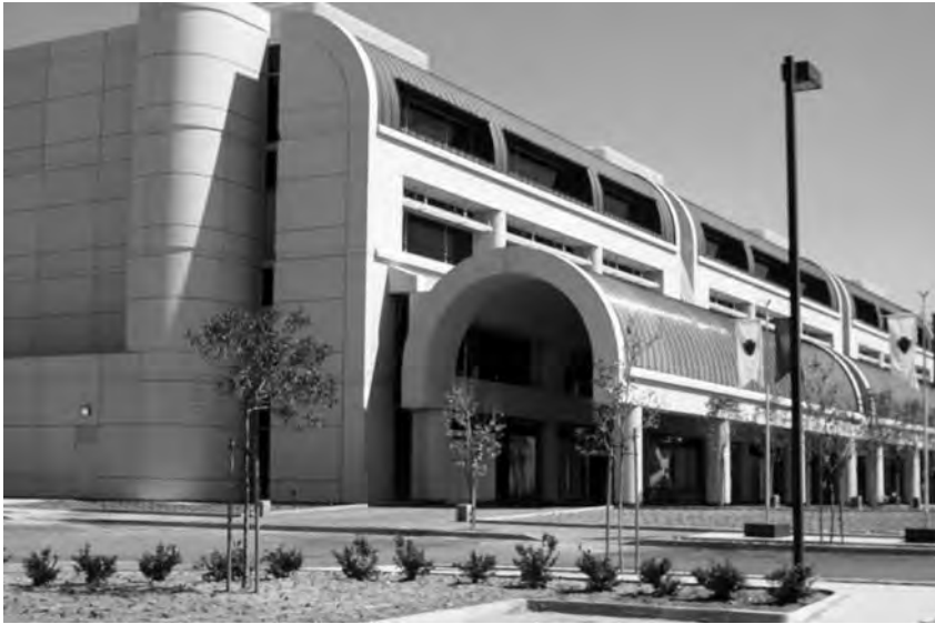
Figure 1.5 Foothill Communities Law and Justice Center, Rancho Cucamonga, California. Courtesy of James M. Kelly. NISEE Online Archive, University of California, Berkeley
