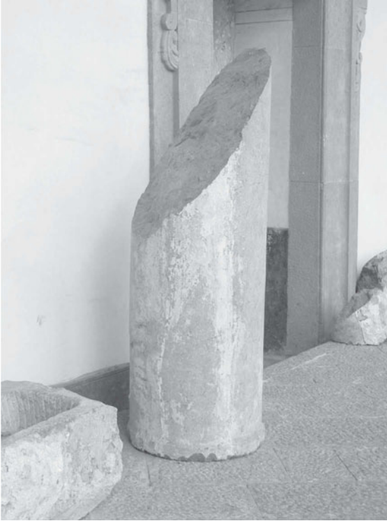
Figure 1.31. An ancient stone column ('cortile di Palazzo Bonet', Via S. Anna, 21 Palermo, Italy) evidencing a typical failure mode in compression through localisation of damage (compare with Fig. 1.10).
