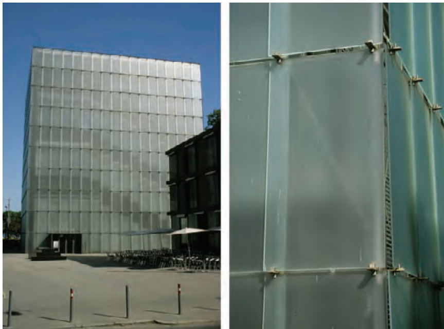
4.39 Glass “wrap” facade (left) and close up of glass panels (right) used as shingles and hung from the facade of the Kuntshaus Art Gallery in Bergenz, Austria. DONALD CORNER
