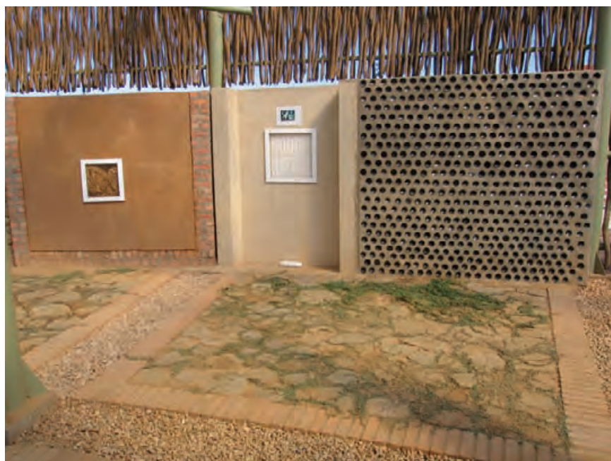
5.60 A sample wall at HRDC demonstrates the use of a variety of appropriate materials and construction techniques. HEIDI SPALY
