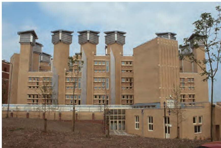
4.166 Stack ventilation towers exhaust warm air at Lanchester Library at Coventry University, Coventry, UK.
