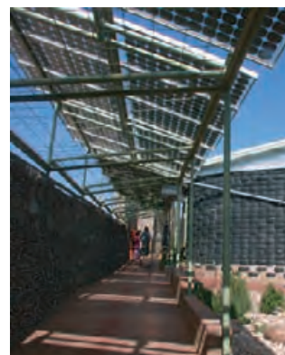
5.59 Photovoltaics as shading devices along walkway. NINA MARITZ
