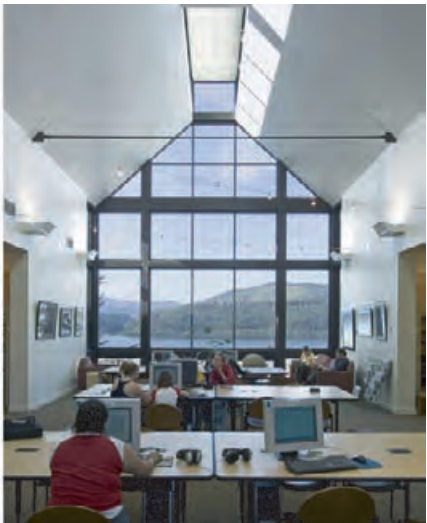
4.74 The Hood River Public Library (left) in Hood River, Oregon uses daylight and natural ventilation strategies; a long, clerestory monitor (right) illuminates the main reading area in the Library addition. FLETCHER FARR AYOTTE, INC.
