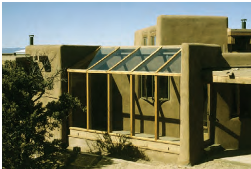
4.133 An adobe residence with an attached sunspace in Santa Fe, New Mexico.
