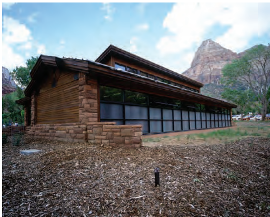
4.130 Zion National Park Visitor's Center in Springdale, Utah showing a Trombe wall and clerestory (direct gain) windows. ROBB WILLIAMSON, DOE/NREL
