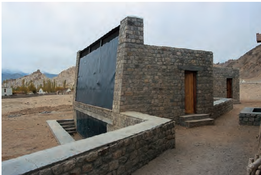
5.50 The latrine building with solar collector. CAROLINE SOHIE, ARUP + ARUP ASSOCIATES
