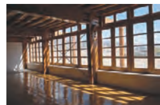
5.45 School rooms feature southeast-facing direct gain windows that ensure early morning warm-up in Shey's sunny climate. CAROLINE SOHIE, ARUP + ARUP ASSOCIATES
