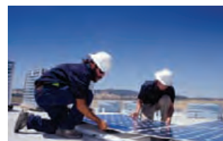
4.223 Installation of lightweight, interlocking photovoltaic panels.
