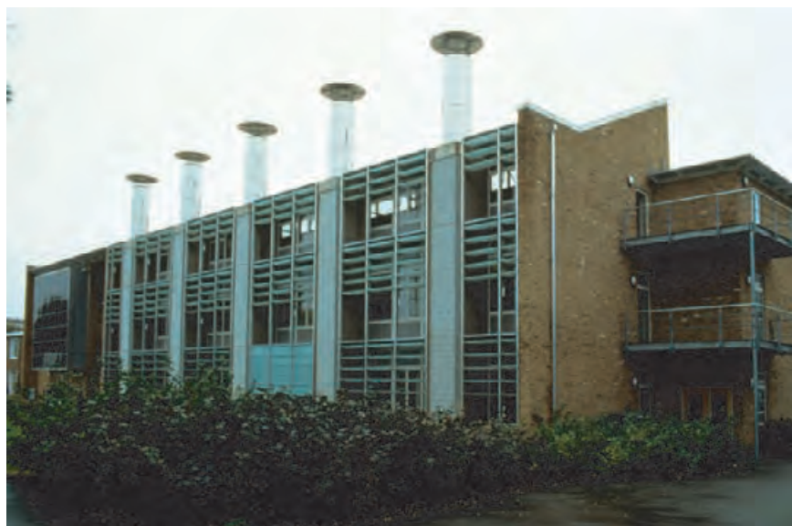
4.164 South facade features photovoltaic panels, solar chimneys (with glass block to assist) and a stack ventilated top floor at the Building Research Establishment offices, Garston, Hertfordshire, UK. THERESE PEPPER
