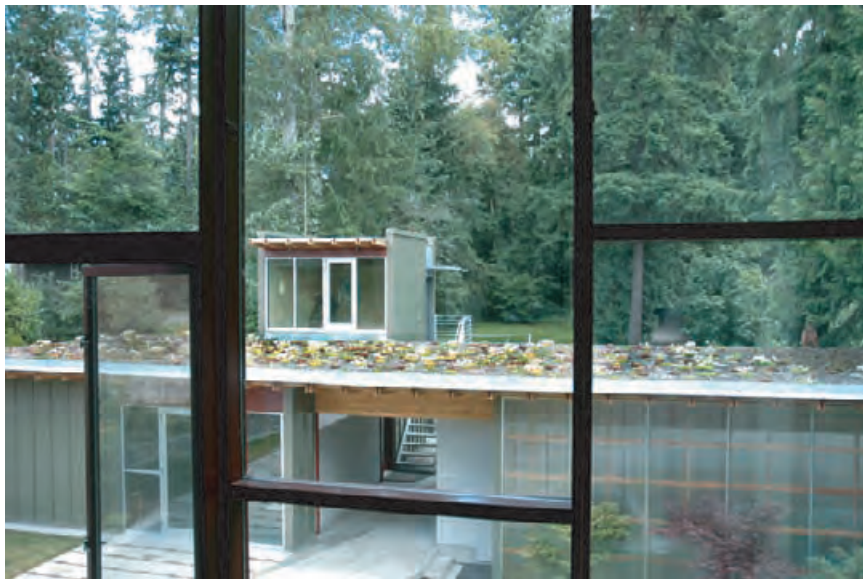
4.51 Green roof on the Roddy/Bale garage/studio in Seattle, Washington has a variety of native plants and ground cover. MILLER/HULL PARTNERSHIP
