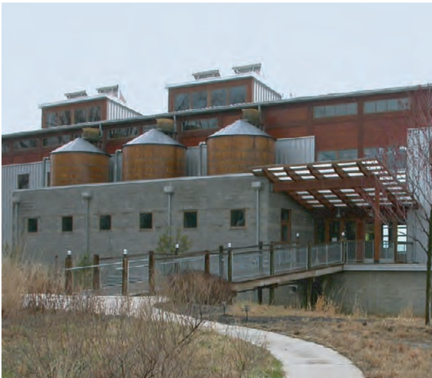
4.275 Cisterns assembled from recycled pickle barrels from a nearby factory are part of the highly-visible rainwater catchment system at the Chesapeake Bay Foundation in Annapolis, Maryland.
