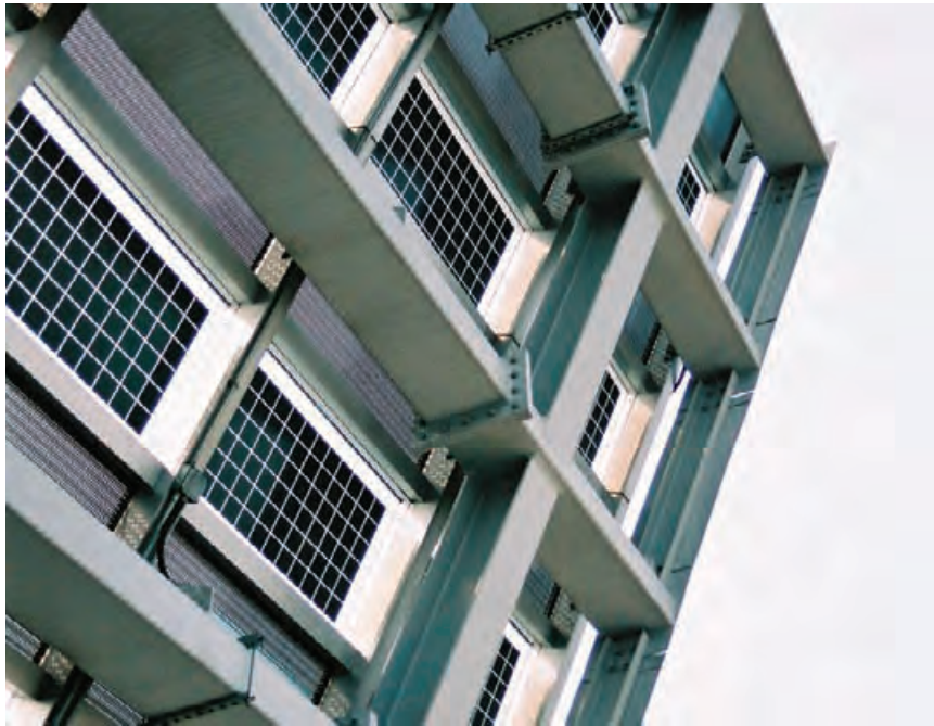
5.114 Building integrated photovoltaic cells laminated within the glazing are framed by a steel truss on the roof of the building. ROCCO DESIGN LTD.
