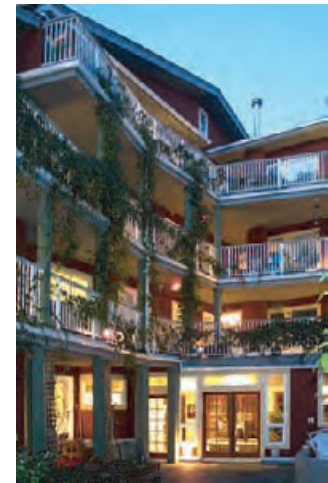
4.258 Quayside Village courtyard uses recycled water in North Vancouver, British Columbia, Canada. COHOUSING DEVELOPMENT CENTER
