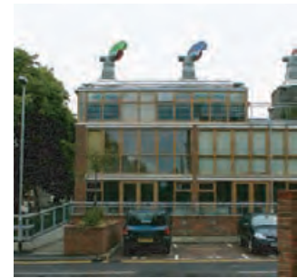
5.14 Southern facade of a residential unit at BedZED showing sunspaces and wind COWLS. BRUCE HAGLUND
