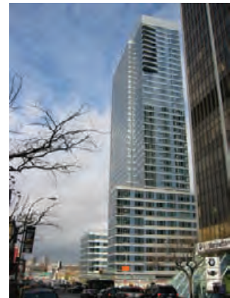
5.67 The massing of the 38-story building creates 7 corner apartments on each floor. FXFOWLE ARCHITECTS, PC
