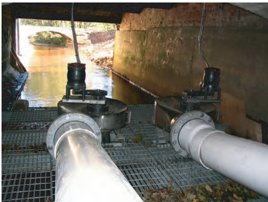
4.239 Looking downstream from two microhydro turbines at the Tanfield Mill in Yorkshire, England. The installation is part of an ongoing development in renewable energy projects focusing upon microhydro applications. NAUTILUS WATER TURBINE, INC.
