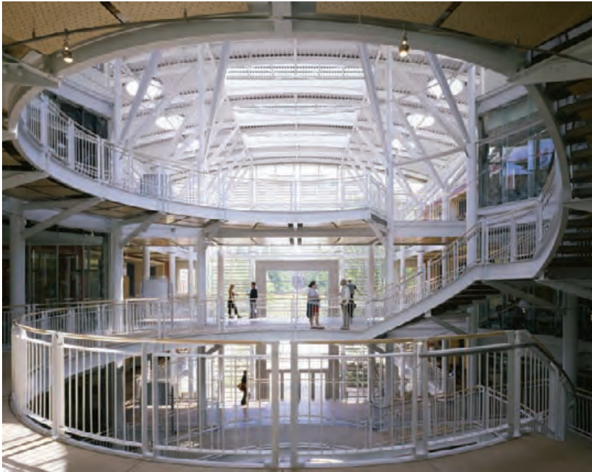
5.87 The Lillis atrium serves as an entry, circulation, and social space. Balconies along a circular stair provide study areas where students gather. The atrium also exhausts air from the classroom wings via stack ventilation. LARA SWIMMER PHOTOGRAPHY
