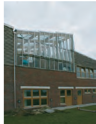
5.27 The ecological wastewater treatment facility occupies a greenhouse. TISHA EGASHIRA
