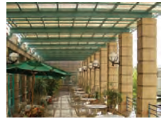
4.107 South-facing shaded outdoor balcony at Arizona State University School of Architecture, Tempe, Arizona.
