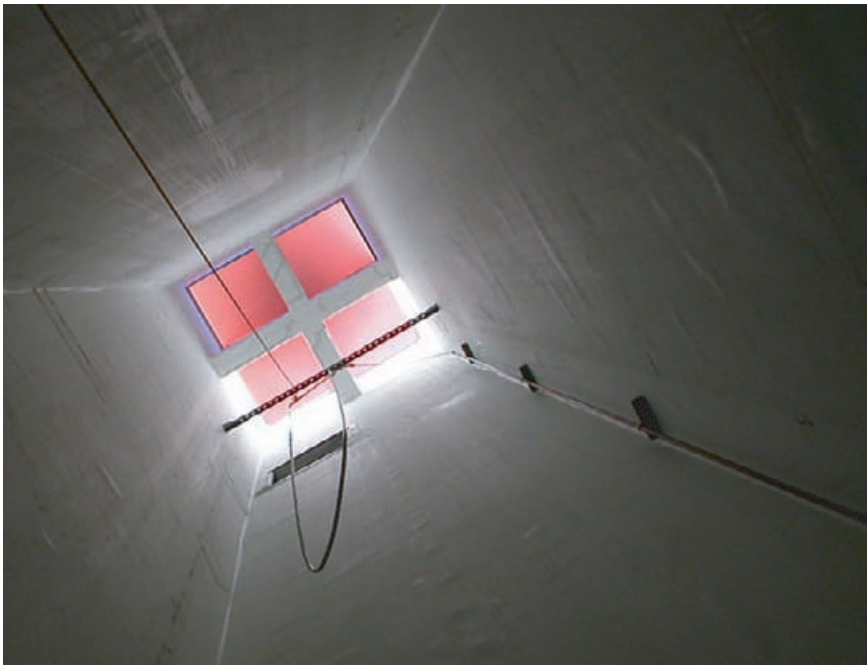
4.176 Looking up into the mister (the equivalent of a wetted pad) at the top of the cool tower of the Global Ecology Research Center. ROBERT MARCIAL
