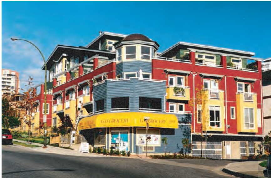
4.261 Quayside Village Cohousing Community in North Vancouver, British Columbia, Canada, a mixed use community with 19 residential units, uses a greywater recycling system to irrigate the community's compact, highly productive gardens. COHOUSING DEVELOPMENT CENTER
