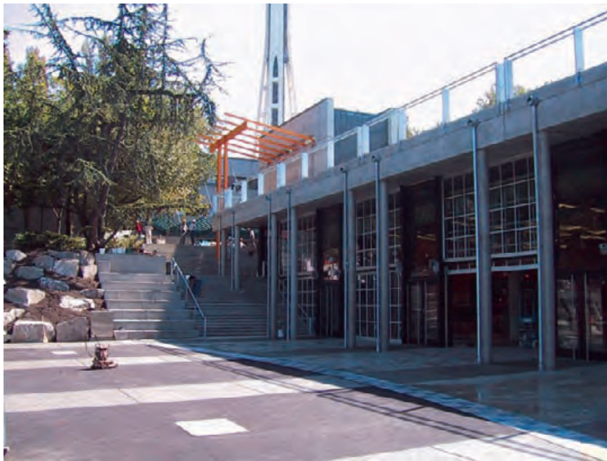
4.197 Tower plaza entry (in the foreground) to the Fisher Pavilion during construction shows the grade change to the top of the building via the stairway. MILLER/HULL PARTNERSHIP
