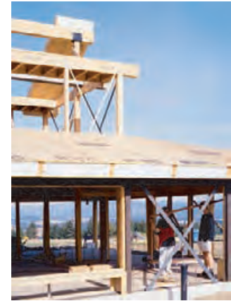
4.22 Residential construction using SIPs roof panels in Idaho.
