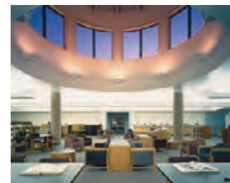
4.70 A clerestory “oculus” provides toplighting (integrated with electric lighting) at the Ryan Library at Point Loma Nazarene University in San Diego, California. ED GOHLICH
