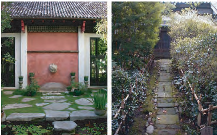
4.281 Garden pavers and grass (left) provide a permeable, green courtyard at the Chinese wing of the Honolulu Academy of Arts in Honolulu, Hawaii. A hierarchy of stone sizes and landscaping (right) provides a pervious entry path to a private house in Kanazawa, Japan.
