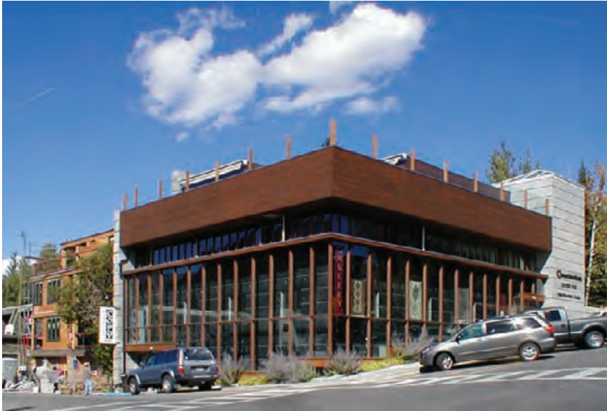
4.128 Thermal storage (Trombe) walls behind the glazed facades of this retail building in Ketchum, Idaho collect solar energy. BRUCE HAGLUND
