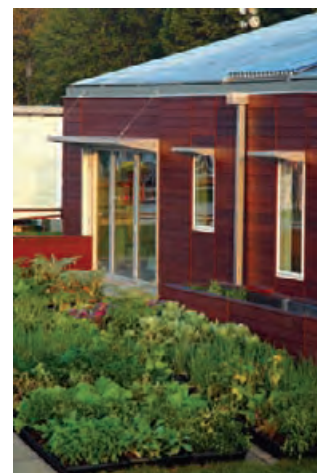
5.36 The Cornell University Solar Decathlon House utilized photovoltaics and evacuated tube solar collectors to provide for all of the energy needs during the competition. NICHOLAS RAJKOVICH
