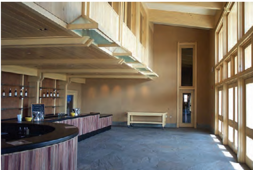
4.21 The Lytton Springs Winery has a daylit tasting room with smooth earthplastered strawbale walls and maple cabinetry and woodwork. MISHA BRUK, BRUKSTUDIOS.COM
