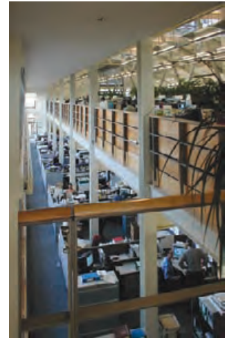
5.10 Daylight distribution to lower floors is facilitated by voids in the center and at one edge of the upper floor plate. TISHA EGASHIRA
