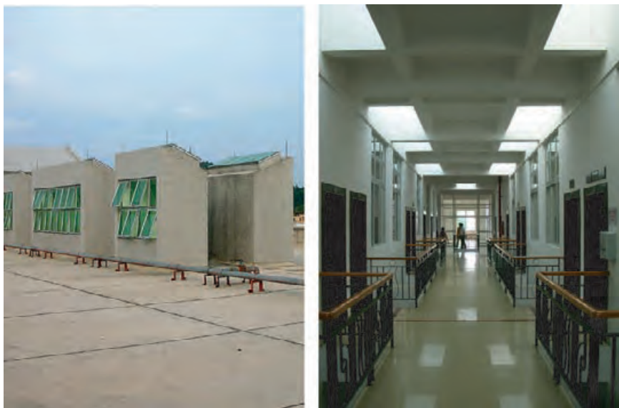
4.73 Skylight and clerestory monitors on the roof (left) of the administration building at Guangdong Pei Zheng Commercial College in Huadu, China; resulting toplighting distributed by light wells (right) provides illumination for four floors along a circulation corridor.
