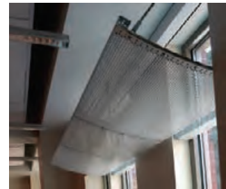
5.83 Light shelves made of metal screen bounce light up to the ceiling plane in the classrooms. SRG PARTNERSHIP
