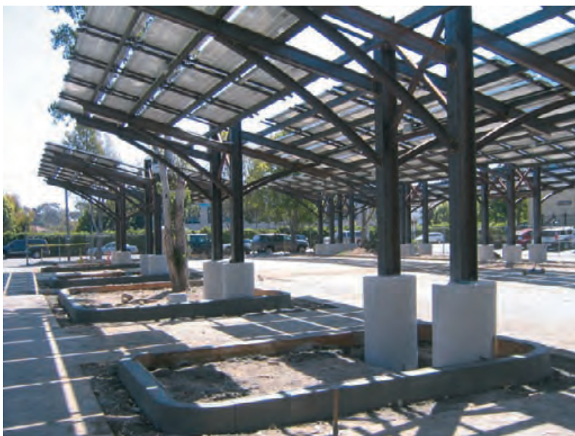
4.228 Photovoltaic panels shade parking areas as well as produce 67 kW of electricity at the Patagonia Headquarters, Ventura, California. MILLER/HULL PARTNERSHIP
