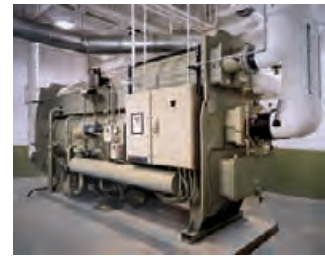
4.199 A single-stage, direct-fired absorption chiller. TRANE
