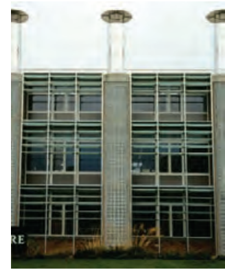
4.158 Solar chimneys at the Building Research Establishment offices, Garston, Hertfordshire, UK. THERESE PEFFER
