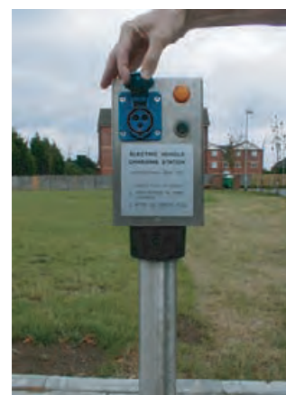
5.29 Free electric vehicle charging stations powered by photovoltaics. TISHA EGASHIRA
