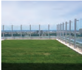
5.69 One of the green roofs used to mitigate stormwater runoff and the urban heat island effect.
