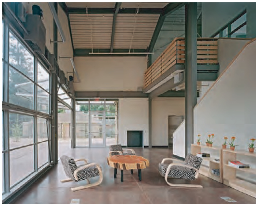
4.177 Exit opening—located in the lobby area—of the cool tower at the Global Ecology Research Center. © PETER AARON/ESTO
