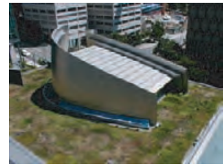
4.43 Green roof on Seattle City Hall in Seattle, Washington.
