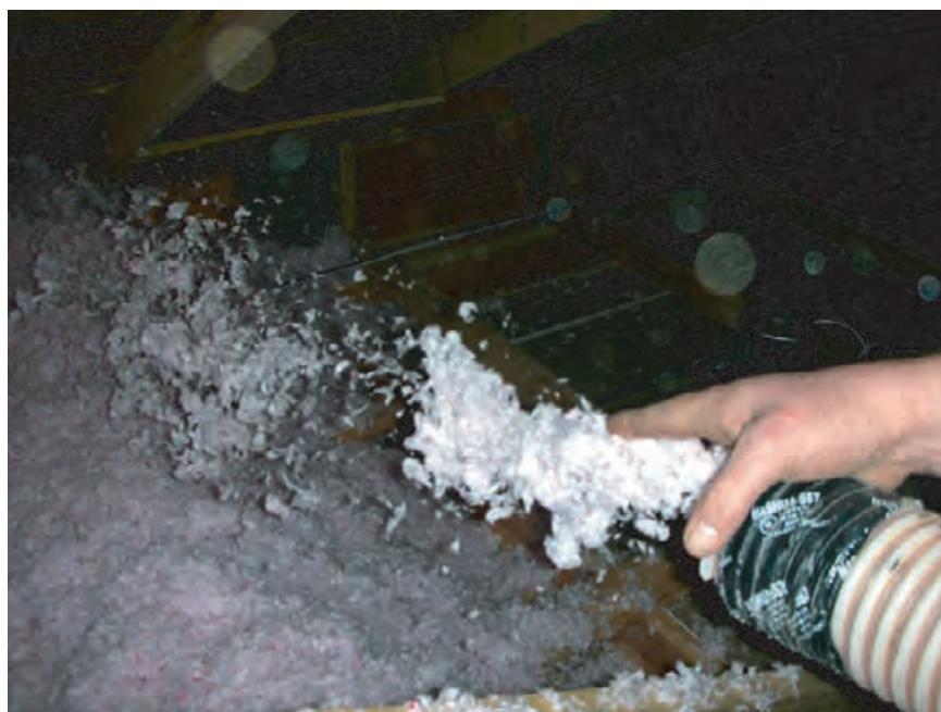
4.8 Loose-fill glass fiber insulation being blown into a new attic. This insulation is also used in existing homes because of its ease of application in difficult-to-reach areas.
