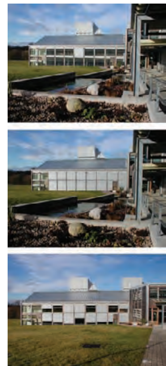
5.6 Three-image sequence shows exterior shades on the southeast facade of the lower pavilion controlled by the BMS, but with user override. TISHA EGASHIRA
