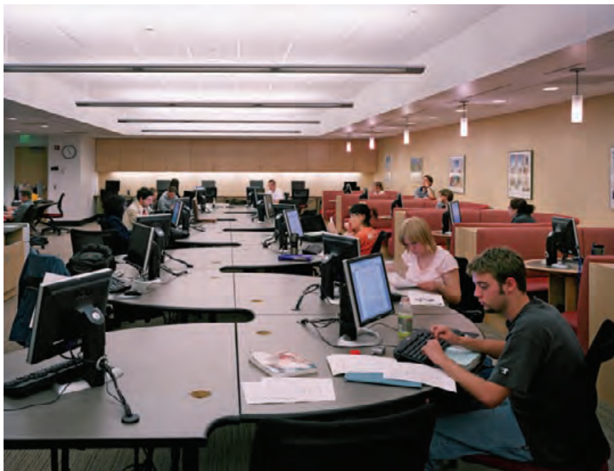
4.116 Indirect fluorescent luminaires (lighting fixtures) direct light to a reflective ceiling recess in a computing center at the Christopher Center at Valparaiso University, Indiana.
