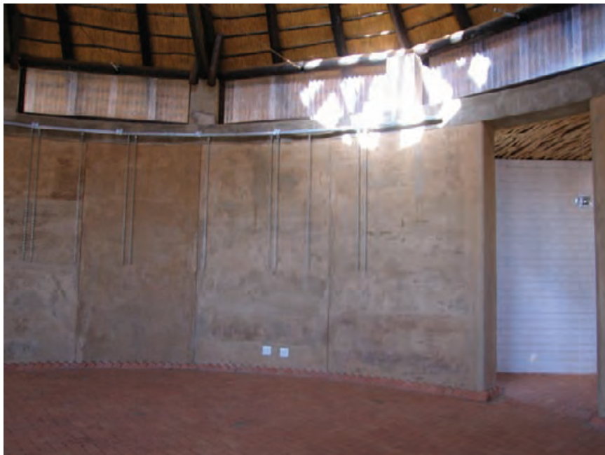
5.62 The exhibition hall, constructed of rammed earth (compacted by hand) and with reusable steel shutters. The load-bearing walls have a 4% cement mix and walls with 0–2% mixes alternate as infill panels. HEIDI SPALY
