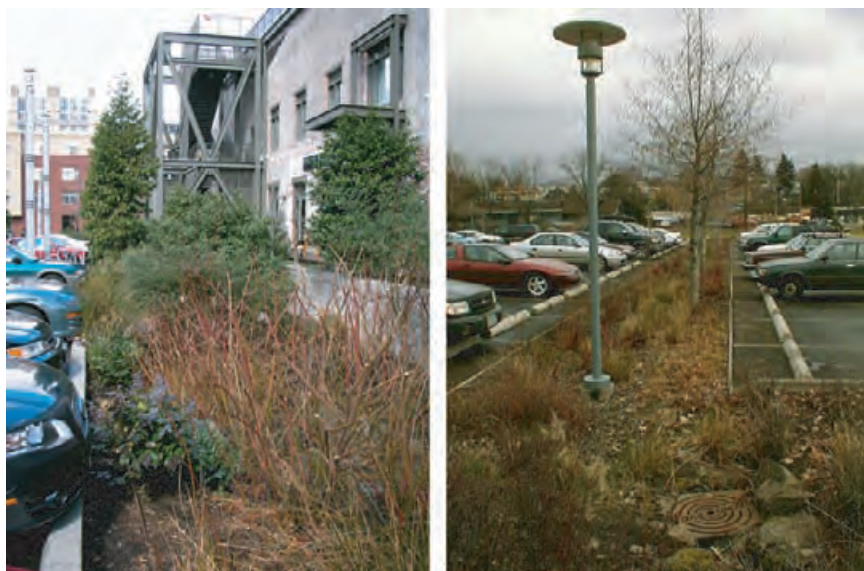
4.292 In Portland, Oregon, vegetated bioswales at the Jean Vollum Natural Capital Center (left) and the Water Pollution Control Laboratory (right) take rainwater runoff from the adjacent building and parking lot.
