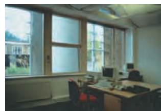
4.163 Windows open into the solar stack in an office space at the Building Research Establishment. The undulating ceiling provides a channel for cross ventilation across the building for night ventilation of thermal mass. THERESE PEPPER
