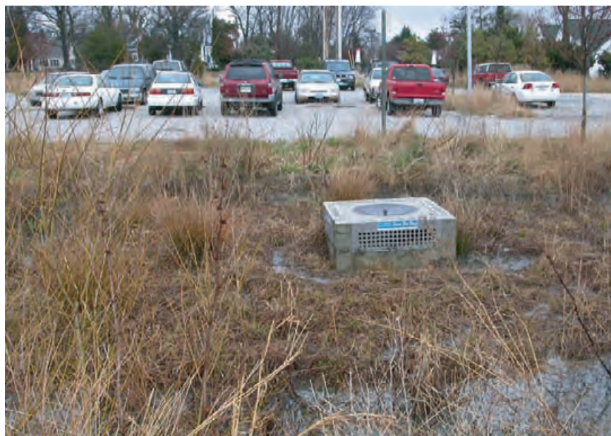
4.296 Wetland retention pond adjacent to a pervious surface parking lot at the Chesapeake Bay Foundation in Annapolis, Maryland. The raised overflow component allows for the infiltration of water during most storm events before returning any site runoff directly to the Bay.
