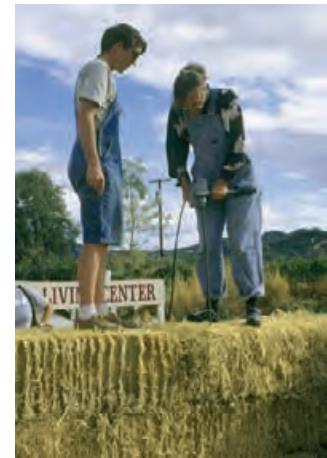
4.11 Drilling to place rebar into a strawbale.
