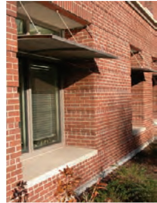
5.82 External shading on south-facing classrooms.
