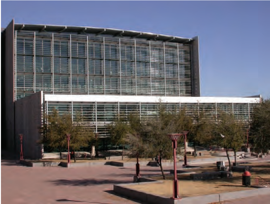
4.108 South-facing facade with horizontal shading louvers on the Burton Barr Central Library in Phoenix, Arizona.
