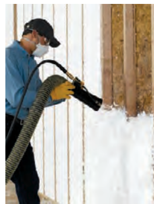
4.4 “Spider” is a lightweight glass fiber insulation bound with a non-toxic, water-soluble adhesive that also binds to cavity surfaces for gap-free coverage.
