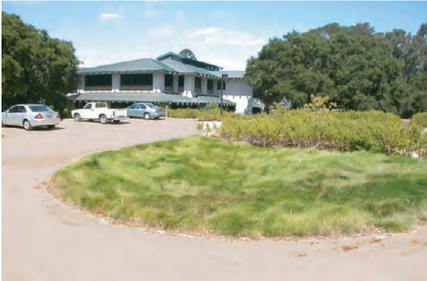
4.290 A swale planted with native California grasses and shrubs, next to a pervious surface parking lot at the Hewlett Foundation in Menlo Park, California.
