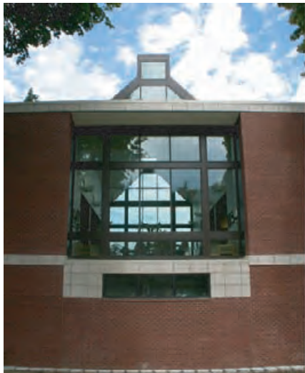
4.74 The Hood River Public Library (left) in Hood River, Oregon uses daylight and natural ventilation strategies; a long, clerestory monitor (right) illuminates the main reading area in the Library addition. FLETCHER FARR AYOTTE, INC.
