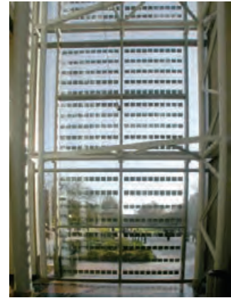
5.88 South-facing glass curtain wall has a 5.9 kW photovoltaic array. The PV cells are spaced farther apart at lower levels for better views and daylighting and closer together higher on the wall to produce more energy.
