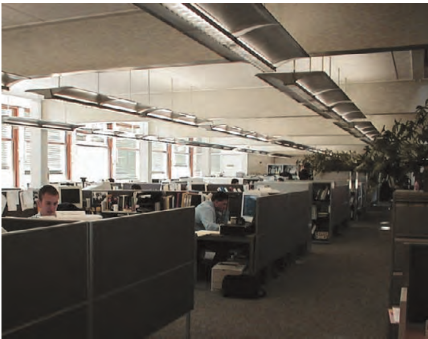
5.11 The lower floor receives daylight from the side and from above. Specially designed lighting fixtures provide direct and indirect illumination and sound absorption. TISHA EGASHIRA
