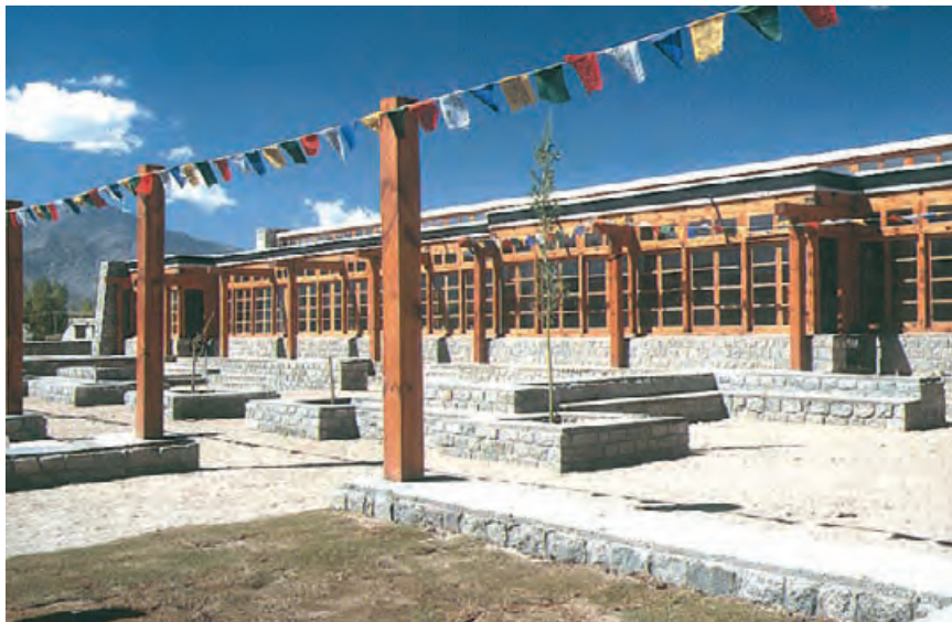
5.41 A series of outdoor classrooms comprise the Infant School courtyard of the Druk White Lotus School—one of several such courtyards. The planter boxes shown in this photo have been planted with willows. CAROLINE SOHIE, ARUP + ARUP ASSOCIATES
