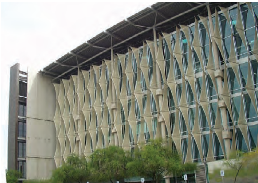
4.109 North-facing facade of the Burton Barr Central Library with “sail-fins” to shade against early morning and late evening sun during the summer months.
