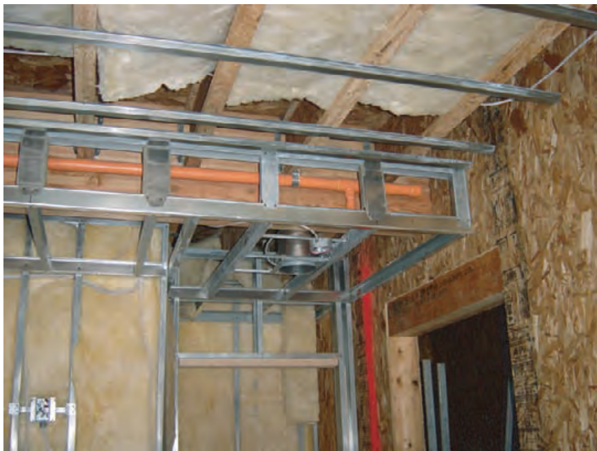
4.29 Combining SIPs (to the right) and conventional interior framing—to use the respective assets of each method to best advantage. AMELIA THRALL
