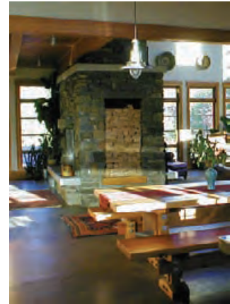
4.121 The concrete floor and stone fireplace absorb solar radiation from window and skylight apertures at the Bundy Brown residence in Ketchum, Idaho. BRUCE HAGLUND
