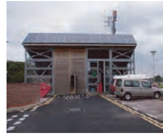
5.26 The CHP plant and its BIPV (building integrated photovoltaics) roof. TISHA EGASHIRA
