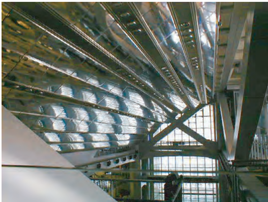
4.89 Specular reflectors (another way of thinking about light shelves) at the top of an atrium in the Hong Kong Shanghai Bank, Hong Kong, direct daylight to floors below.
