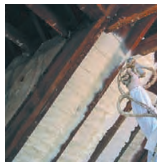
4.3 Application of open-cell polyurethane produced using water as a blowing agent.
