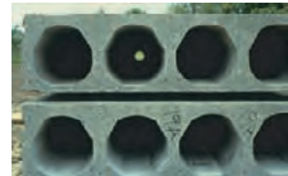
4.183 Cored concrete slabs used as thermal storage and air circulation channels in a night ventilation system. JOHN REYNOLDS
