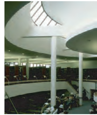
4.68 Skylight with large splayed distribution surfaces at Mt. Angel Abbey Library in St. Benedict, Oregon.
