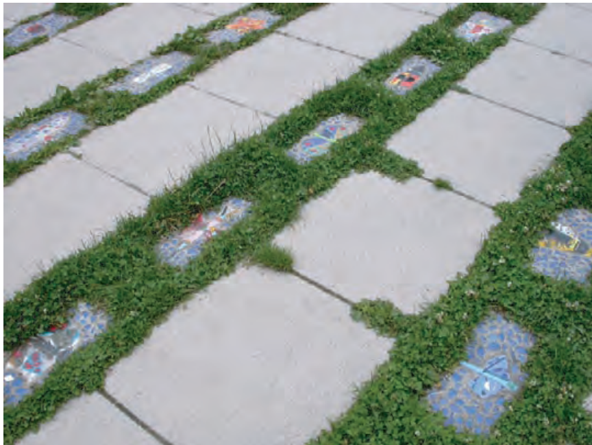
4.284 Pavers and tile artwork create a pervious patio near the dining hall of the IslandWood Campus on Bainbridge Island, Washington.
