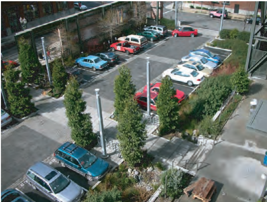
4.291 A porous paved parking lot is surrounded by vegetated bioswales at the Jean Vollum Natural Capital Center (Ecotrust Building) in Portland, Oregon.
