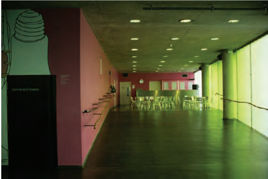
4.94 Translucent and tinted side apertures introduce daylight and modify its color as it falls on concrete floors and ceilings at the Laban Centre in London, UK. DONALD CORNER
