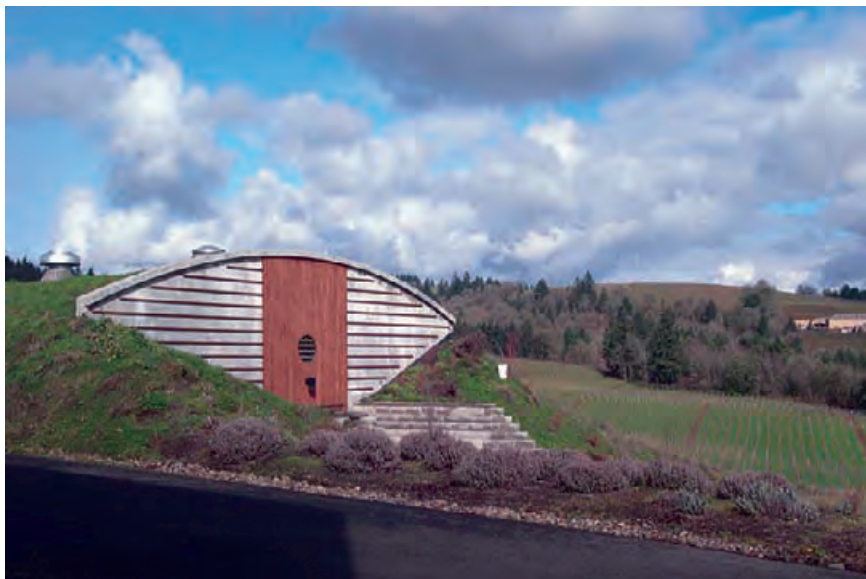
4.194 Vineyards farmed with sustainable practices surround an earth sheltered building serving as a wine processing and storage facility at the Sokol Blosser Winery in Dundee, Oregon. A green roof is integral with the earth sheltering.
