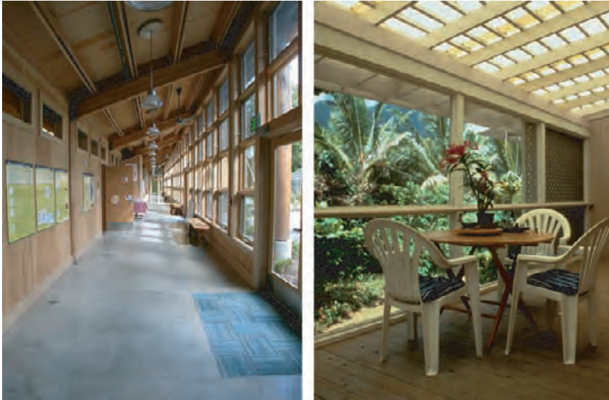
4.156 Operable windows along a corridor (left) allow air movement through a classroom building at IslandWood Campus, Bainbridge Island, Washington. Dog-trot house on Kauai, Hawaii (right) with cross ventilation through wrap-around porches used for indoor and outdoor living.
