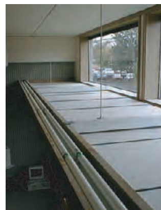
4.86 A matte, light-colored finish on the top of this light shelf diffuses daylight in multiple directions. Fluorescent lighting fixtures are integrated along the edge of the shelf.
