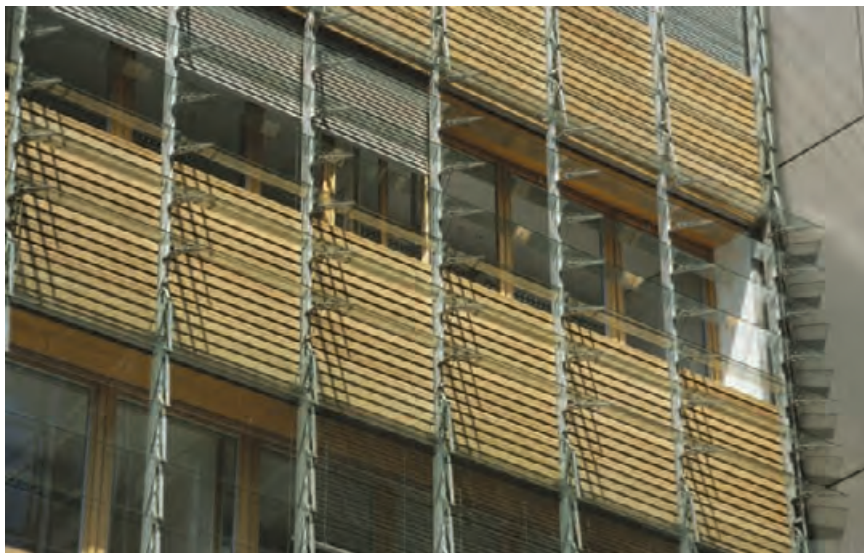
4.40 The double envelope facade of Bayerische Vereinsbank building in Stuttgart, Germany is a “re-wrap” or reconstruction of an existing building in which an operable leaf of glass louvers has been added in front of a system of operable strip windows. There are shades in the cavity.
