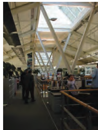
5.8 Roof pods provide daylight to both upper and lower floors.
