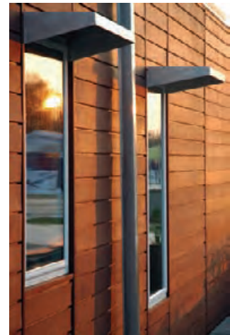
5.38 External shading on the south facade. NICHOLAS RAJKOVICH
