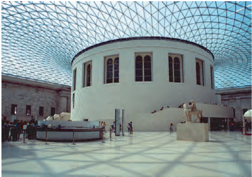
4.75 A glass canopy over the Great Court spans between the old and new portions of the British Museum in London, UK and provides delightful toplighting.
