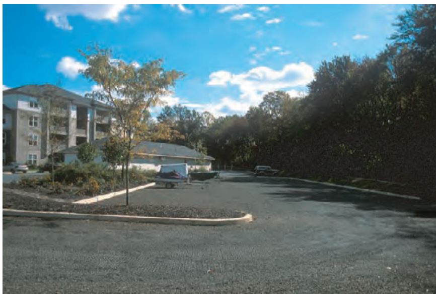
4.282 A porous paving system at an apartment complex in Virginia. INVISIBLE STRUCTURES, INC.
