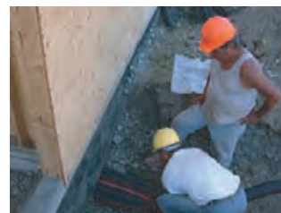
4.188 Inserting earth cooling tubes through a basement foundation wall. TANG LEE
