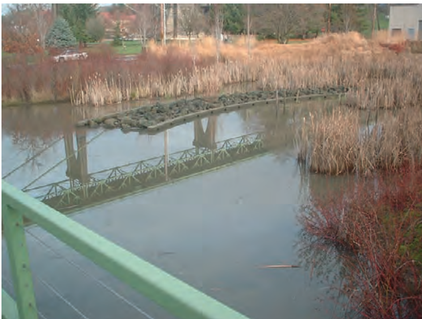
4.295 Native plants, shrubs, and grasses in the retention pond at the Water Pollution Control Laboratory in Portland, Oregon. TROY NOLAN PETERS
