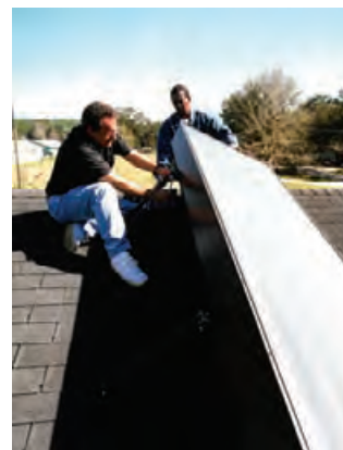
4.139 Typical batch solar thermal collector. FLORIDA SOLAR ENERGY CENTER
