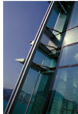
5.110 A ventilated cavity with modest aluminum shading devices and triple glazing with a low- \epsilon coating allows cool air exhausted from the building interior to pass upwards through the space between the glass panes. ROCCO DESIGN LTD.
