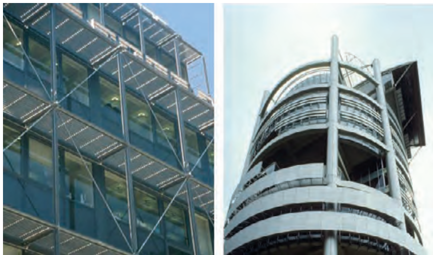
4.112 1 Finsbury Square (left) in London, UK uses classic, stout shading overhangs attached to a glass curtain wall and the Menara Mesiniaga (right) in Kuala Lumpur, Malaysia has horizontal shading bands to block the high equatorial sun. DONALD CORNER | ALISON KWOK
