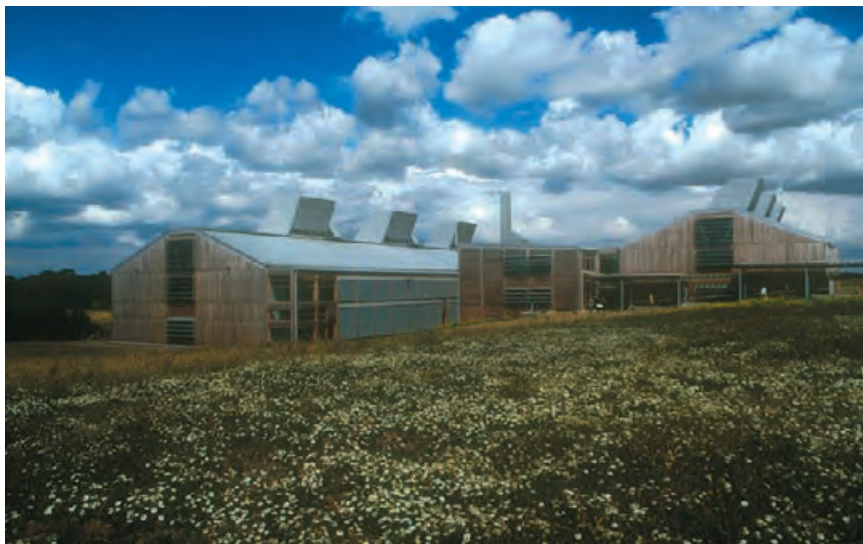
5.2 The Arup Campus, viewed from the south, fits the site contours. ARUP ASSOCIATES
