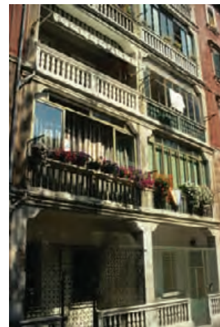
4.35 Glazed balconies in Venice, Italy.
