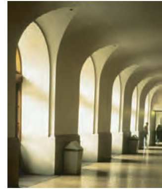
4.77 Sidelighting a corridor using glazed recessed doors; the Hearst Memorial Gymnasium, University of California Berkeley, Berkeley, California.
