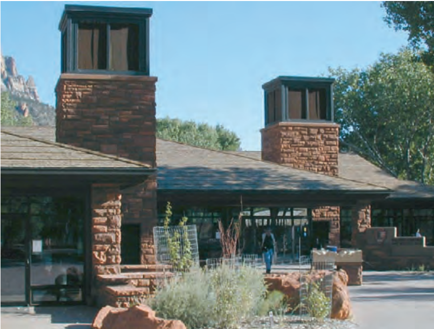
4.174 Evaporative cool towers at Zion National Park Visitor's Center, Zion, Utah. HARVEY BRYAN
