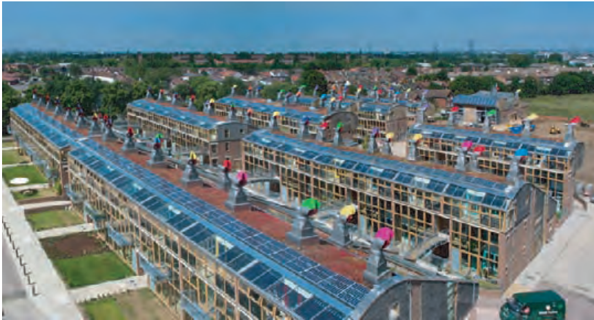
5.25 BedZED roofscape features windcowls, sedum, and photovoltaics. BILL DUNSTER ARCHITECTS/ ZEDFACTORY.COM
