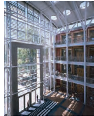
4.221 Atrium facade glazing (PV cells laminated within a glass curtain wall) at the Lillis Business School, University of Oregon, Eugene, Oregon. LARA SWIMMER PHOTOGRAPHY
