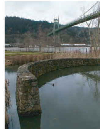
4.293 Stormwater retention pond at the Water Pollution Control Laboratory in Portland, Oregon. TROY NOLAN PETERS
