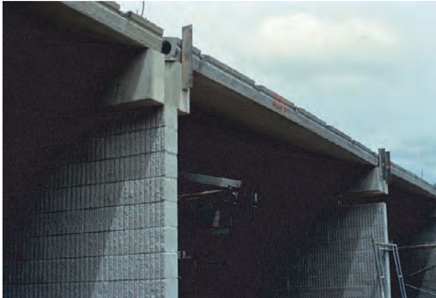
4.184 The Emerald People's Utility District office building in Eugene, Oregon uses mass in the floor, roof/ceiling, and partition walls coupled with cross and mechanical ventilation to cool the building during the overheated season. JOHN REYNOLDS
