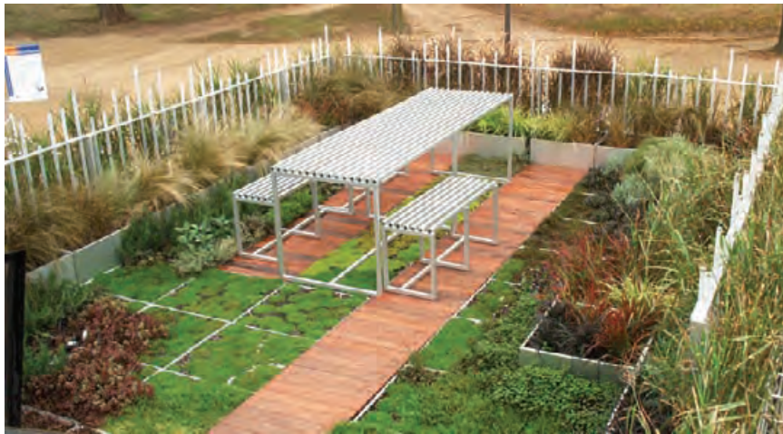
4.46 Extensive green roof and eating area on the 2005 Rhode Island School of Design Solar Decathlon House. JONATHAN KNOWLES
