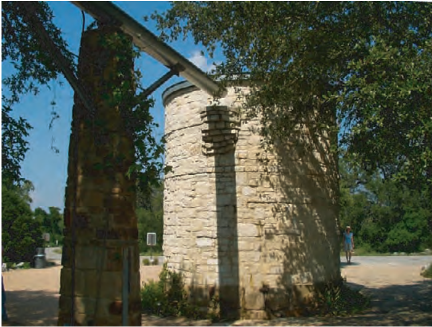
4.274 A large cistern at the entry to the Lady Bird Johnson Wildflower Center in Austin, Texas is constructed with native rock and is part of the extensive rainwater harvesting system at the Center.
