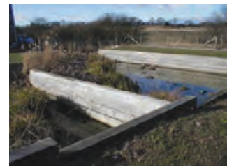
5.12 A retention pond below the buildings holds stormwater for ultimate evaporation or percolation. TISHA EGASHIRA
