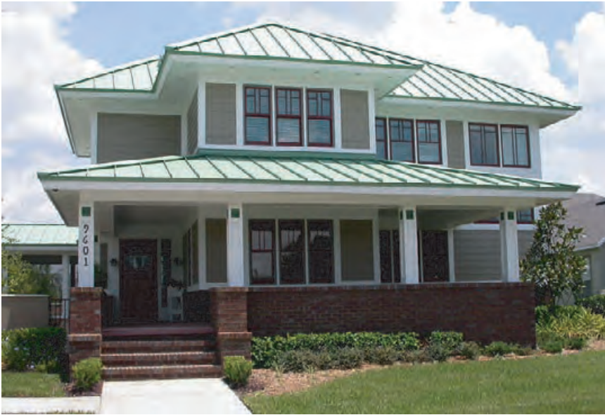
4.30 The Not-So-Big Showhouse in Orlando, Florida used SIPs. Visit www.ntsobigshowhouse.com/2005/virtualtour/ to view a video that includes footage shot in a SIPs factory and a crane setting the dormer of the home into place.
