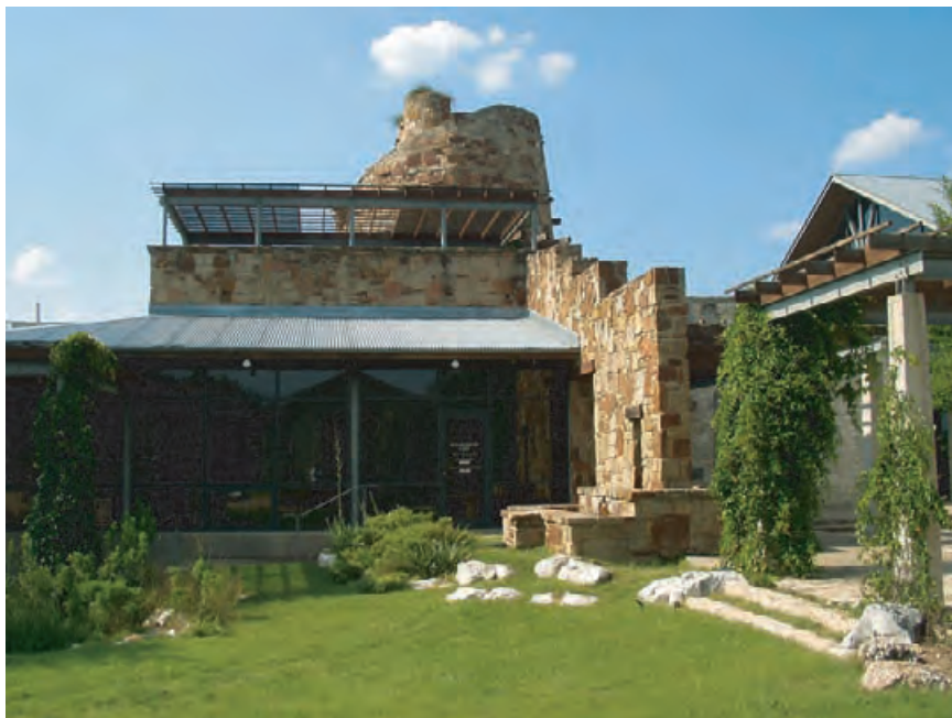
4.273 Observation tower and 5000 gal [18,930 L] cistern collect rainwater from the visitor's gallery and administration buildings at Lady Bird Johnson Wildflower Center in Austin, Texas.
