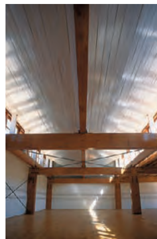
5.47 The splayed roof in the classroom acts as an indirect daylight source. Note the lack of operating electric luminaires.
