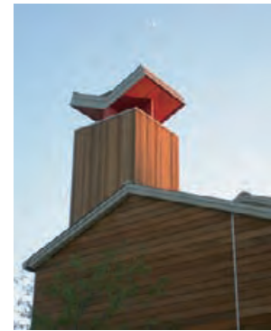
4.169 Evaporative cool tower at the Center for Global Ecology, Stanford University, Menlo Park, California.
