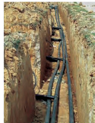
4.146 Installation of a large-scale horizontal ground loop in Arkansas. HYDRO-TEMP CORPORATION
