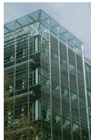
4.36 Outer glazing covers the entire surface of the facade at the Arup offices in London, UK.
