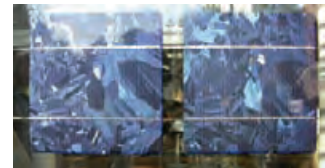
5.89 Glazing panel with embedded polycrystalline PV cells and interconnecting conductor strips.
