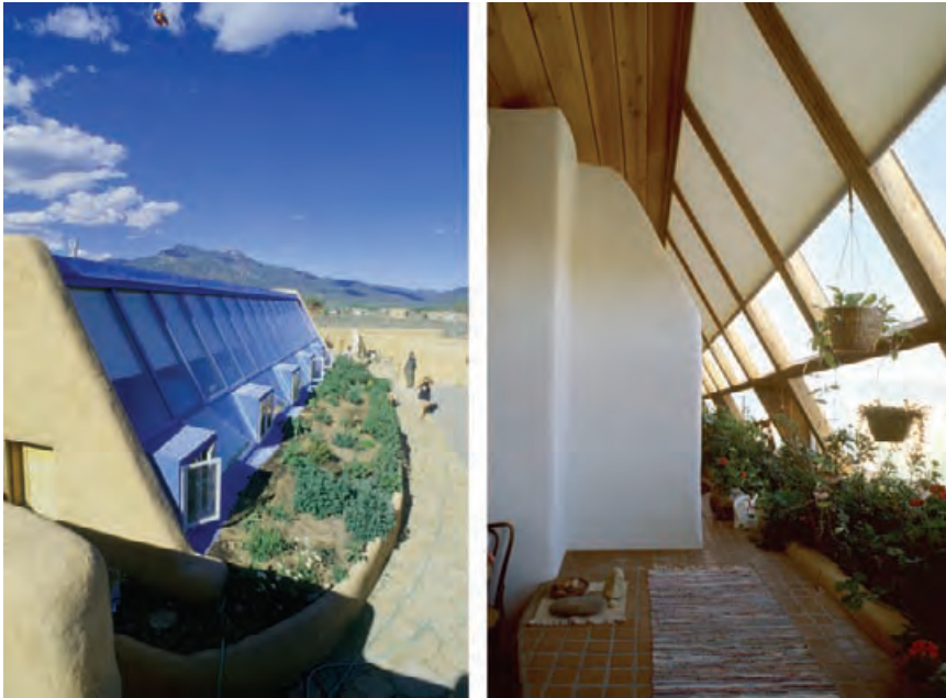
4.125 Classic example of solar apertures, solar control, and thermal mass in the Shaw residence in Taos, New Mexico.
