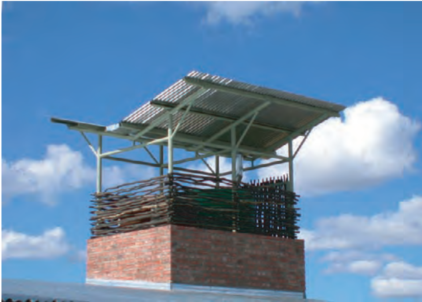
5.57 Evaporative cool tower with prosopis (mesquite) branches used to shade the storage tanks. NINA MARITZ
