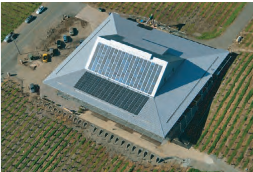
4.227 Photovoltaic panels incorporated into the roof form of the Ridge Winery, California. POWERLIGHT, INC.
