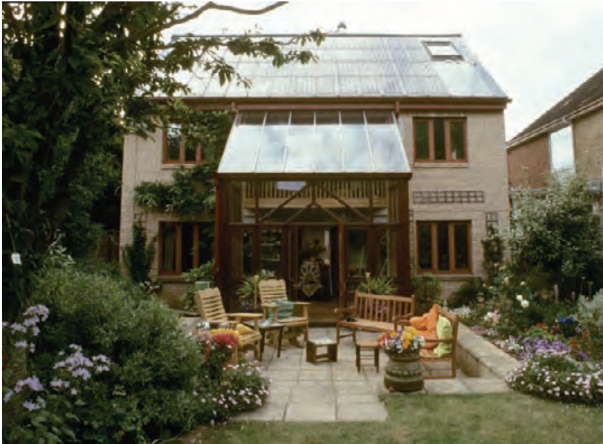
4.135 Ecohouse in Oxford, England integrates a number of strategies including an attached sunspace, roof integrated photovoltaic panels, and flat plate collectors for solar water heating.
