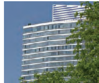
5.65 The Helena Apartment Tower. FXFOWLE ARCHITECTS, PC
