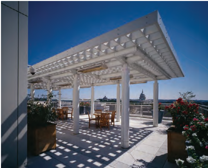
5.97 Shaded outdoor spaces provide break areas for occupants and a respite above the city. The trellis shades 30% of the roof area; container gardens and the white-colored roof reduce the urban heat island effect. ROBERT C. LAUTMAN
