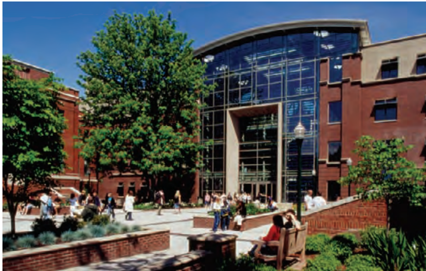
5.79 Entry plaza fronting the Lillis Business Complex; the entry facade is of laminated glass with integrated photovoltaics. LARA SWIMMER PHOTOGRAPHY
