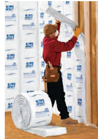
4.1 Installation of faced, formaldehyde-free batt insulation. JOHNS MANVILLE, INC.
