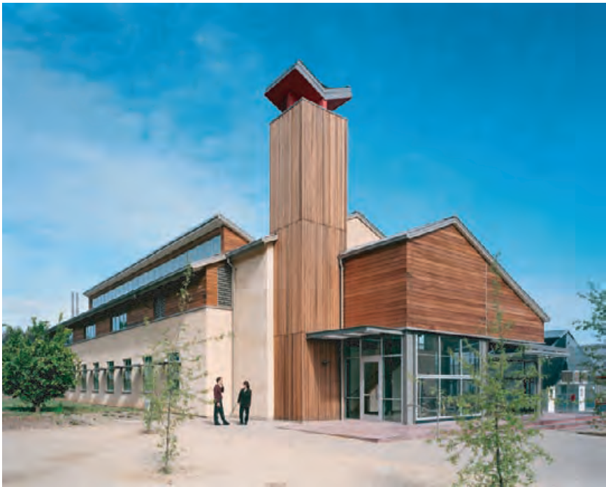
4.175 Evaporative cool tower at the Global Ecology Research Center at Stanford University, Menlo Park, California. © PETER AARON/ESTO
