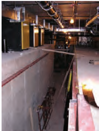
5.70 Blackwater treatment plant under construction. FXFOWLE ARCHITECTS, PC
