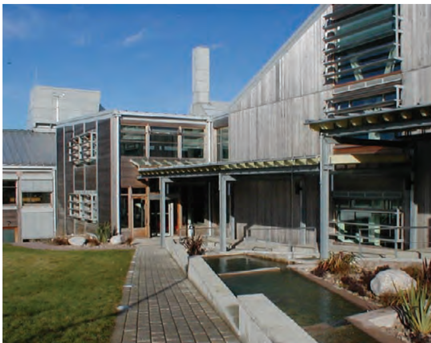
5.13 Water feature next to entry path to the reception cube along the southwest facade of the upper pavilion. TISHA EGASHIRA
