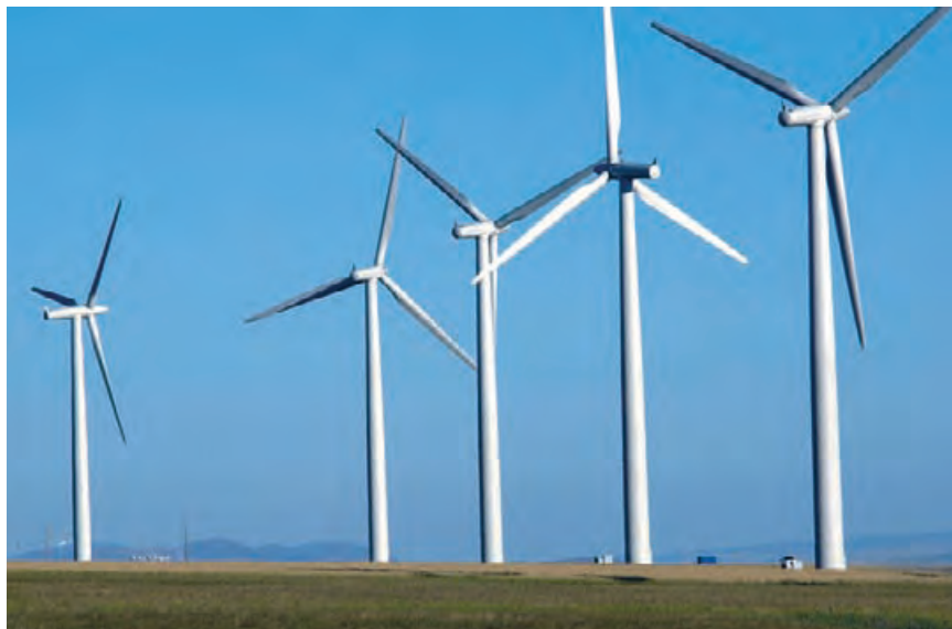
4.235 Nine Canyon Wind Project in Benton County, Washington was completed in 2002. Each of the 37 wind turbines has a rating of 1300 kW, yielding a project capacity of 48 MW.
