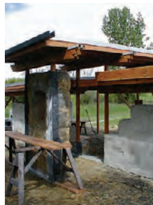
4.14 Strawbale bicycle shelter project under construction in Moscow, Idaho. BRUCE HAGLUND
