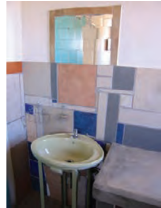
5.56 Bathroom tiling made of secondhand and broken tiles.
