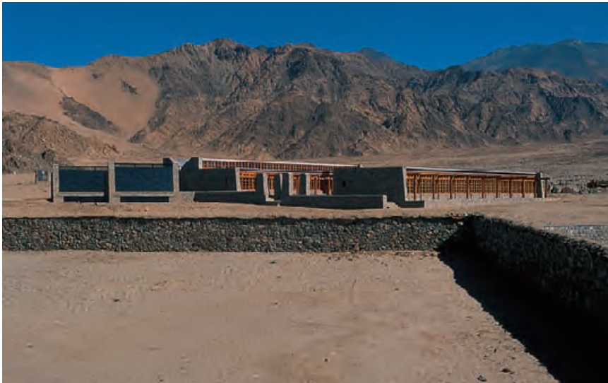
5.44 The Druk White Lotus School classrooms appear to emerge from the landscape. Their orientation takes advantage of early morning sunshine. CAROLINE SOHIE, ARUP + ARUP ASSOCIATES
