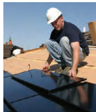
4.224 Monocrystalline silicon roof modules (peak power output of 63 W) are designed to replace composition shingles for residential buildings. POWERLIGHT, INC.
