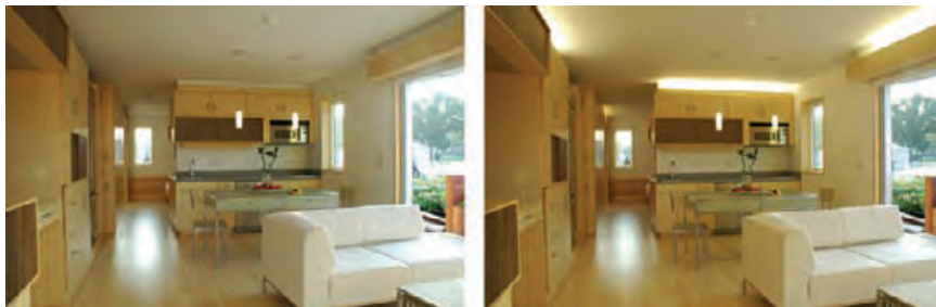
5.39 Electric lighting in the house is automatically dimmed by the building management system, depending upon outdoor light levels, to conserve electrical energy. NICHOLAS RAJKOVICH
