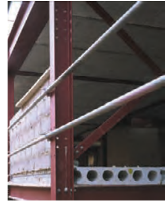
5.23 Construction features recycled steel framing and precast concrete floor planks. GRAHAMGAUNT.COM
