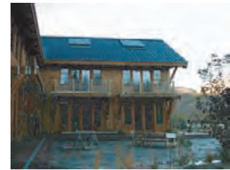
4.225 The Bundy Brown residence in Ketchum, Idaho uses 640 ft 2 [60 m 2 ] of BIPV (in the form of a photovoltaic laminate product adhered to the standing seam metal roof). The system has an output of 3.52 kW. BRUCE HAGLUND
