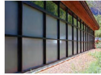
4.126 View of Trombe wall at Zion National Park Visitor's Center in Springdale, Utah. THOMAS WOOD, DOE/NREL
