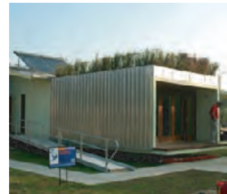
4.44 2005 Rhode Island School of Design Solar Decathlon House with a green roof for outdoor dining.
