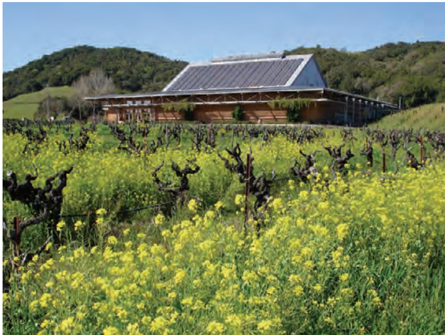
4.18 Ridge Vineyard's Lytton Springs Winery in Healdsburg, California used over 4000 rice-bales and integrates several green strategies including photovoltaics, shading devices (including vines), and daylighting. WILLIAM HOCKER
