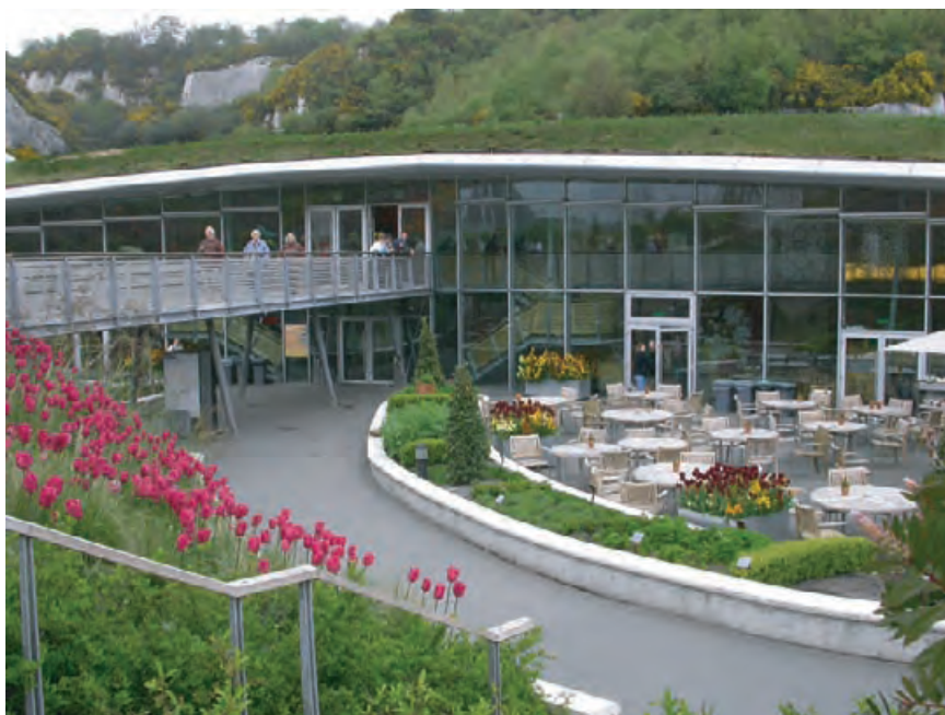
4.52 A green roof covers the restaurant at the Eden Project near St. Austell in Cornwall, UK.
