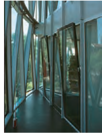
4.32 Buffer zone within the double envelope at the Westhaven Tower in Frankfurt, Germany. DONALD CORNER
