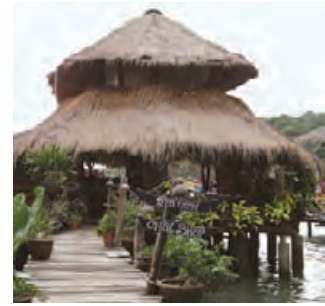
4.151 A café in Bang Bao, Koh Chang, Thailand utilizes high ceilings and windows for cross ventilation combined with thatched overhangs for shading.
