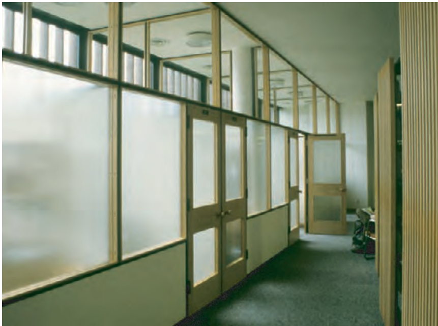
4.67 Three distinct daylight zones—reading cubicles, corridor, and stack area—in the Mt. Angel Abbey Library in St. Benedict, Oregon.
