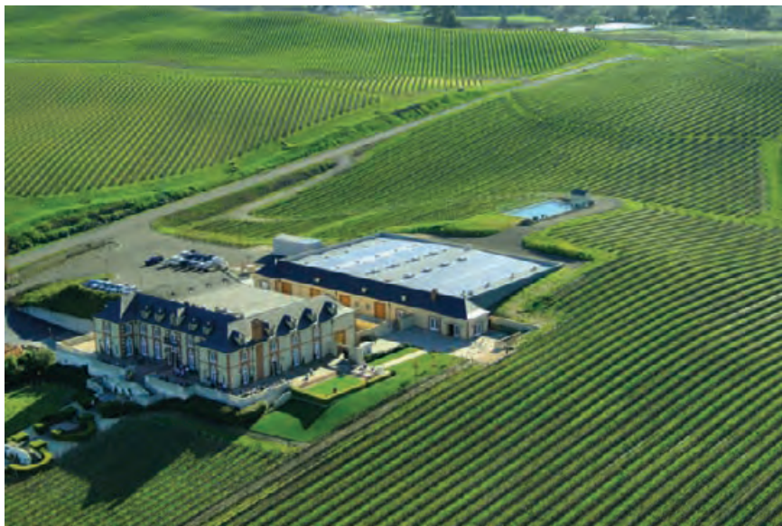
4.195 The earth sheltered Pinot Noir facility of Domaine Carneros Winery in Napa, California, begins to disappear into the soil of the vineyards. The roofscape also features 120 kW of building integrated photovoltaic panels to reduce the winery's annual energy consumption and carbon dioxide emissions. POWERLIGHT, INC.
