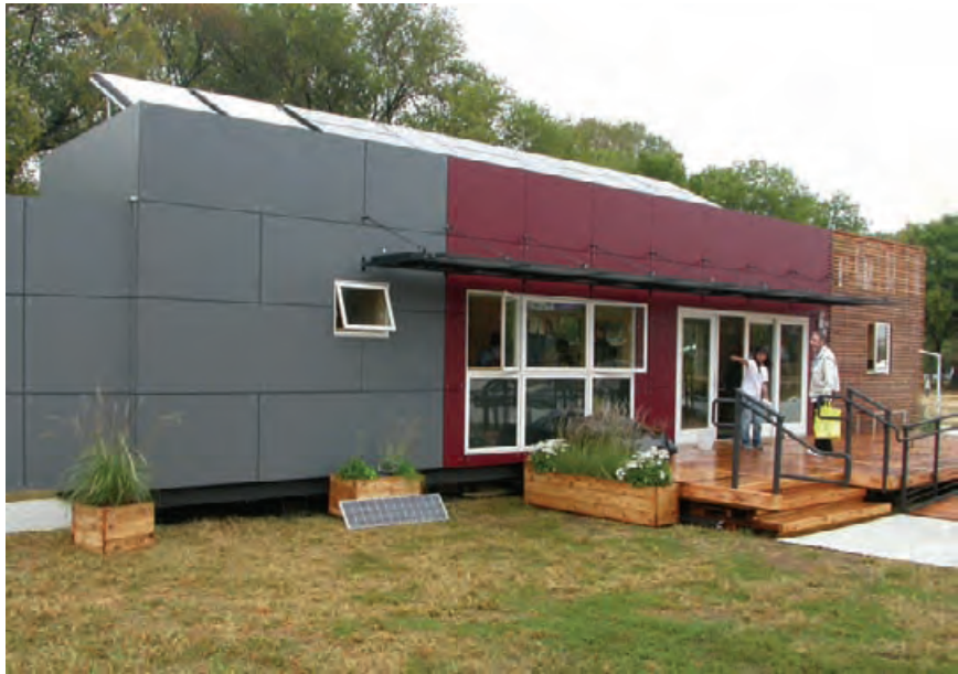
4.142 Flat plate solar thermal collectors (two panels on the left) integrate well with the photovoltaic modules (the array to the right) on the roof of the 2005 Cal Poly San Luis Obispo Solar Decathlon competition entry.
