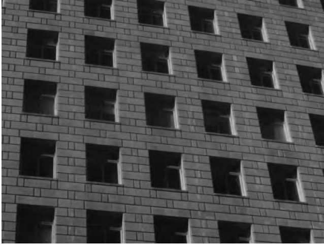
Fig. 9-2. Punched windows Source: FEMA (2009)
