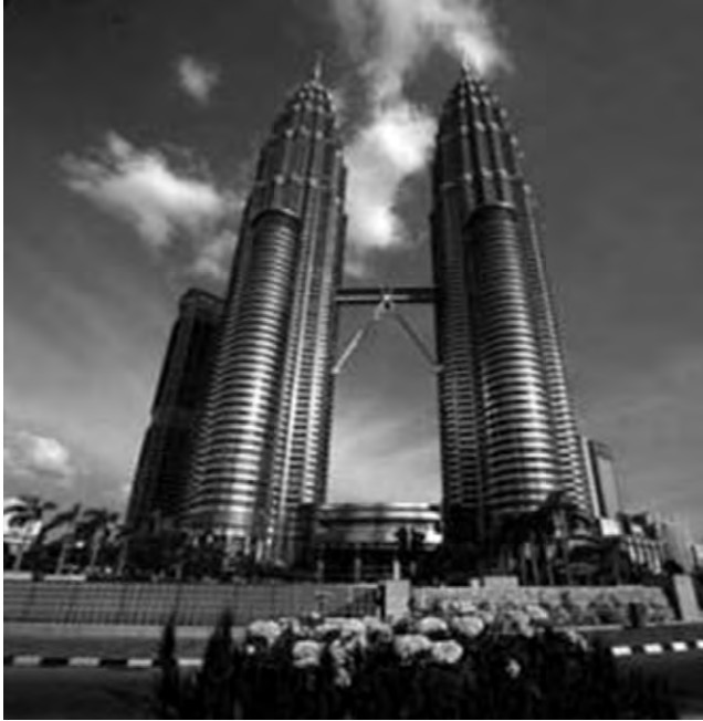
Fig. 3-3. Kuala Lumpur City Centre, Kuala Lumpur, Malaysia; an example of glazing and metal panels
