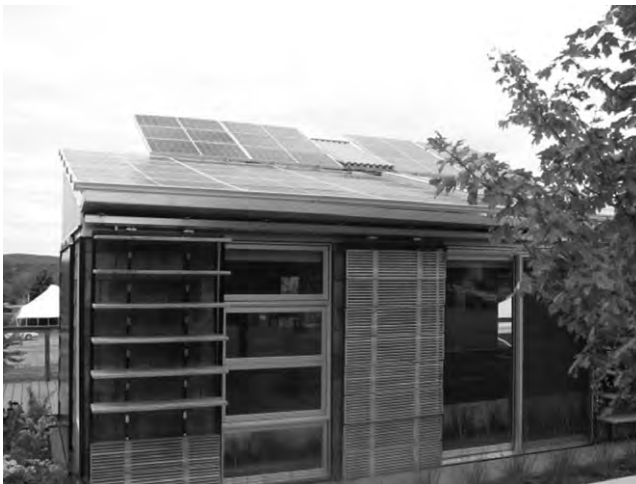
Fig. 11-3. Use of roof-mount solar arrays on Solar Decathlon House at Penn State University
