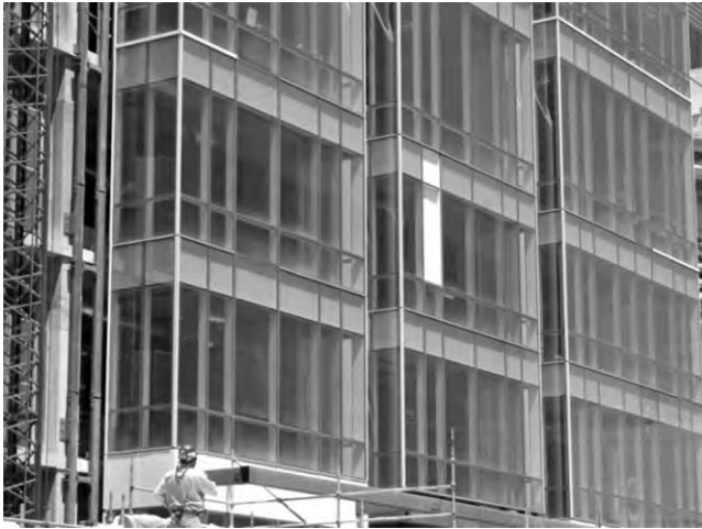
Fig. 8-14. Example of a four-sided SSG curtain wall
