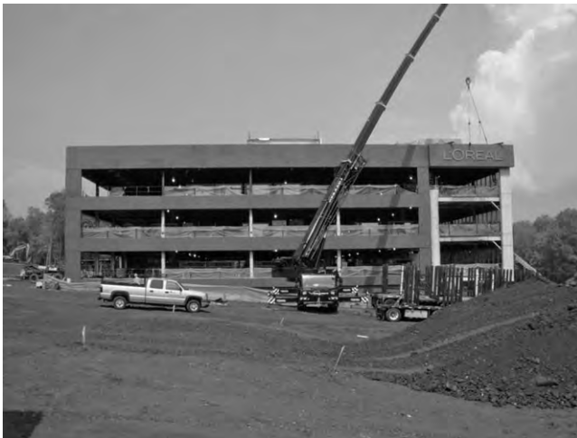
Fig. 3-8. Stone truss panel being installed
