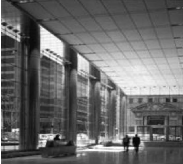
Fig. 3-18. UBS Tower, Chicago, IL; example of a cable net wall Source: Courtesy of Thornton Tomasetti; reproduced with permission
