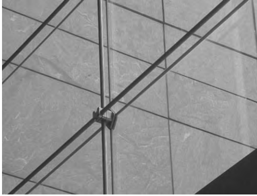
Fig. 9-4. Point-supported windows
