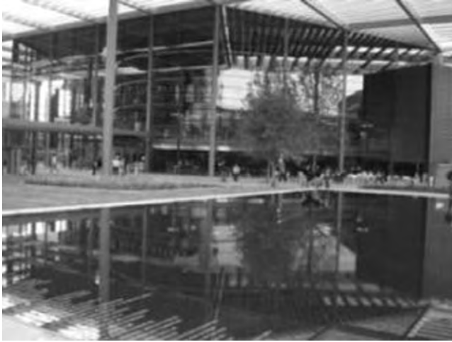
Fig. 3-1. Winspear Opera House, Dallas, TX; an example of all clear glazed façade
