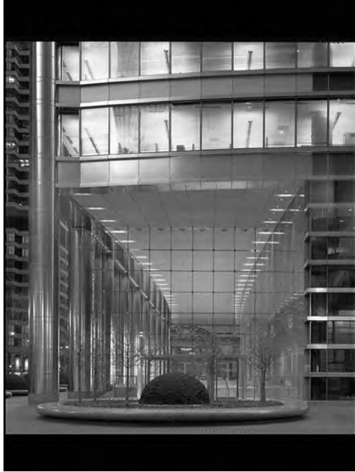
Fig. 3-25. UBS Tower, Chicago, IL
