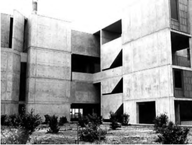
Fig. 9-6. Cast-in-place reinforced concrete envelope Source: FEMA (2009)
