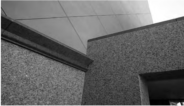
Fig. 3-7. Naples Philharmonic Museum, Naples, FL; an example of natural stone façade (granite)
