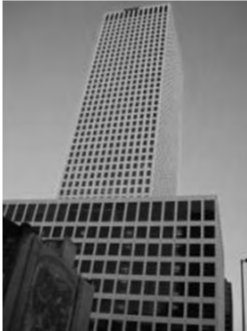
Fig. 3-2. One Shell Square, New Orleans, LA; an example of a high-rise building with a glazing and natural stone façade
