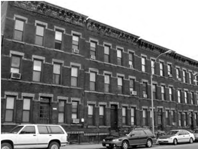
Fig. 9-7. Slender, nonreinforced masonry envelope Source: FEMA (2009)
