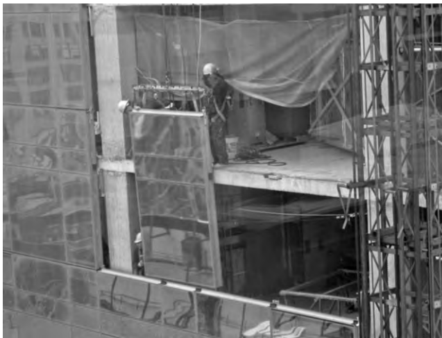
Fig. 8-11. Example of a unitized curtain wall system under installation in a multistory building
