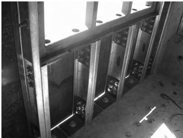
Fig. 9-21. Steel stud blast system
