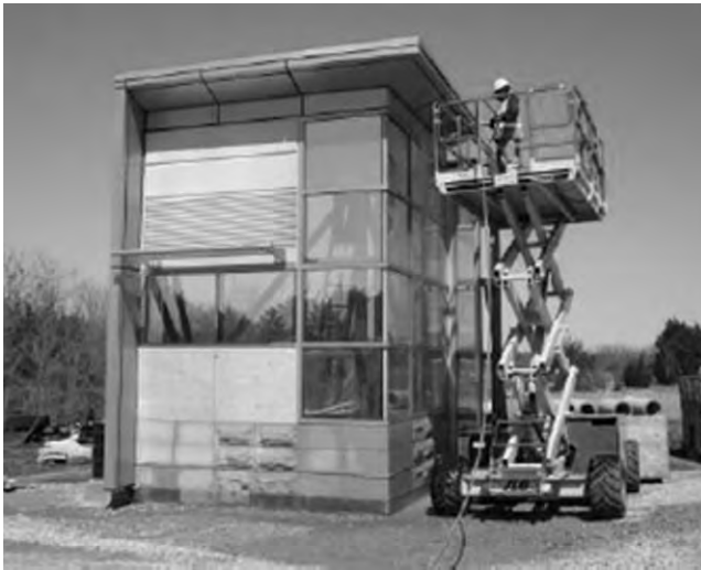
Fig. 4-1. Example of a field visual mockup showing multiple substrates and components
