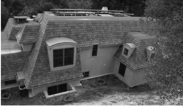
Fig. 11-4. Roof-mount solar arrays and support framing on a house in Los Altos Hills, CA (view from hilltop, solar panels facing downhill)
