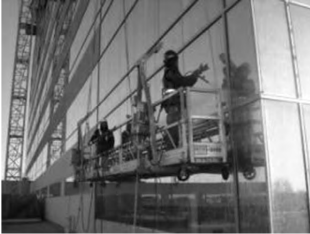
Fig. 4-15. A hose nozzle test AAMA 501.2
