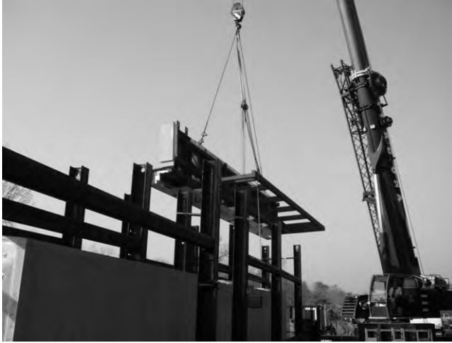
Fig. 3-9. Stone truss panel being hoisted from transportation vehicle; note the steel frame back-up behind the stone panels
