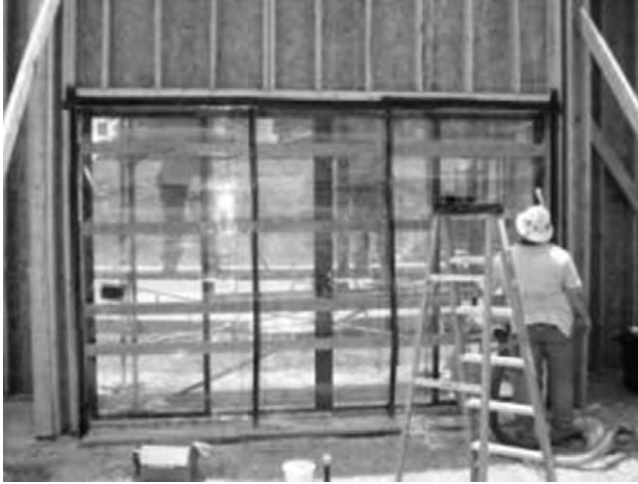
Fig. 4-13. A representative box chamber around a specimen that tests air leakage and water infiltration
