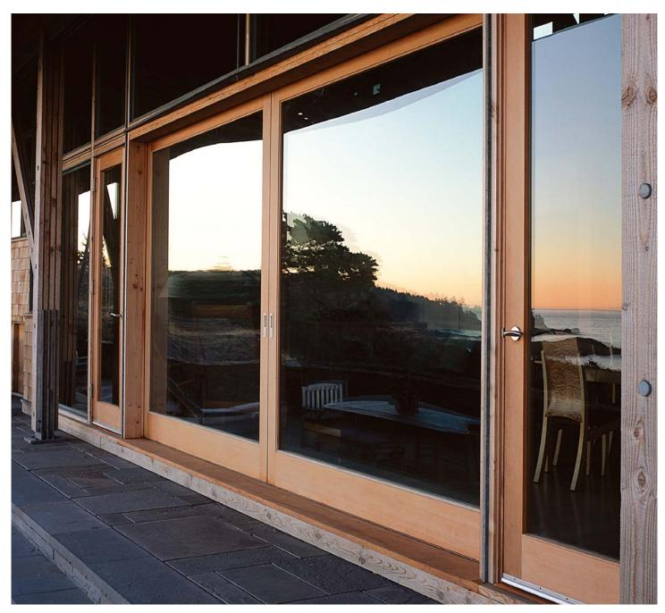
The steel band strength that allows this wall of glass to withstand high winds, at the same time makes the wall seem more delicate.
