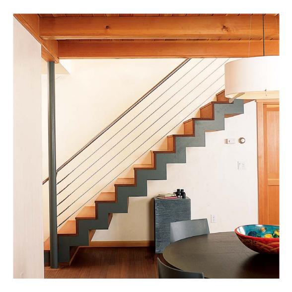
LEFT | Laser-cut steel allows this free-form stair to float in space, while the stainlesssteel cable in the railing is so delicate that it almost disappears.
