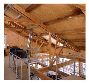
ABOVE 1 The second-floor loft is hung from the bottom chords of the roof trusses. Galvanized-steel railings and the exposed stainless-steel chimney add to the industrial aesthetic of this beach house.
