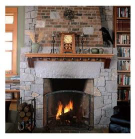
Combining small pieces of granite, brick for the chimney, and a wood mantel creates a fireplace that's just the right scale for the room. The square opening reveals that this is a Rumford fireplace, one of the most efficient heaters.
