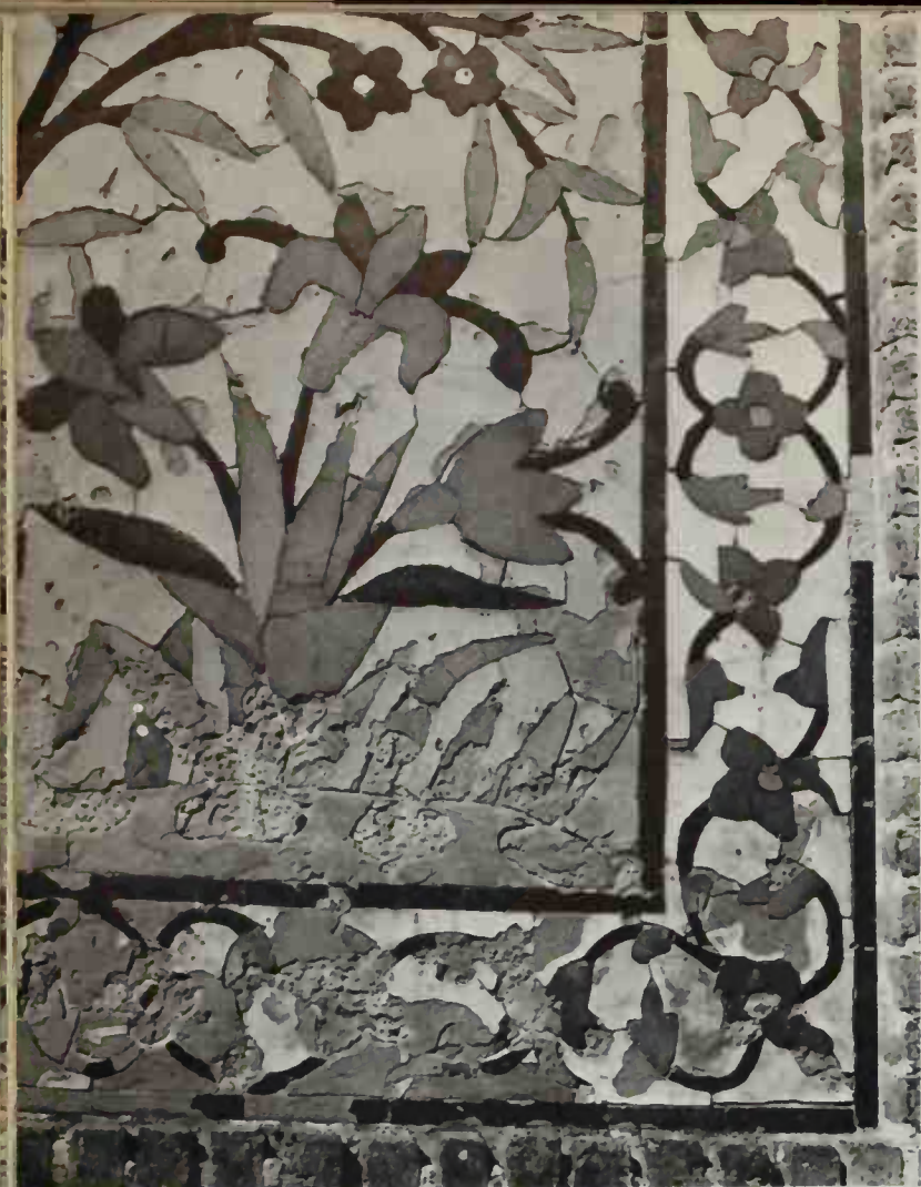
The separate nature of each petal, stem and leaf is evident in this mosaic tile-work from the courtyard. The damaged parts reveal the thinness of the coat of glaze
