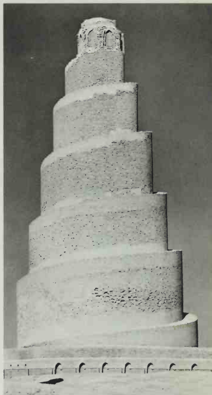
The brick minaret of the Great Mosque, the largest mosque in the world, built about AD 850. The ramp rises more steeply as it ascends in order to preserve an equal height for each diminishing circuit
