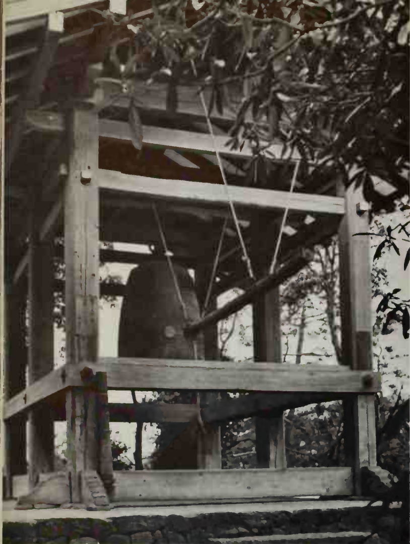
The Bell Tower, showing the balk of timber suspended on ropes which is swung against the side of the bell to sound it
