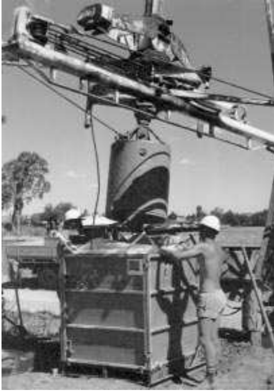
6.16 Calweld bucket drill dumping into sample container.
