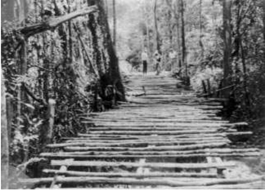
6.1 Local timber access for drilling across swamp; Ampulit, Kalimantan, Indonesia.
