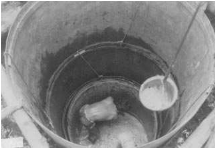
6.6 Reduction in caisson diameter with depth.
