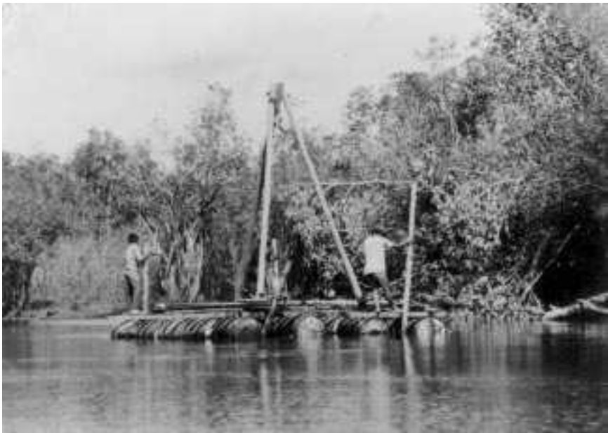
6.2 Floating drill platform for Banka drill; Ampulit, Kalimantan, Indonesia.
