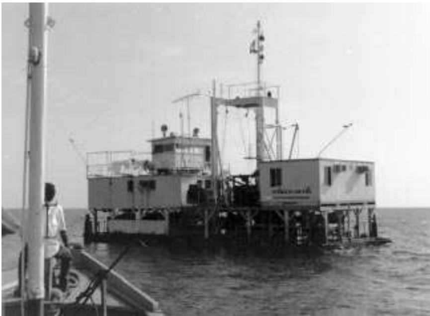
6.25 The drilling vessel Supphayakornthoranee – Andaman Sea Offshore Project, Thailand.
