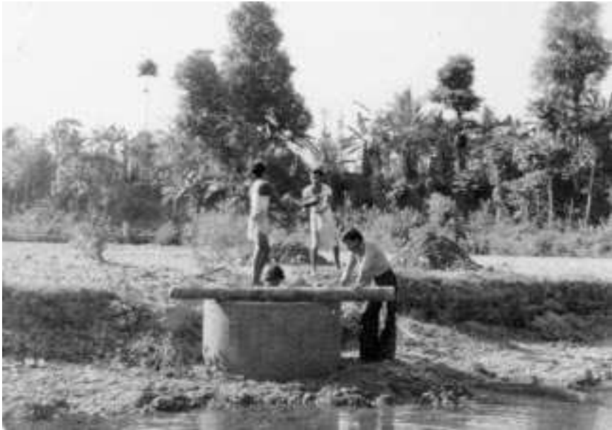
6.4 Driving a flush-jointed caisson, Punna Puzza, Kerala, India.
