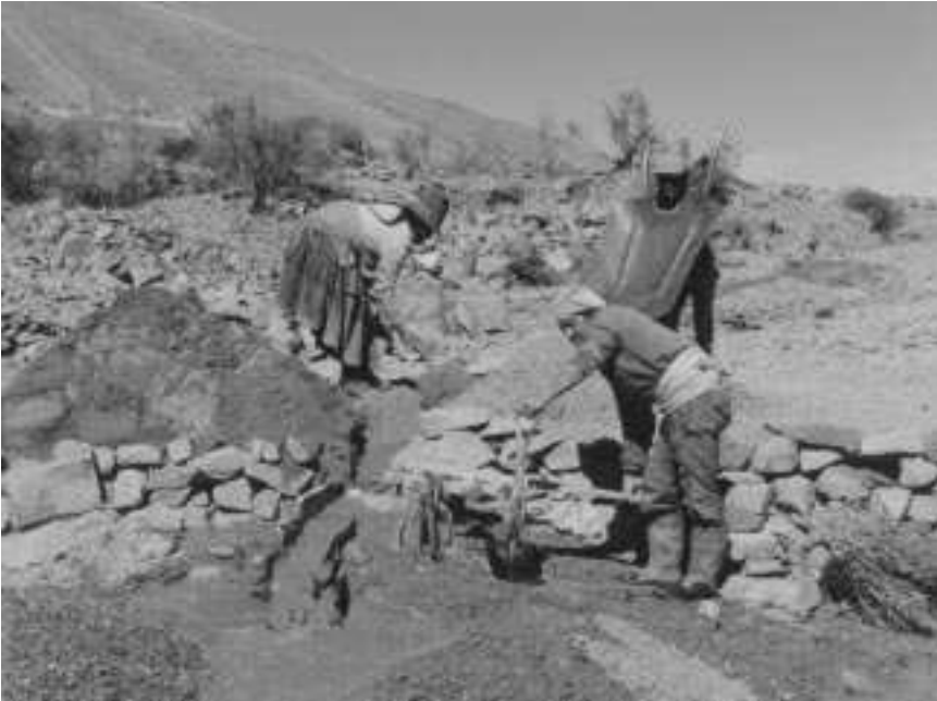
7.9 Ground sluicing alluvial deposits in Bolivia.
