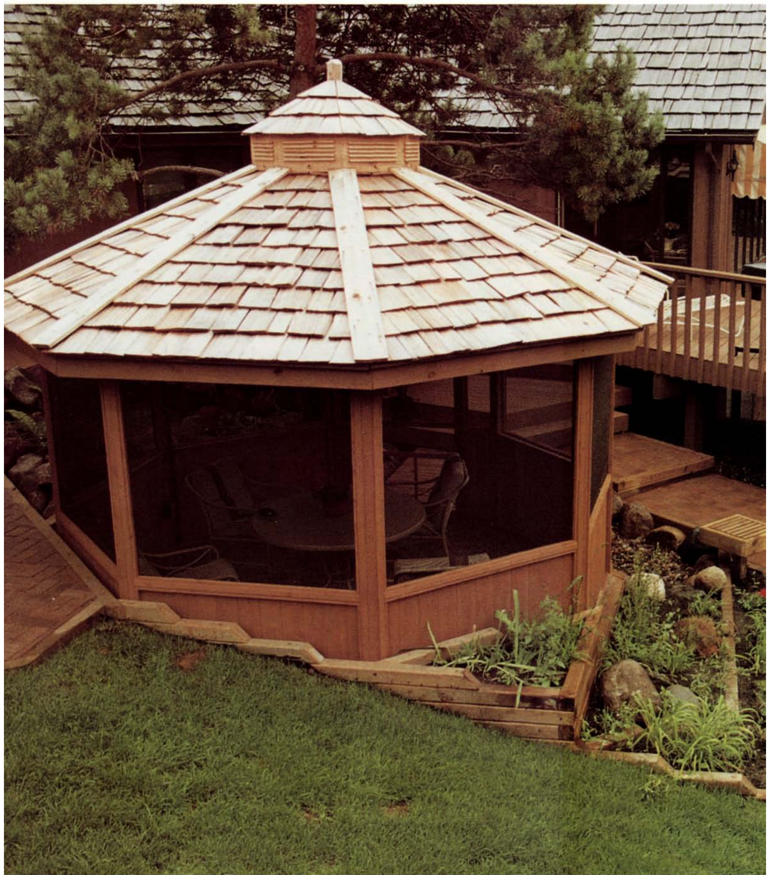
Gazebos should blend in with the architectural and environmental landscape. The gazebo featured above avoids visual isolation by meshing perfectly with its surroundings.
