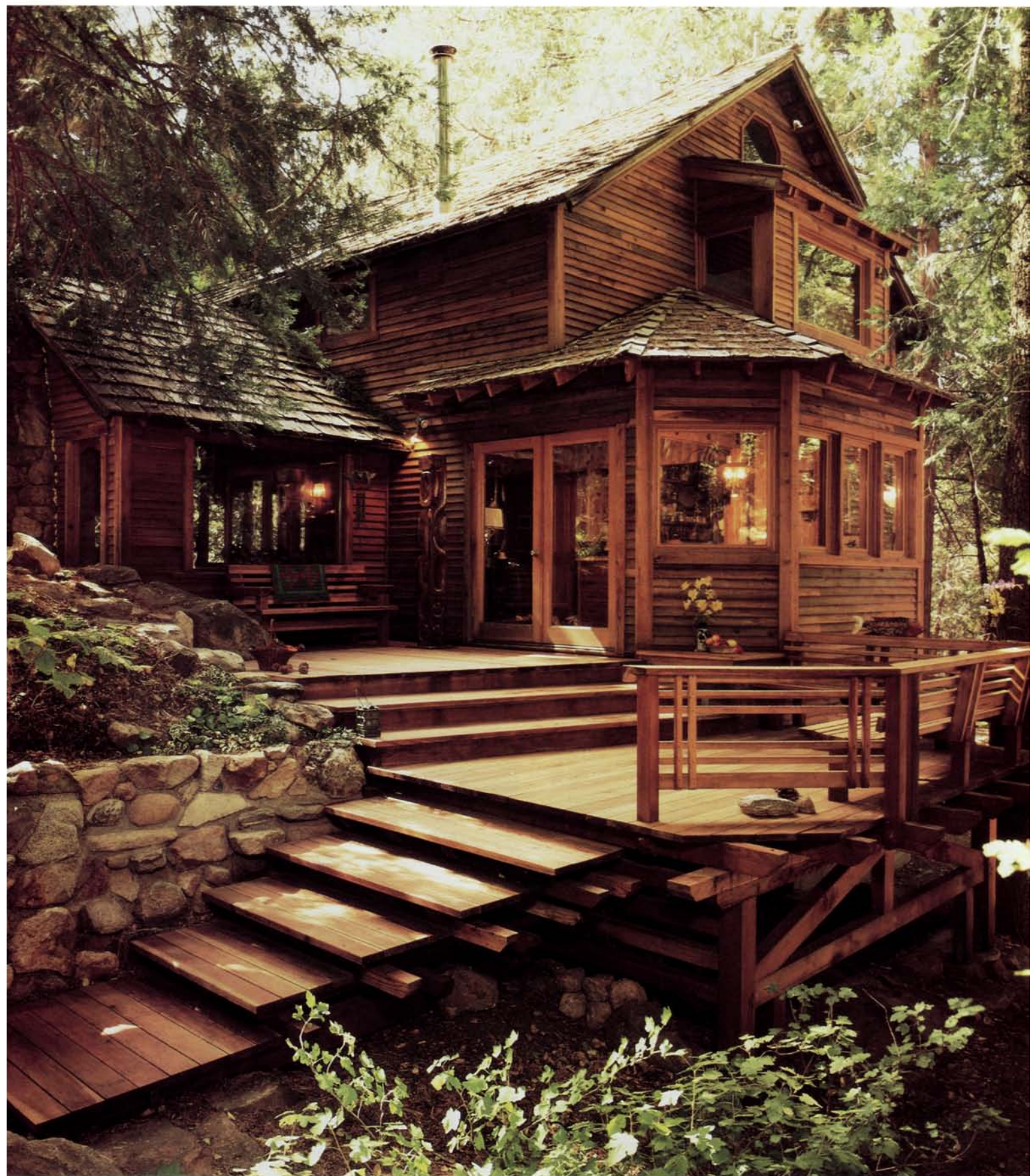
Combining two deck design ideas creates an effective outdoor activity area. The space created by the shape of the house is filled by the top level of the deck. A second level, elevated above uneven terrain, wraps around an extended bay window to create a separate sitting area.
