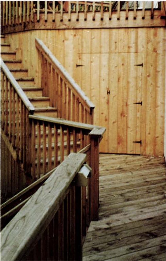
Many deck designs take full advantage of the space beneath the upper levels of a deck by turning these areas into enclosed storage sheds.
