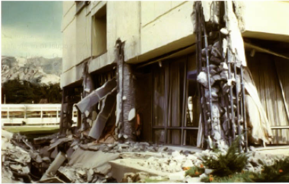
Olive View Memorial Hospital following the San Fernando earthquake of 1971. The columns supporting the discontinued shear walls are required by ASCE 7-10 to be designed for seismic load effects including overstrength factor.
