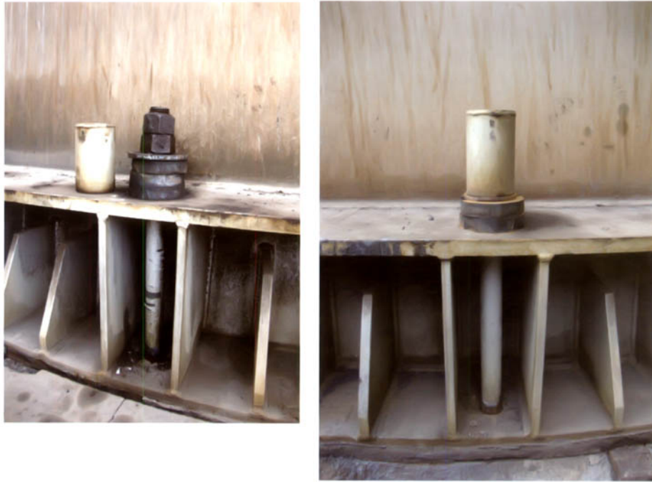
Anchors in concrete used for nonbuilding structure anchorage in Chile Courtesy of J. Silva, ASCE/SEI 2010 Chile Earthquake Reconnaissance Team
