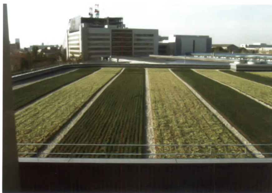
Weight of landscaping and other materials at roof garden is to be included in effective seismic weight.
