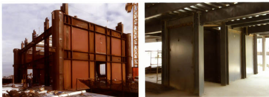
Special Steel Plate Shear Walls
