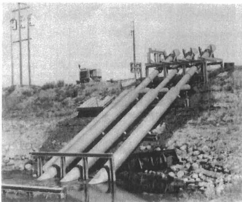
**Figure 9-10.** Incline-mounted line shaft pump.
