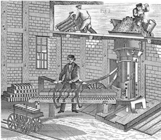
Fig. 16 First upright auger extruder powered by steam, 1858
