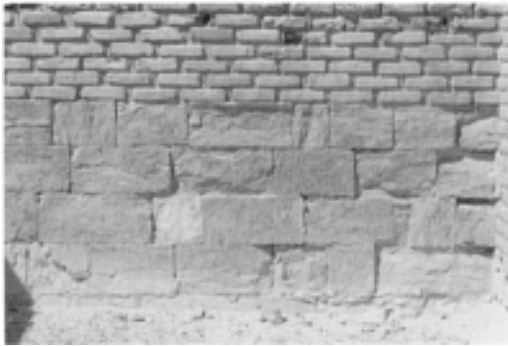
Stone and brick construction, Qasr al-Tuba, Jordan
