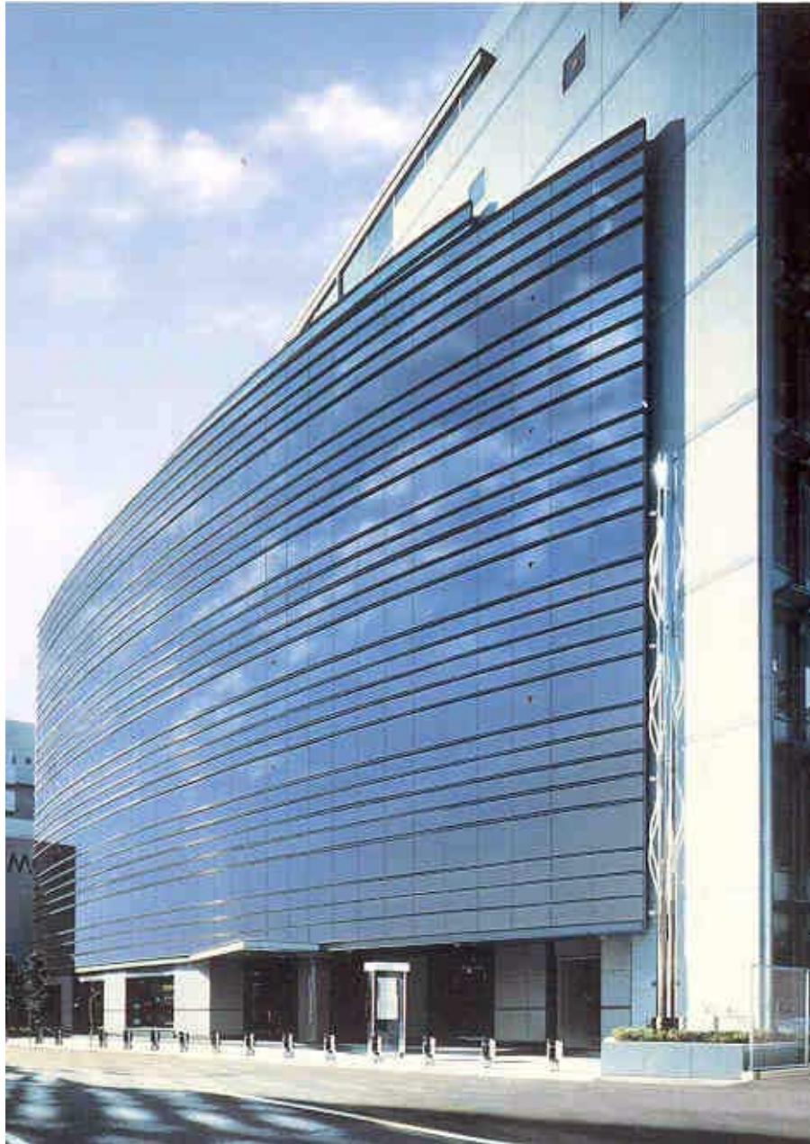
a)View of building
