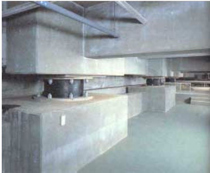
Fig. 5.7: Rubber bearing seismic isolation system.
