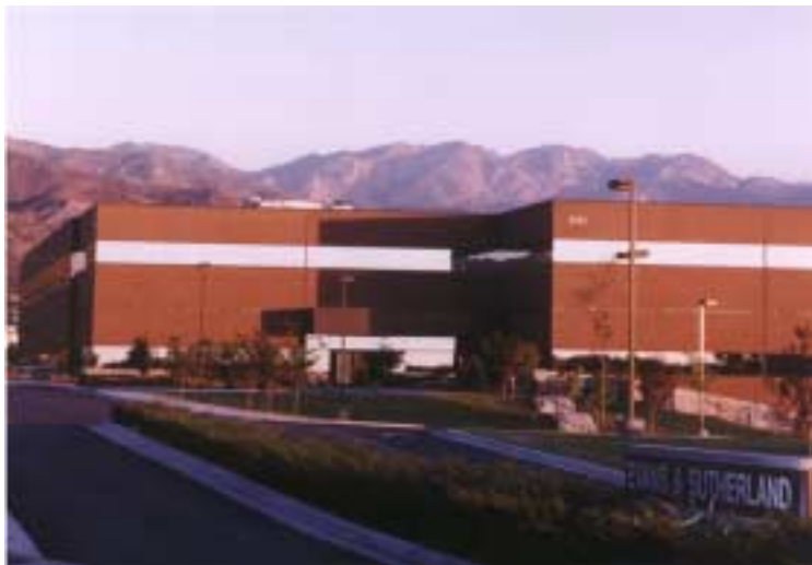
Fig. 5.21: Evans and Sutherland Facility
