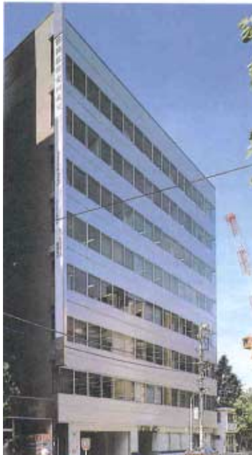
Fig. 5.24: Bridgestone Toranomom Building
