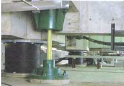
Fig. 5.13: Steel rod damper combined with a NRB.
