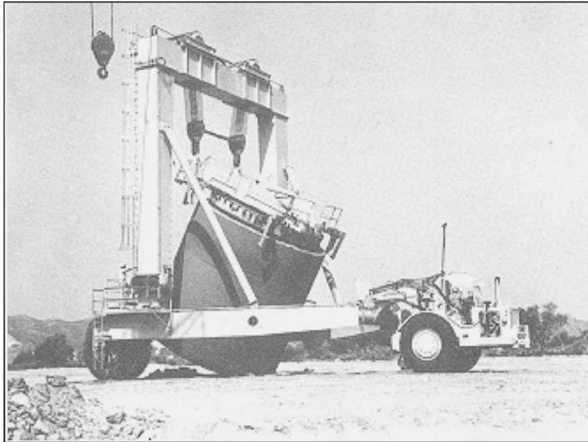
Figure 13-6 Specialized equipment for handling and transporting 252-in. (6,400-mm) (ID) pipe weighing 225 tons (204 metric tons) each
