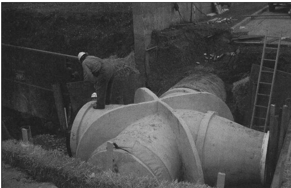
Figure 2-9 Installation of a large-diameter wye with reducer attached
