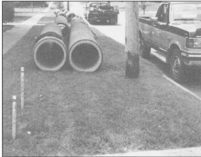
Figure 17-2 24-in. (600-mm) lined cylinder pipe strung along a right-of-way
