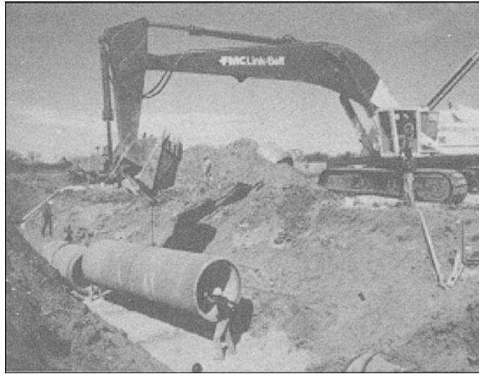
Figure 14-4 Pipe being laid on granular foundation
