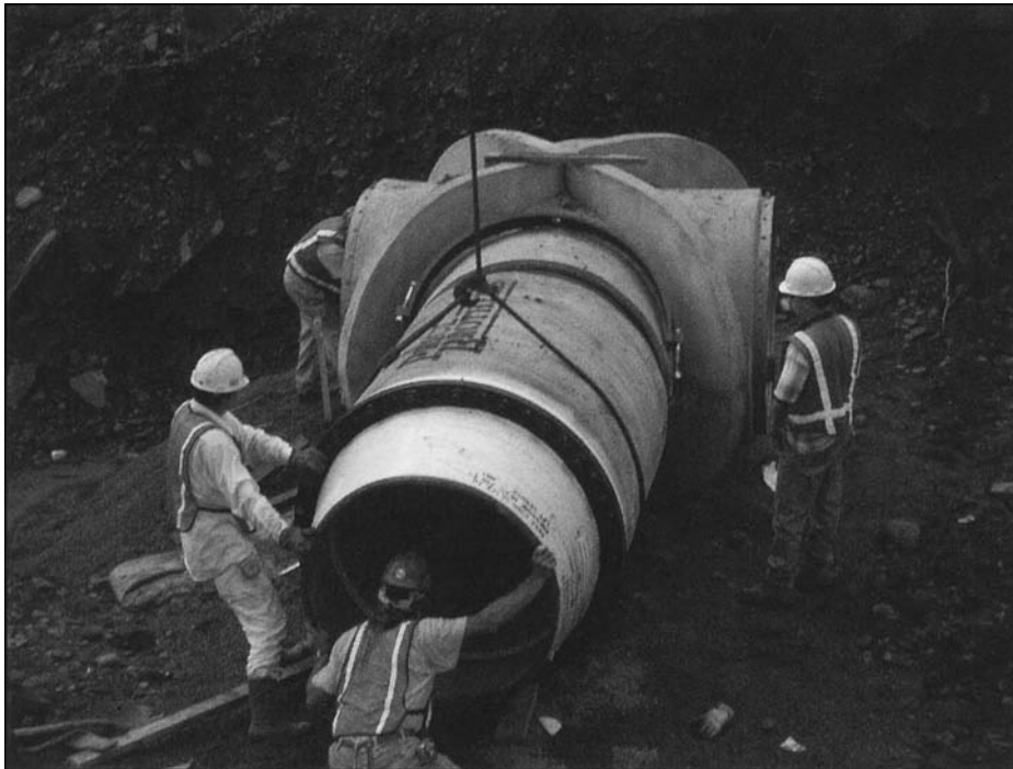
Figure 8-4 A tee or cross is used for 90° lateral connections
