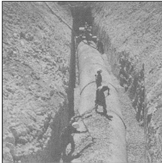
Figure 14-4 Pipe being laid on granular foundation
