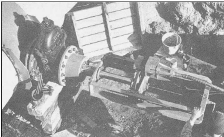
Figure 16-4 Large-diameter tapping assembly
