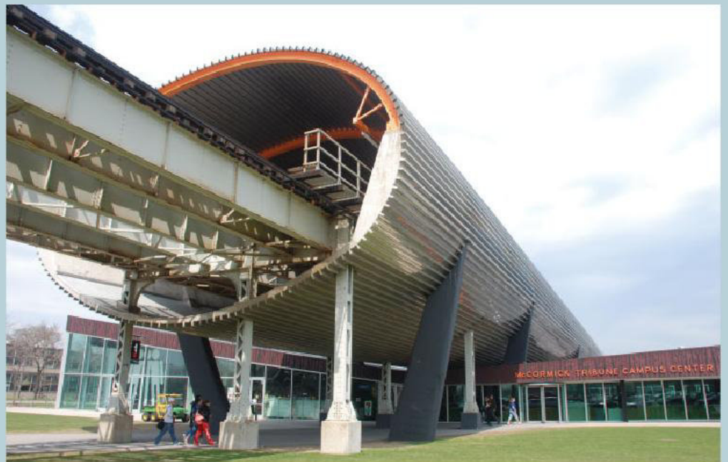
The building slides underneath the elevated railway's sound-absorbing tube.
