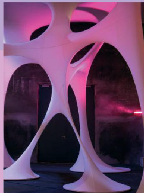
Chris Bosse, Entry Paradise Pavilion, Zeche Zollverein, Essen, Germany, 2006 The form of the membrane was produced through an iterative series of simulations, including a space-packing algorithm that subdivides the whole volume. The spatial model was then developed as a continuous minimal surface, and optimised for the cutting pattern using sail-making software. The 500 cubic metres (17,657 cubic feet) of membrane weighs only 17 kilograms (37.5 pounds), and can be put up or taken down in one hour.
