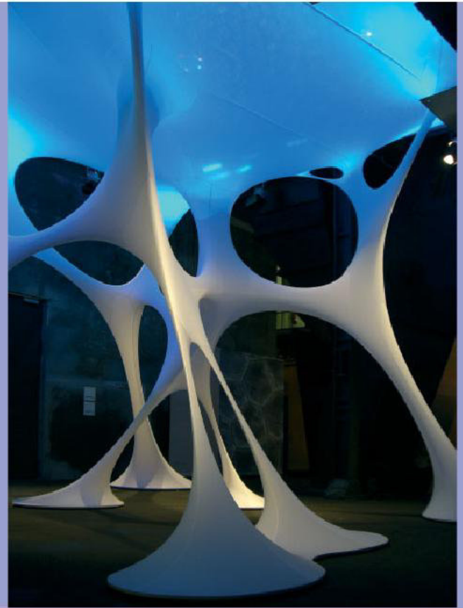
Chris Bosse, Entry Paradise Pavilion, Zeche Zollverein, Essen, Germany, 2006 The form of the membrane was produced through an iterative series of simulations, including a space-packing algorithm that subdivides the whole volume. The spatial model was then developed as a continuous minimal surface, and optimised for the cutting pattern using sail-making software. The 500 cubic metres (17,657 cubic feet) of membrane weighs only 17 kilograms (37.5 pounds), and can be put up or taken down in one hour.
