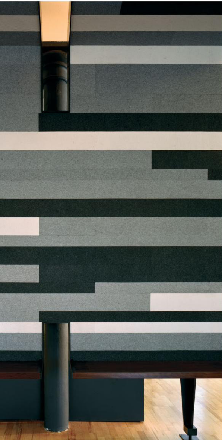
The industrial felt absorbs sound and draws an occupant's view through the length of the space, providing a self-healing material for temporary installations and exhibitions.
