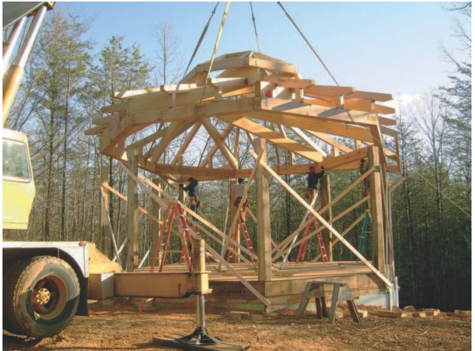
▲ 11.9 The finished skeleton. (Photo: Fred Oesch.)
