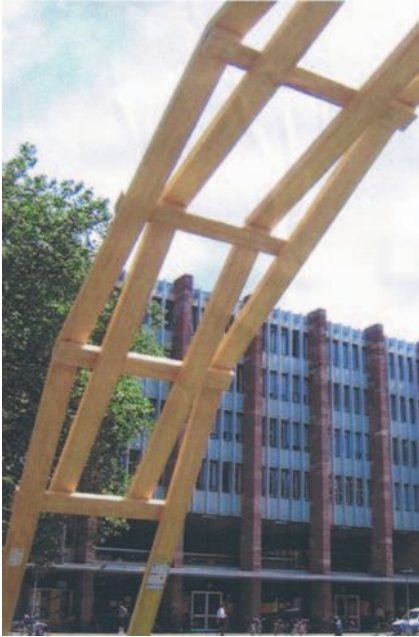
▲ 3.22 Student explorations – da Vinci-like bridge design detail.
