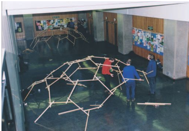
▲ 3.13 Constructing a multiple RF grid dome – 4.
