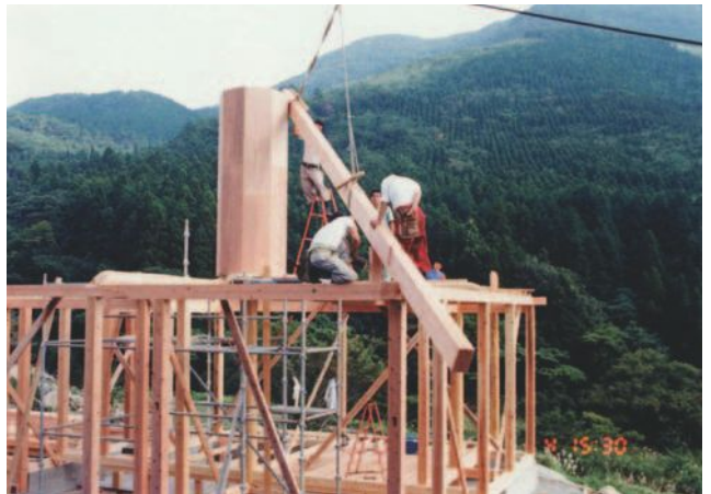
▲ 8.19 More beams are positioned around until a full circle is formed. (Photo: Yoichi Kan.)
