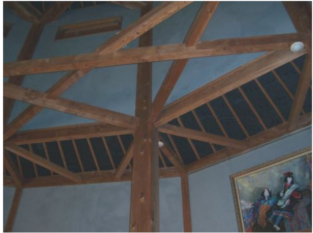
▲ 7.37 The RF-like ring beam reduces buckling.
