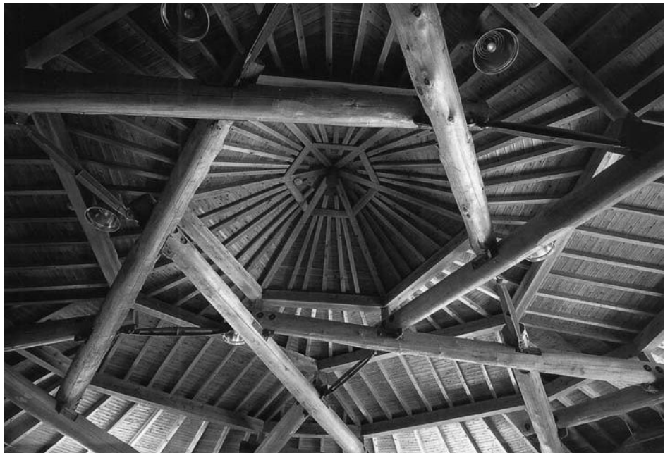
▲ 9.1 The complex round-wood structure. (Photo: Keikaku-Inc.)
