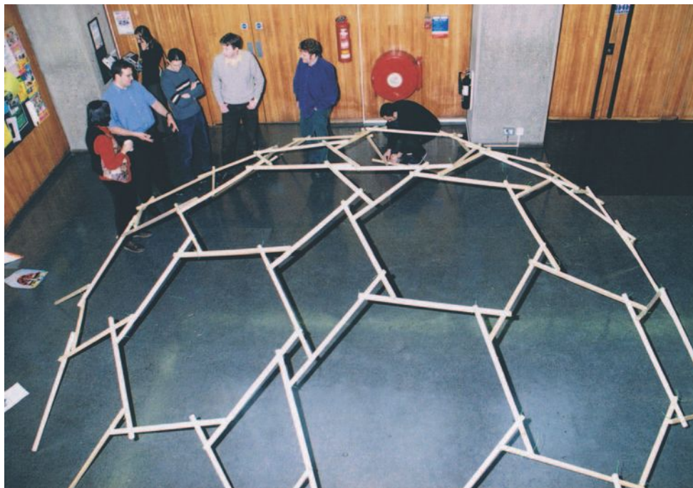
▲ 3.14 Constructing a multiple RF grid dome – 5.
