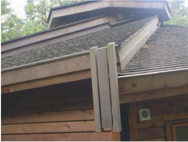
▲ 10.19 Eaves detail – front view.
