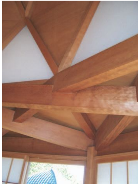
▲ 7.30 Complex notched timber connections.
