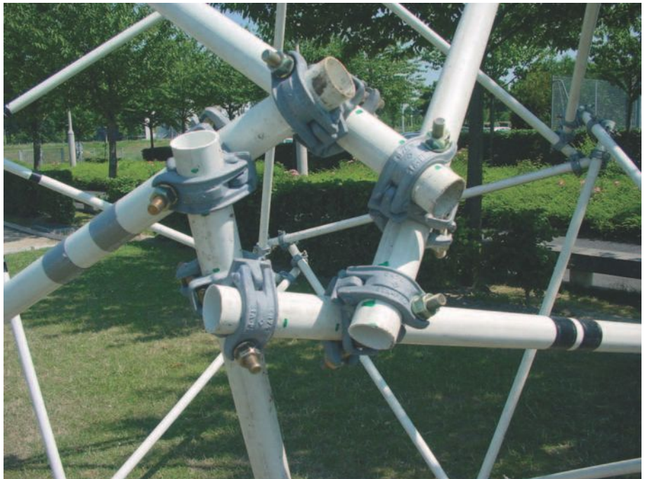
▲ 3.34 Baverel's multiple RF grid sphere – detail. (Photo: Olivier Baverel.)
