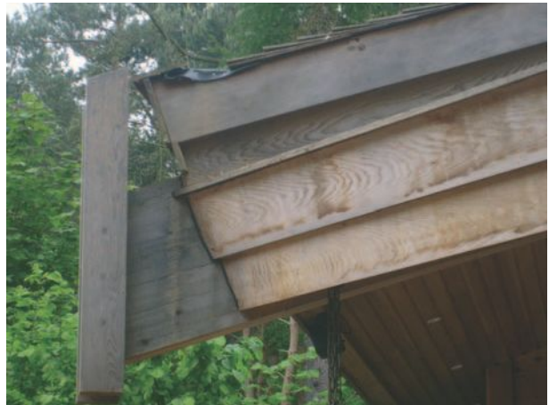
▲ 10.18 Eaves detail – side view.
