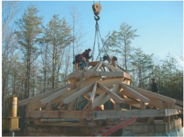
▲ 11.8 Fitting the roof light. (Photo: Fred Oesch.)
