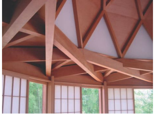
▲ 7.28 The double spiralling RF structure supports a geodesic dome.
