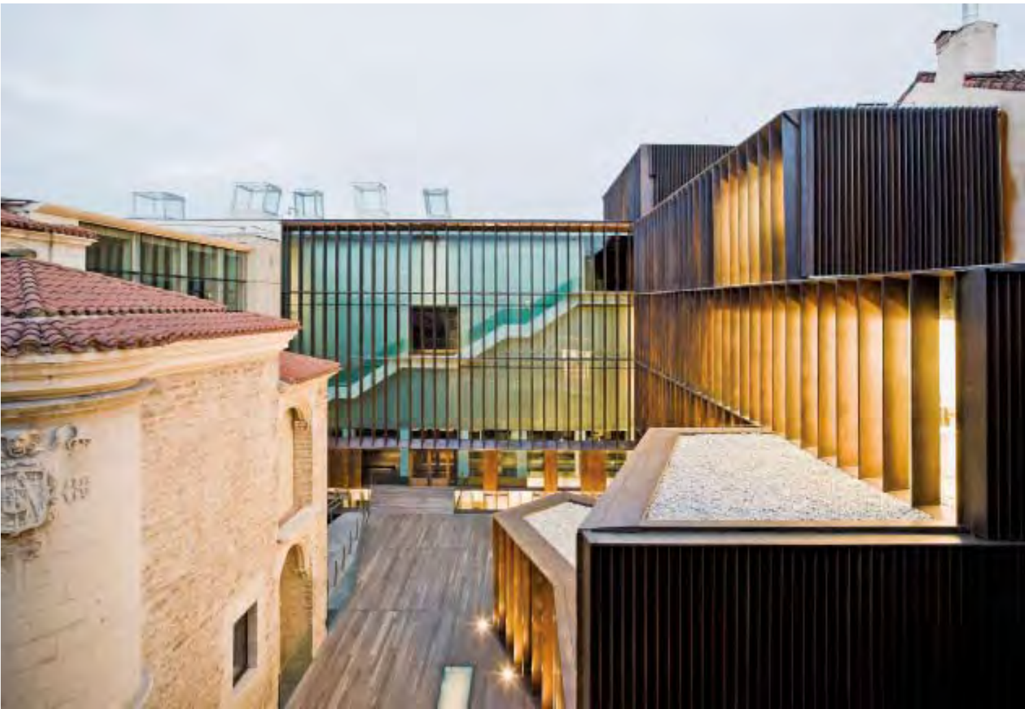
Cast bronze pieces configure the outer façades that define the access court
