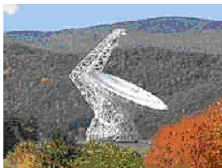
Figure 14. Green Banks 110-m offset Gregorian radio telescope, from www.gb.nrao.edu.
