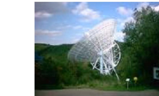
Figure 13. Effelsberg 100-m radio telescope, with homologous structural design.
