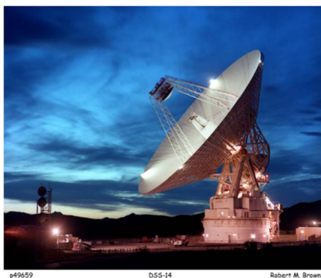
Figure 12. 70-m JPL Goldstone shaped reflector antenna.
