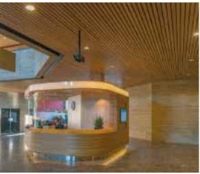
solid red oak slats are clipped onto a metal carrier system, which can be easily dismantled to access technical
