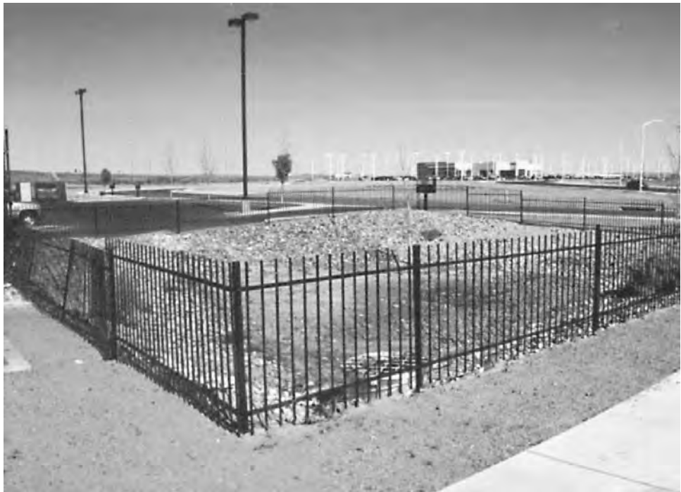
Figure 6.4 Photograph of infiltration bed in New Mexico.
