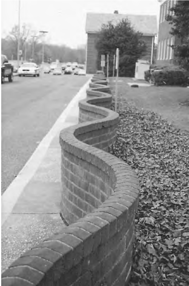
Figure 4.65 Photograph of serpentine brick wall.
