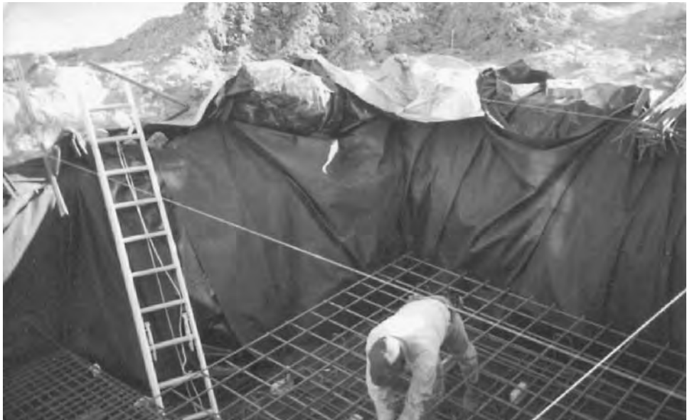
Figure 7.31 Photograph of lined foundation excavation.
