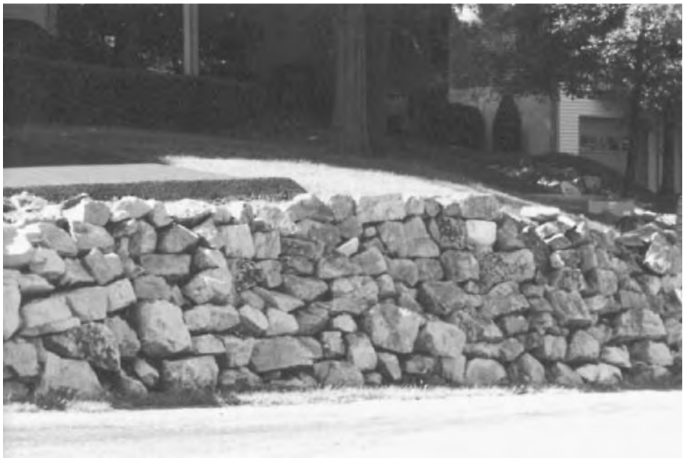
Figure 3.20 Photograph of dry laid stone wall.
