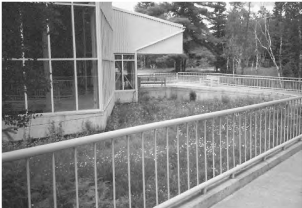
Figure 9.16 Native wildflowers were used to landscape around the protective structure in Petroglyphs Provincial Park, Ontario, Canada.
