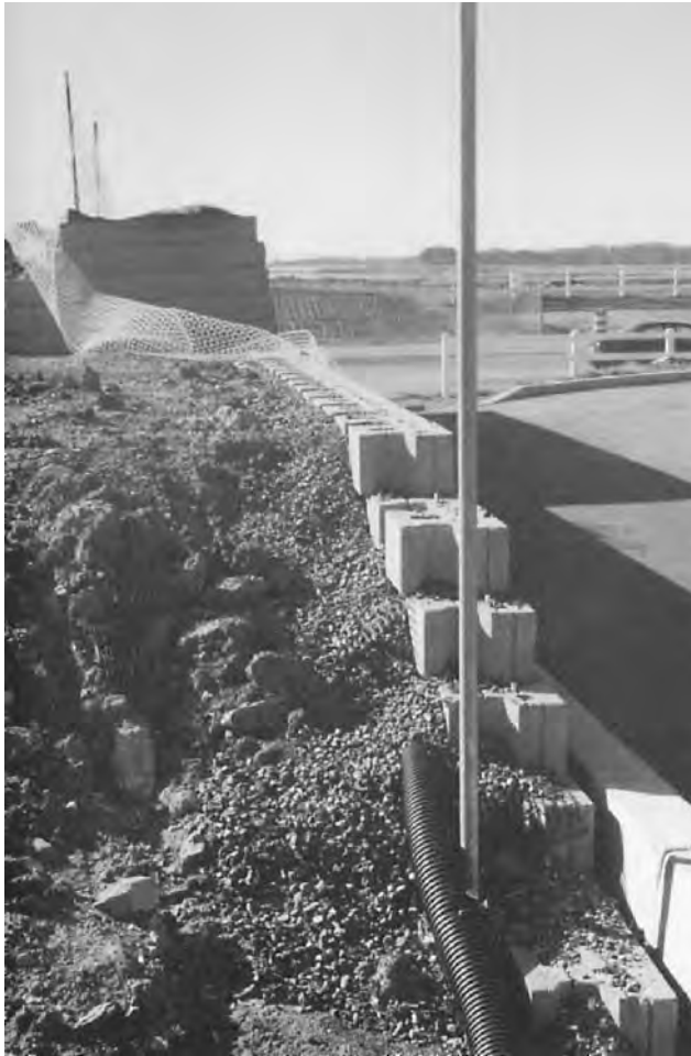
Figure 3.16 Photograph of interlocking walls.
