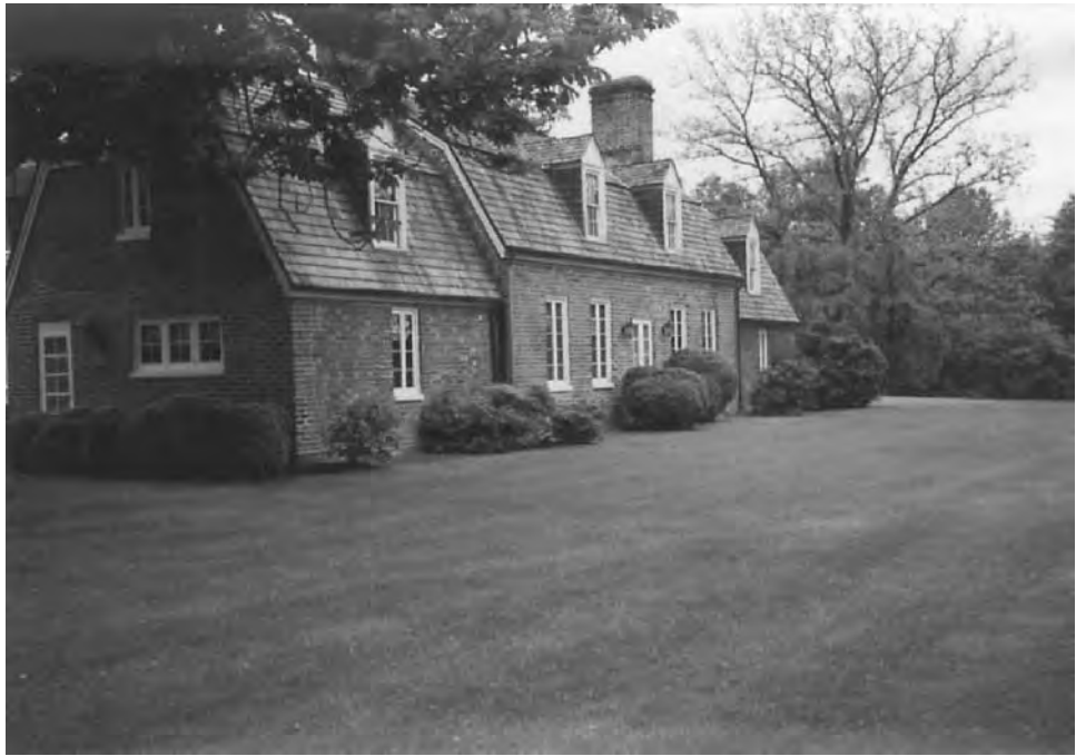
Figure 11.2 Foundation plantings were not used at the time this house was built in the 1600s in Maryland.
