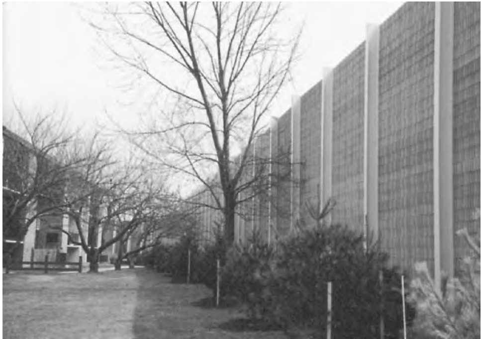
Figure 3.8 Photograph of sound walls.
