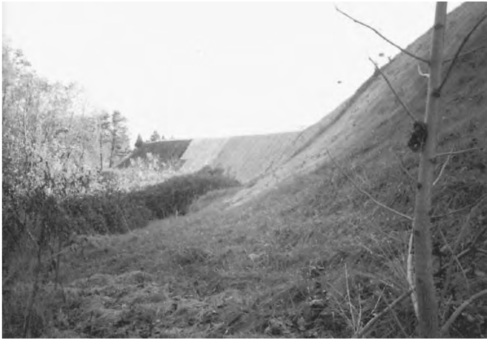
Figure 3.24 Photograph of stabilized slope.
