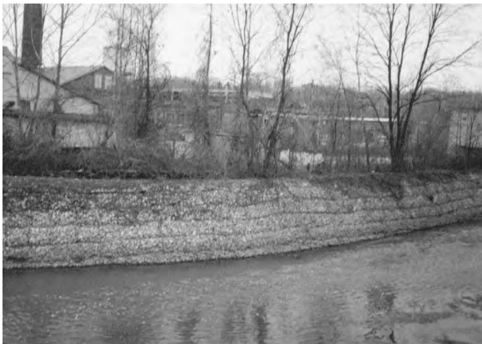
Figure 7.23 Photograph of a gabion-stabilized stream.
