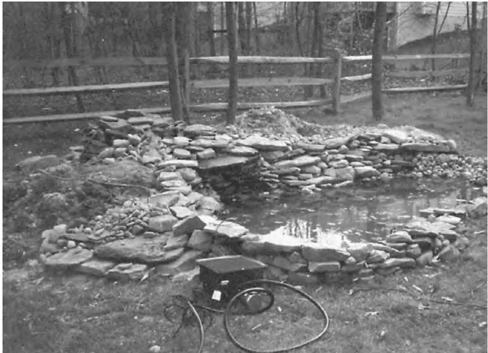
Figure 4.68 Photograph of pond installation.
