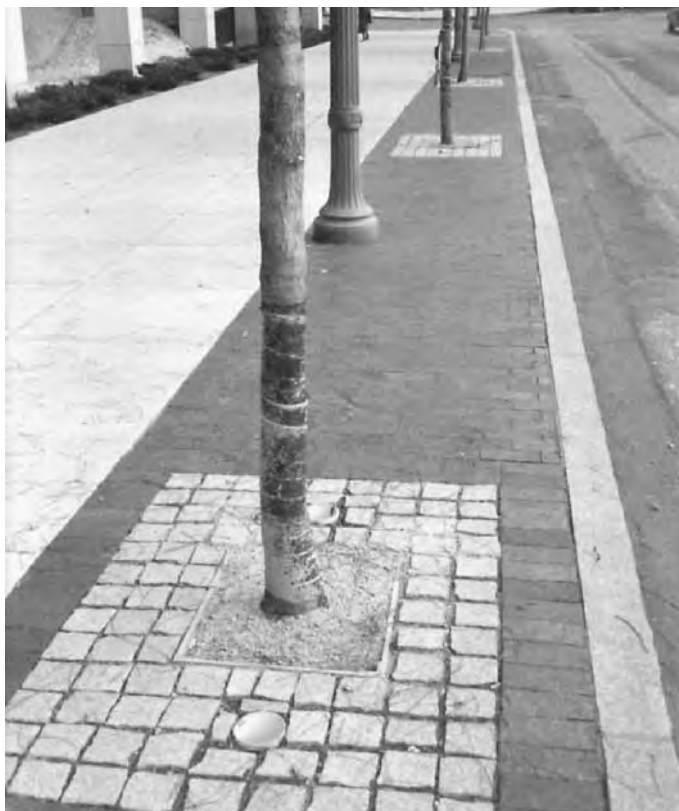
Figure 9.27 Photograph of pavers installed over the root zone of trees.
