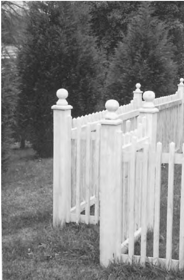
Figure 4.53 Photograph of picket fence corner detail.
