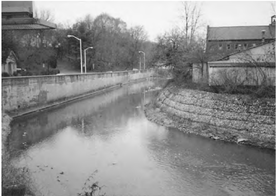
Figure 3.22 Photograph of gabion wall.
