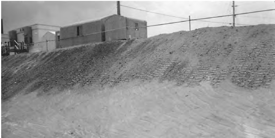
Figure 3.4 Photograph of roughened surface.
