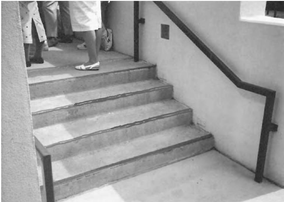
Figure 4.6 Photograph of stair treads with painted nosing.
