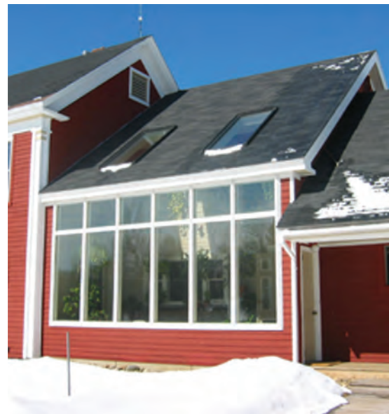
FIGURE 5.5 The sunspace serves as a bright, cheerful entrance to a two-story colonial house. Tall vertical glazing faces south to capture the rays of the low winter sun.
