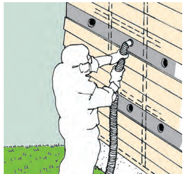
FIGURE 8.10 One way to insulate an existing home is to remove siding at intervals, drill holes in the sheathing, and blow loose fiber insulation into the cavities. The holes are then patched and the siding is replaced.
