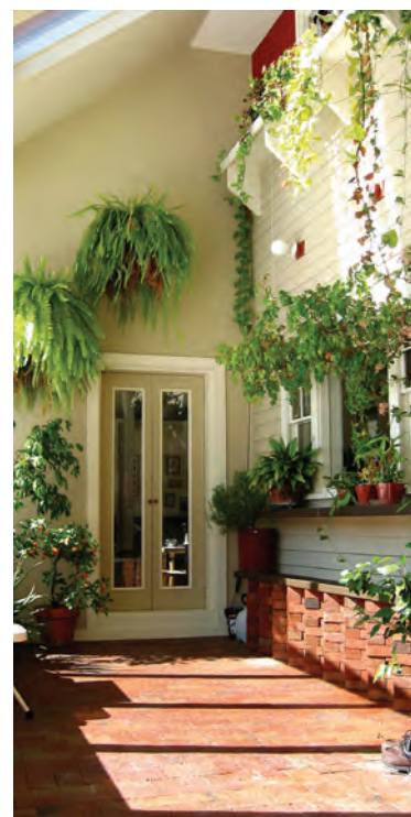
FIGURE 5.6 Plants thrive inside this sunspace without heat from the house. The brick floor and rear wall absorb solar heat during the day and slowly release it at night to keep the interior warm.
