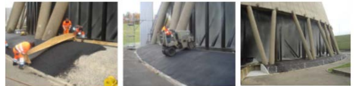
Figure 4: Modification of the air inlet around the tower basin of the NPP Leibstadt
