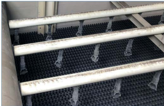
Figure 6: The bottom of the existing nozzles was found to less than 10" from the top of the fill section.
