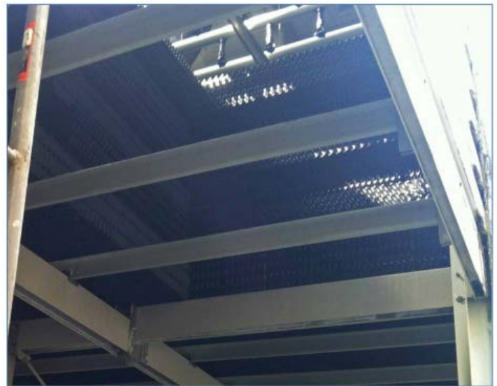
Figure 9: The existing tower had a fill fill depth of seven feet which was found to be detrimental to airflow.
