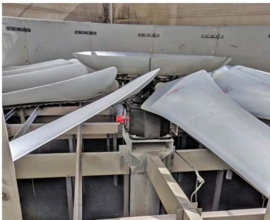
Figure 15: New mechanical equipment installation with adapter plate.
