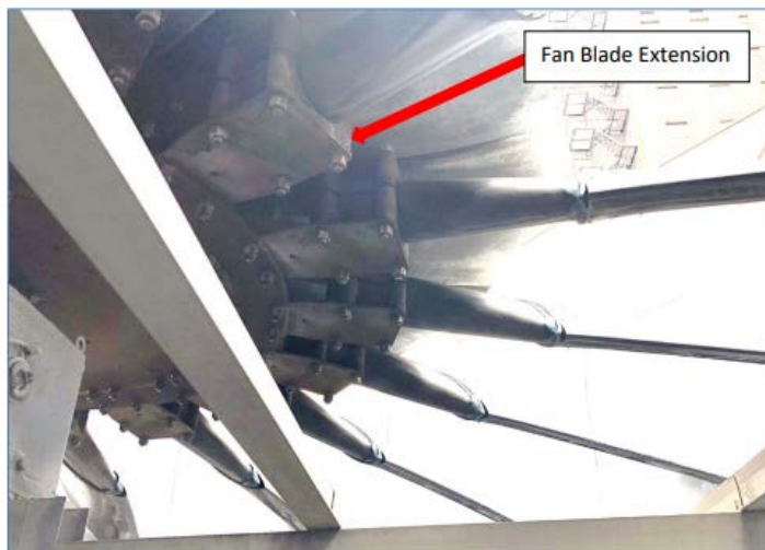
Figure 7: The existing fan assembly employed blade clamp extensions to increase the diameter of the fan assembly.
