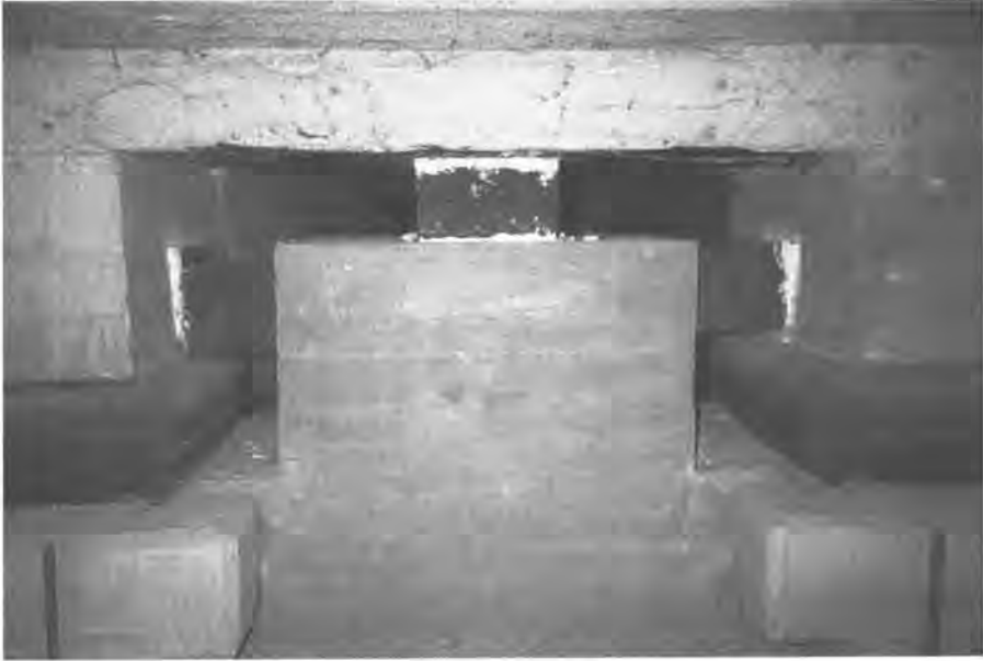
Fig. 1.3 Seismic fuzes used in the Pestalozzi School.
