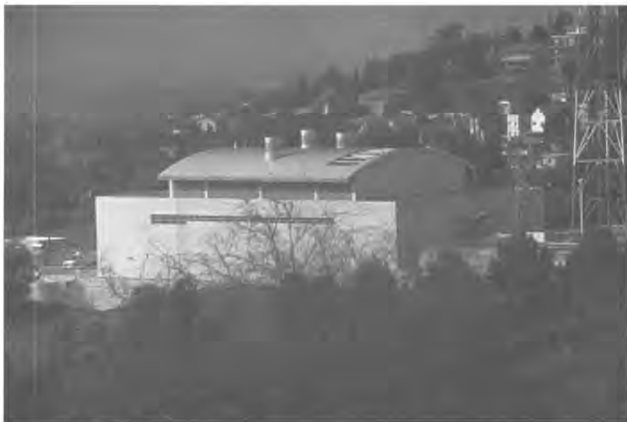
Fig. 1.6 Emergency Operations Center, Los Angeles, California.
