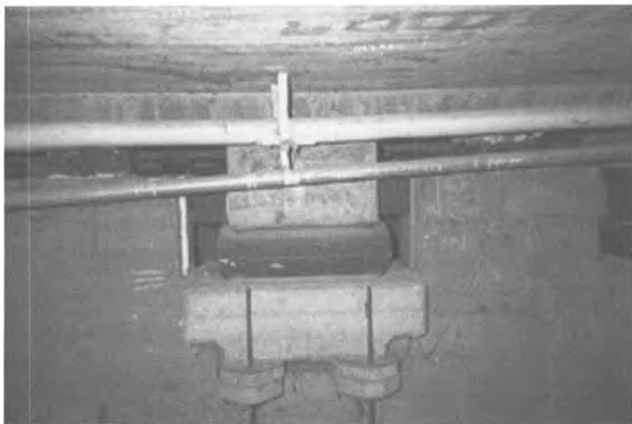
Fig. 1.2 Bearings used in the Pestalozzi School.
