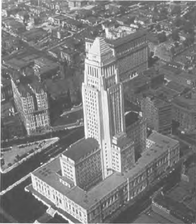
Fig. 1.12 Los Angeles City Hall.
