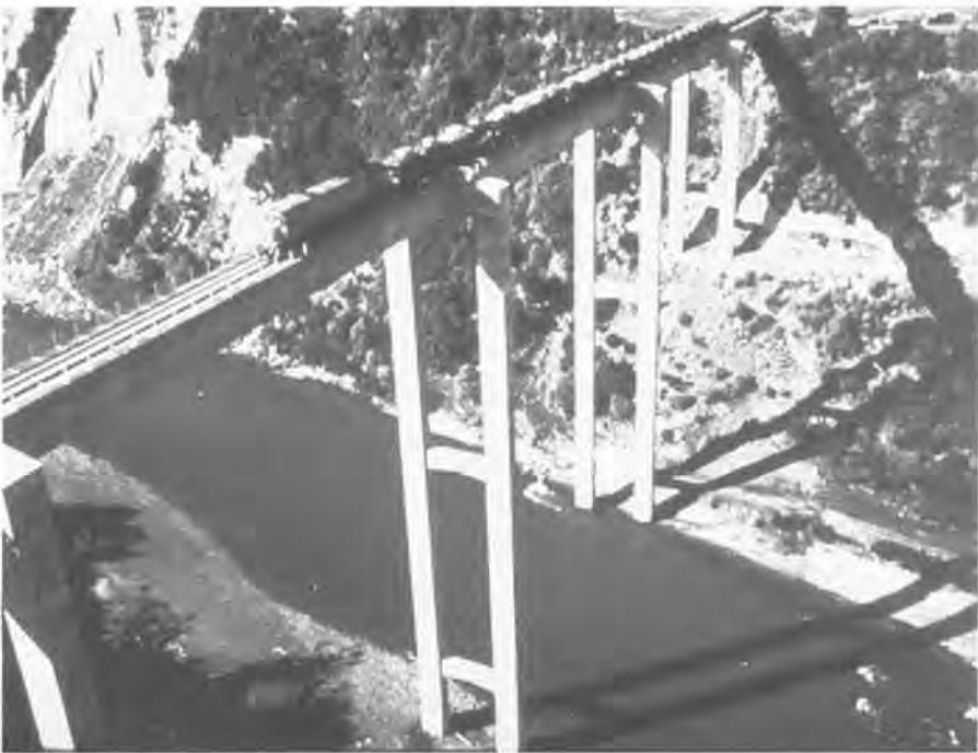
Fig. 3.11 South Rangitikei River Bridge.
