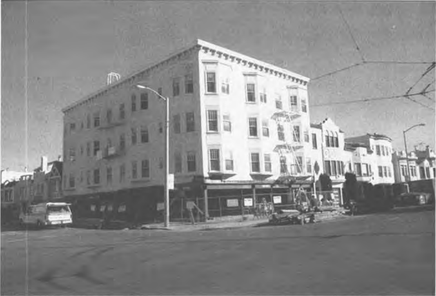
Fig. 1.14 Marina Apartments, San Francisco, California.
