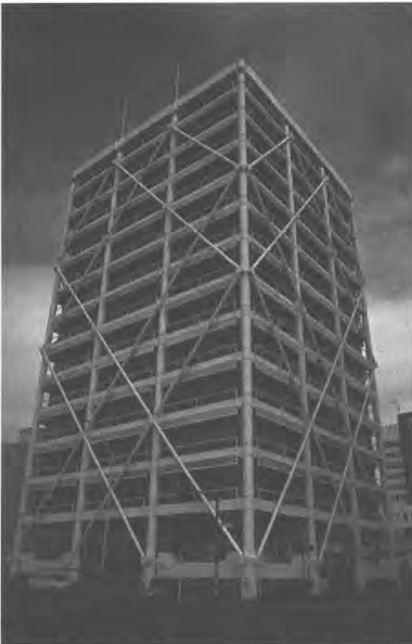
Fig. 1.19 Union House, Auckland, New Zealand.
