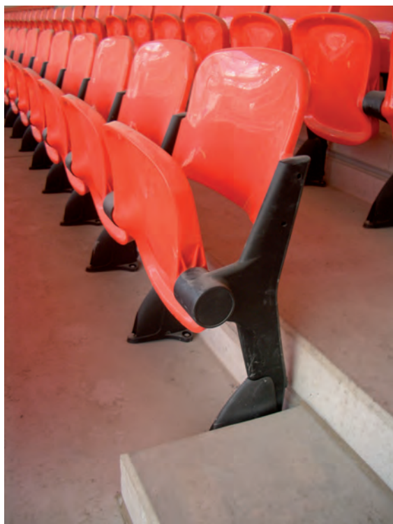
Figure 12.3 Tip-up seats can cost more than other types, and can be less robust, but they are becoming the norm.
