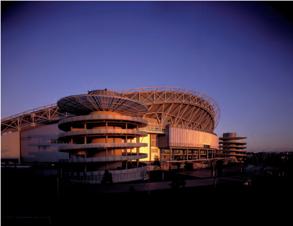
Figure 14.5 Circular ramps in Telstra Stadium Sydney (the Sydney 2000 Olympic stadium) – see also Figure 5.6b and Appendix 3.
