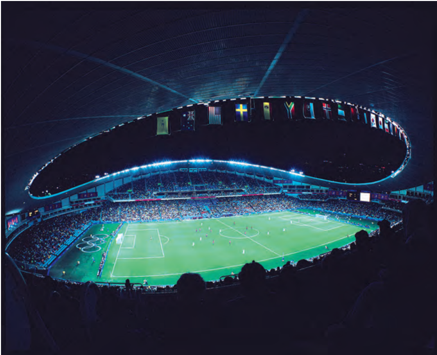
Figure 5.5 Sydney Football Stadium in Australia is a well-resolved overall design. The stands are deepest and highest where most people want to sit, and the roof sweeps gracefully round the field. Architects: Philip Cox Richardson Taylor & Partners.
