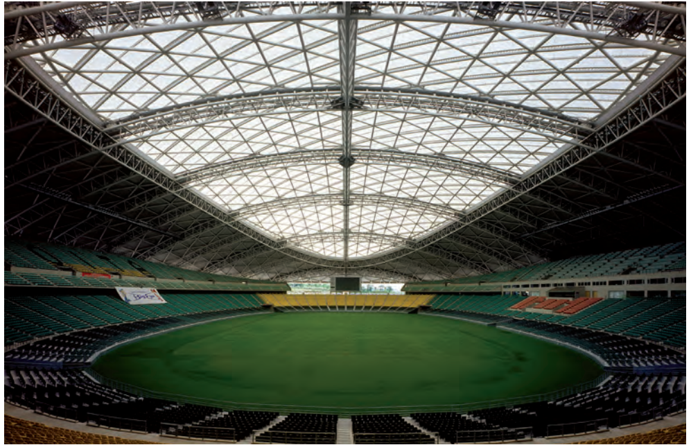
Figure 5.14 The Oita Stadium in Japan (see also Figure 4.5 and Appendix 3) has a particularly neat closing roof, consisting of two lightweight panels that slide together to meet above the centre of the playing field. The action is reminiscent of the closing of an eye. Architects: Kisho Kurokawa and associates.
