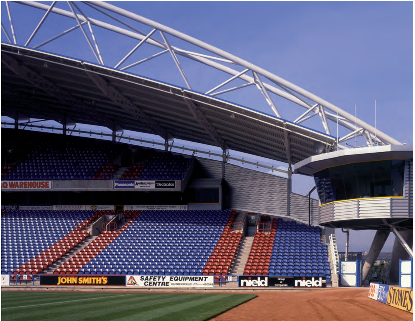
Figure 19.2 The control room at Galpham Stadium, in Huddersfield, is located to give a clear view over the playing field which cannot be obstructed by, for instance, spectators.
