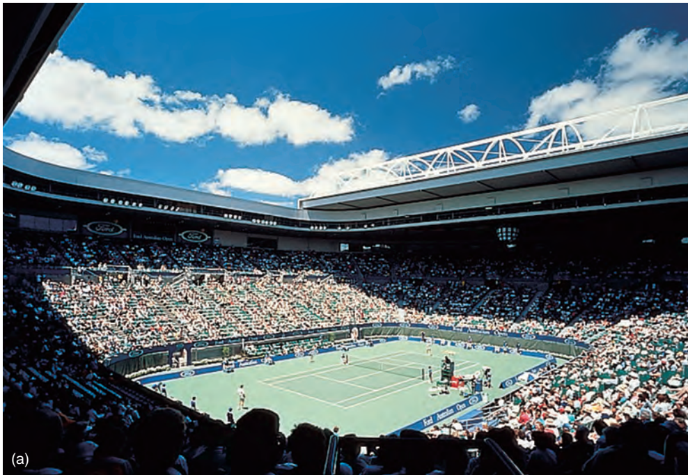
Figure 1.15a and b The Rod Laver Arena at the Melbourne and Olympic Parks, Australia (originally known as the Centre Court, Flinders Park), was a pioneering structure when built in the 1980s. Architects: Peddle Thorp & Learmonth in association with Philip Cox & Partners.
