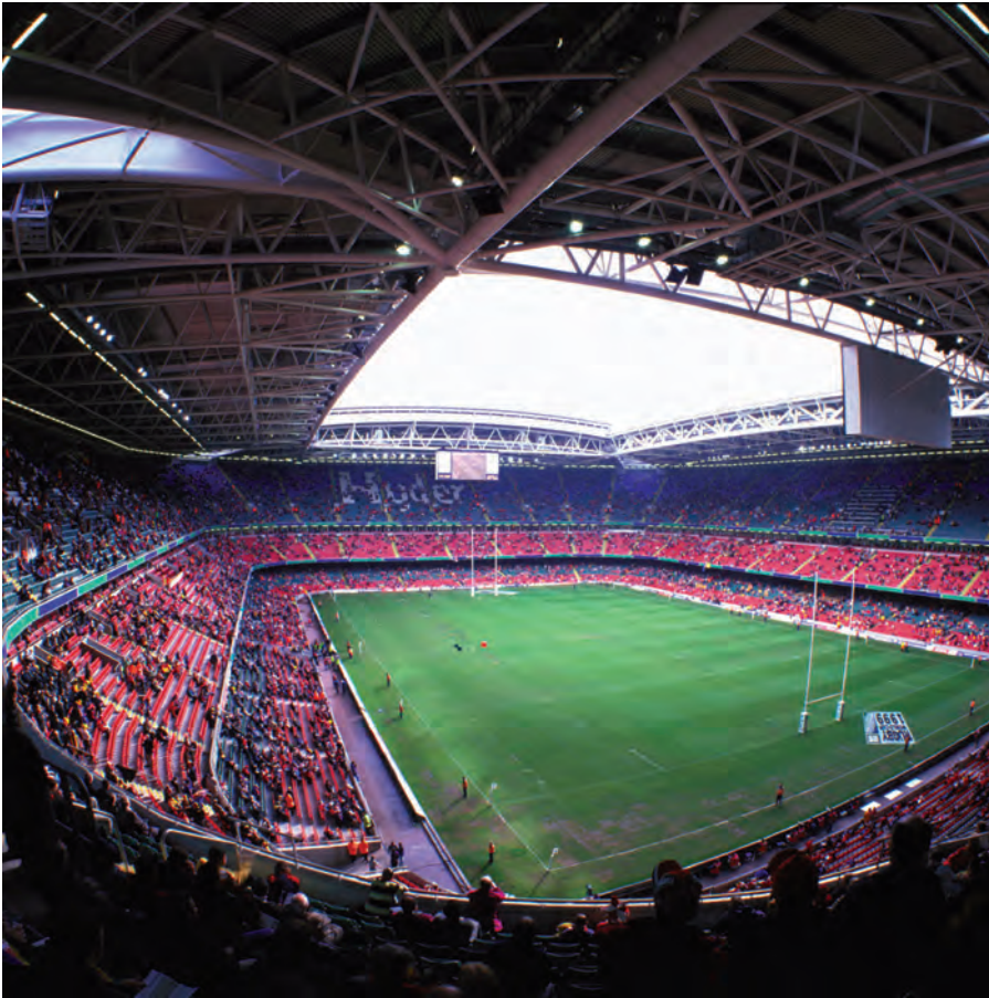
Figure 5.15 The Millennium Stadium in Cardiff, Wales (see also Appendix 3) is a pioneering example of a stadium with a very large retractable roof. Architects: HOK Sport Architects.
