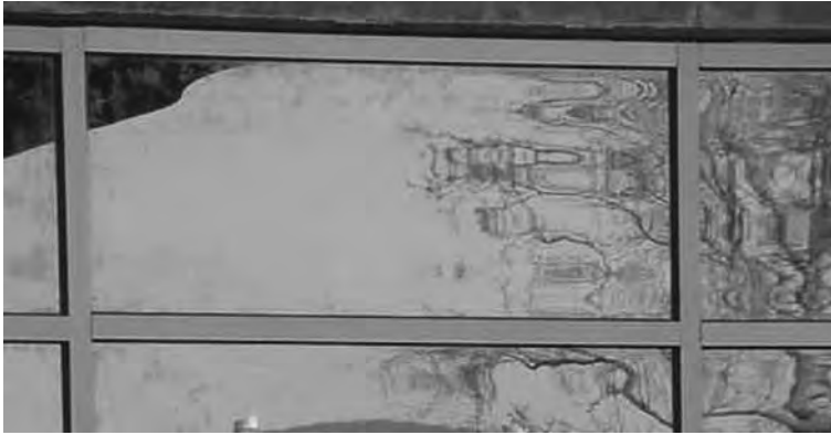
6.4 Typical reflection distortion in heat-treated glass for relatively long viewing distances.
