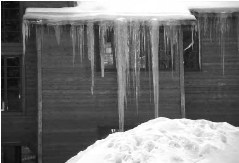
3.17 Snow up against building. Note: top of window just above ground snow. Window head is \pm 10 feet (3.048 m) above grade (Matrix IMA Archive photograph).
