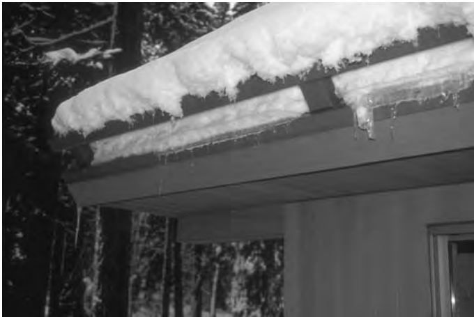
3.12 Structurally designed snow arrester. Note: heat tracing in gutter not powered at time of photo (Matrix IMA Archive photograph).
