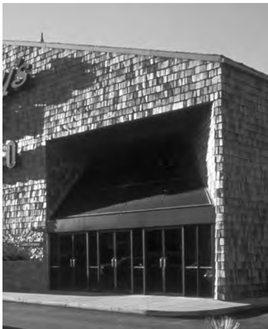
3.9 Fully sheltered sloped glazing entry below main roof rake (Matrix IMA Archive photograph).
