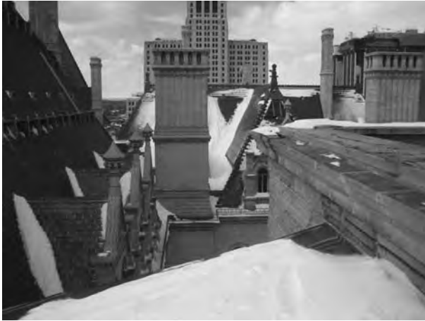
4.2 Gutters and drainage trough waterproofing height must be sized based on an anticipated height of snow accumulation.
