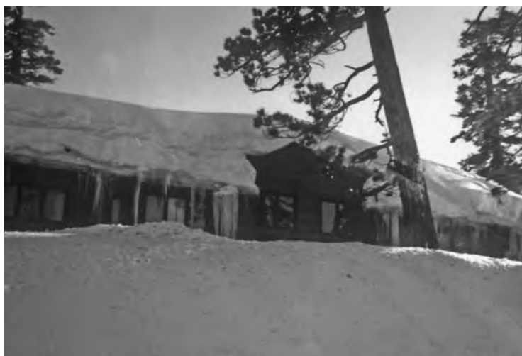
3.10 Massive unbalanced drift snow on north facing 5 to 12 warm roof. Note: sun and wind from south (Matrix IMA Archive photograph).
