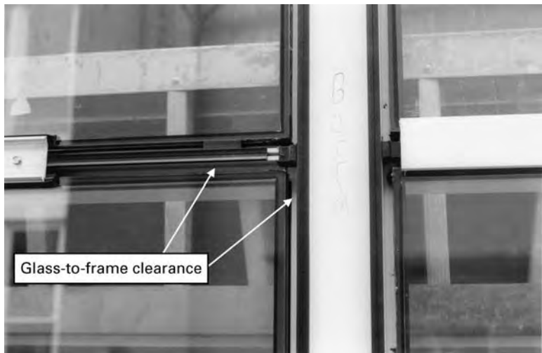
2.8 Typical glass-to-frame clearance.
