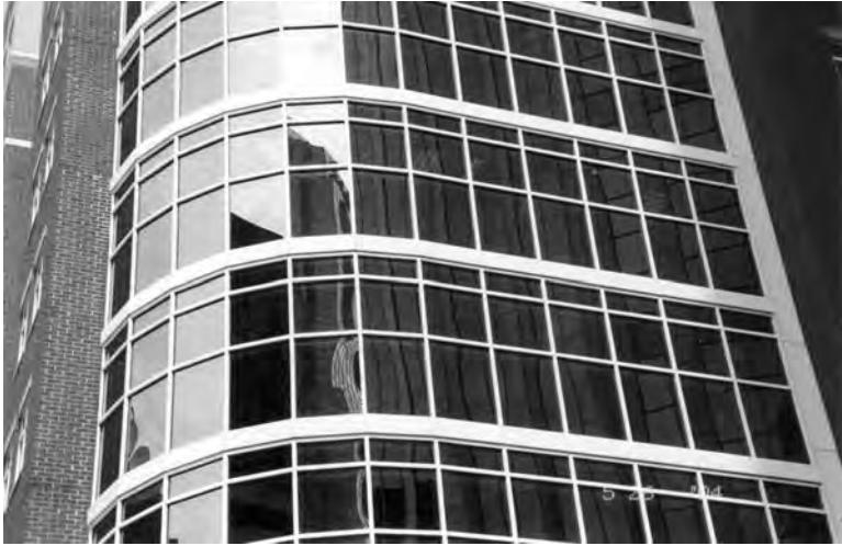
2.3 Typical dry-glazed curtain wall system.
