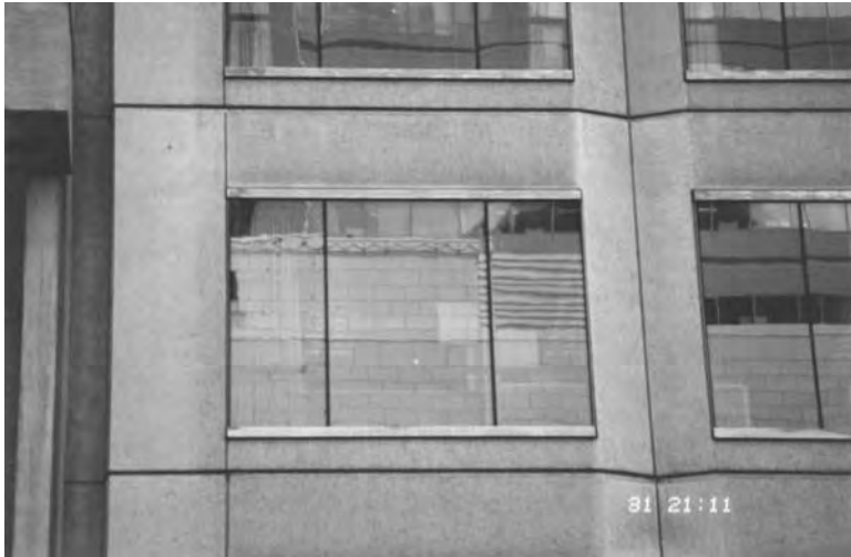
2.5 Typical punched window glazing system.
