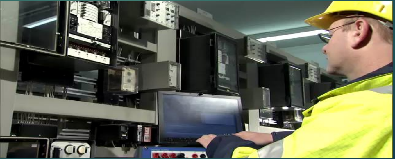
Set-up system configuration of a numerical protection system (Beckwith M-3425)
