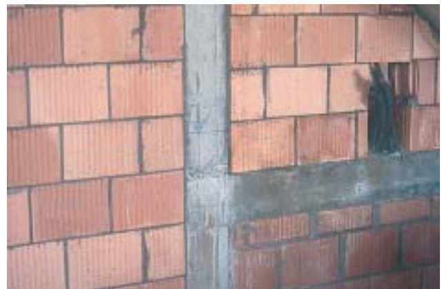
12/5 This is why it is recommended to fill in the joints between structural masonry walls and reinforced concrete structural walls with mortar (Switzerland 2001).
