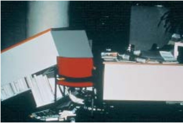
35/4 Filing cabinets can tip over, particularly if the drawers are not secured (Morgan Hill, California 1984).
