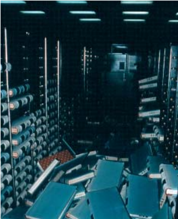
35/5 Open bookshelves empty themselves at each strong earthquake. Valuable books can be secured by the use of retaining bars or inclined shelves (Loma Prieta, California 1989).
