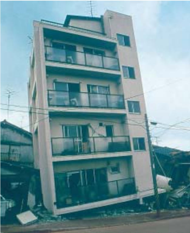
4/5 The well-braced upper part of the building collapsed onto the ground floor...
