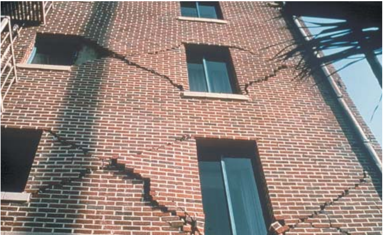
32/3 This facade cladding was insufficiently anchored and could not follow the deformations of the reinforced concrete frame structure (Northridge, California 1994).
