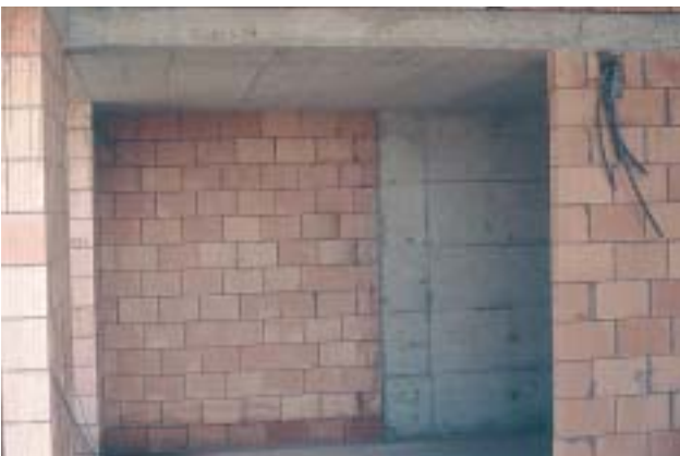
12/4 Structural masonry walls, reinforced concrete structural walls and slabs should respond together when subjected to shear, compression, and if possible tension (Switzerland 2001).
