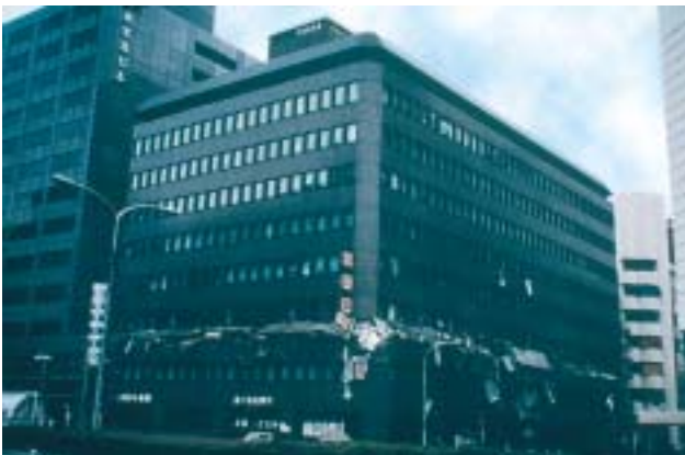
5/1 In this commercial building the third floor has disappeared and the floors above have collapsed onto it (Kobe, Japan 1995).
