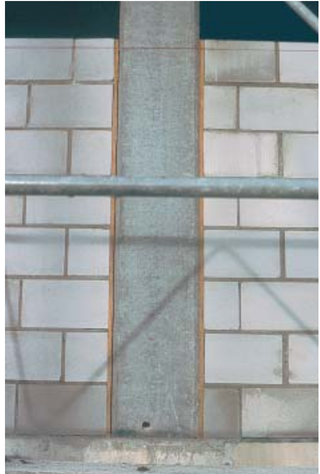
17/6 A possibility to avoid or strongly reduce the unfavourable effect of infill parapet walls into frames, is the addition of joints between the infill wall and columns. The joint was realized correctly, since it is filled by a soft and therefore strongly compactible rock wool sheet. However, the width only permits a 1% free lateral drift ratio of the column (Switzerland 2001).
