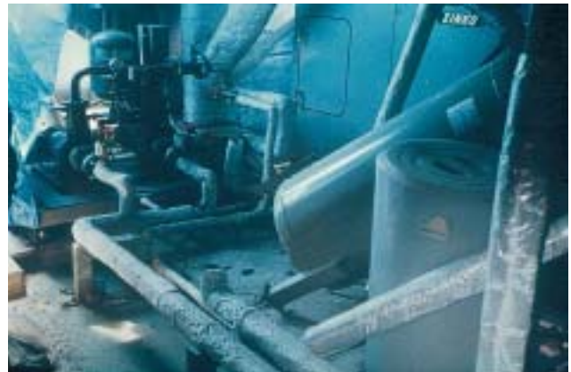
35/2 Containers and machines can tilt if they are not sufficiently anchored (Kobe, Japan 1995).
