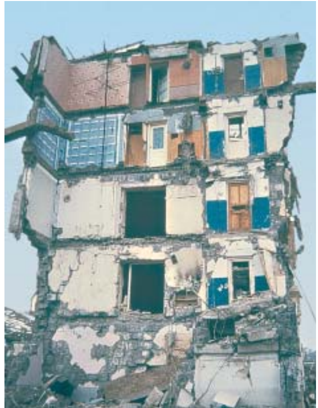
22/2 22/3 In these houses also, the slabs consisted only of precast elements, which were insufficiently connected between each other and with the walls (Armenia 1988).
