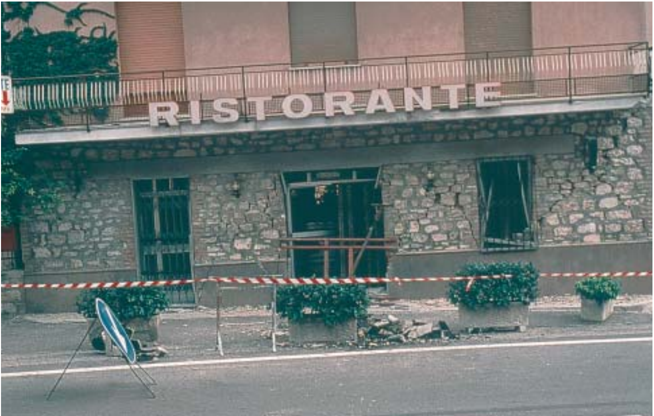
16/2 Here, the masonry columns in the ground floor of a restaurant behaved as short columns. They were highly damaged by diagonal cracks (Umbria, Italy 1997).
