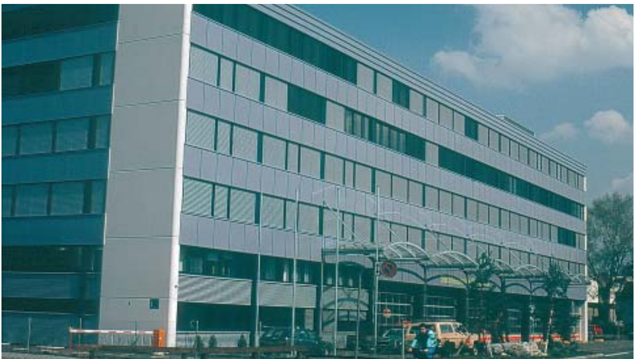
9/4 The structural walls were included as prominent elements in the architectural concept (Switzerland 1994).
