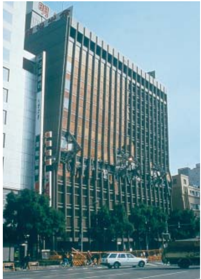
5/2 In this office building also, an upper storey failed. The top of the building has collapsed onto the floor below, the whole building rotated and leaned forwards.
