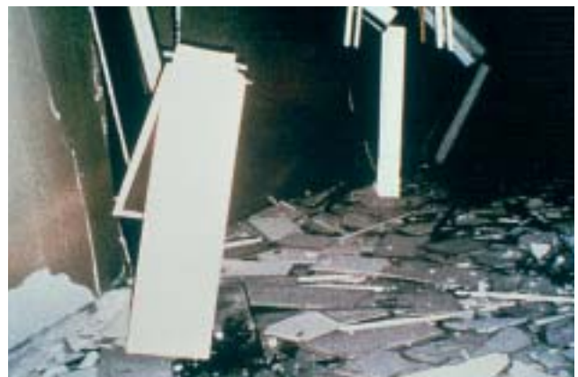
34/3 34/4 Poorly fastened light fittings, such as these, can fall and endanger people (San Fernando, California 1971).
