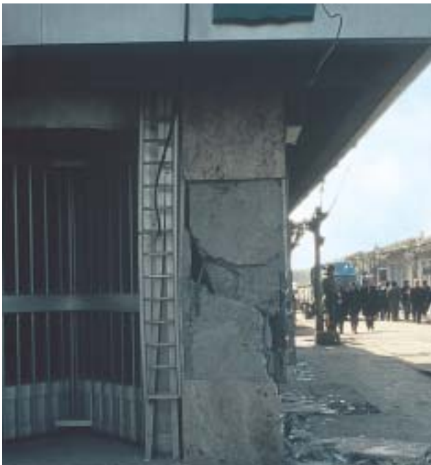
16/2 Here, the masonry columns in the ground floor of a restaurant behaved as short columns. They were highly damaged by diagonal cracks (Umbria, Italy 1997).
