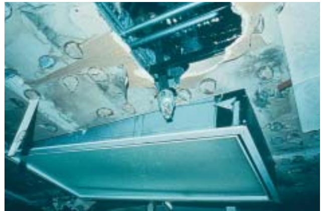
34/2 ... that hang from thin wires only constitute a safety threat to people (Northridge, California 1994).
