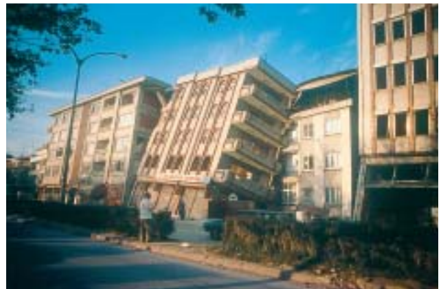
30/2 This inclined building sank unevenly and leans against a neighbouring building (Turkey, Izmit 1999).
