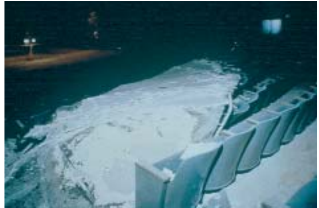
34/2 ... that hang from thin wires only constitute a safety threat to people (Northridge, California 1994).
