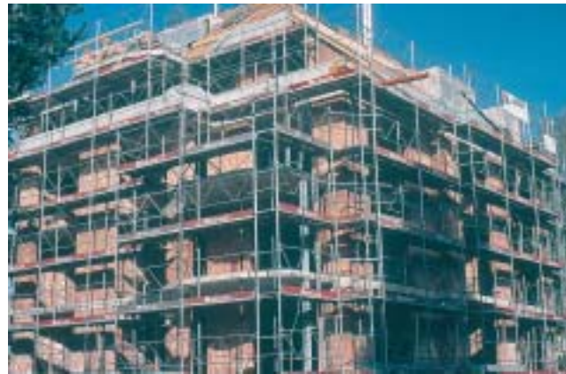
12/1 Such – and also lower! – new masonry structures, without bracing reinforced concrete structural walls, are extremely vulnerable to earthquakes (Switzerland 2001).
