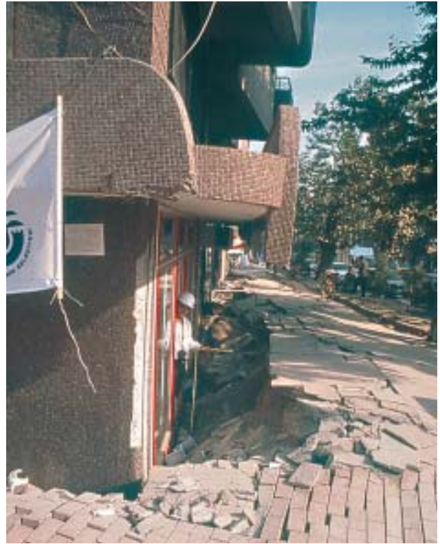
30/1 This building sank evenly about 1 m due to soil liquefaction. The displaced soil caused a bulge in the road (Izmit, Turkey 1999).
