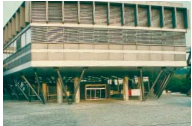
6/5 Originally, the only horizontal bracing in this 70's auditorium building at the Hönggerberg Campus of ETH Zurich were reinforced concrete walls with little torsional resistance situated at the rear of building. Because of the considerable distance between the bracing and the centre of mass of this large building, it would have twisted significantly in the plan for even a relatively weak earthquake (seismic zone 1 according to SIA 160). The few highly loaded reinforced concrete columns in the ground floor would have experienced substantial displacements, particularly in the front of the building. However, the column detailing was inadequate for the required ductility. Additional steel columns were therefore built in on three sides of the building exterior. They form a truss that can transfer the horizontal seismic forces to the existing foundations. This upgrading also fulfilled the need for a strengthening of the cantilevered structure for gravity loads.
