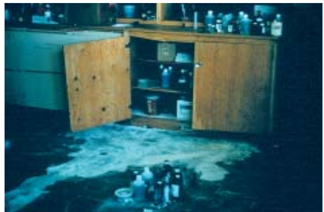
35/3 In this chemistry laboratory, unsecured glass containers broke when they fell from the table and through open cabinet doors (San Fernando, California 1971).
