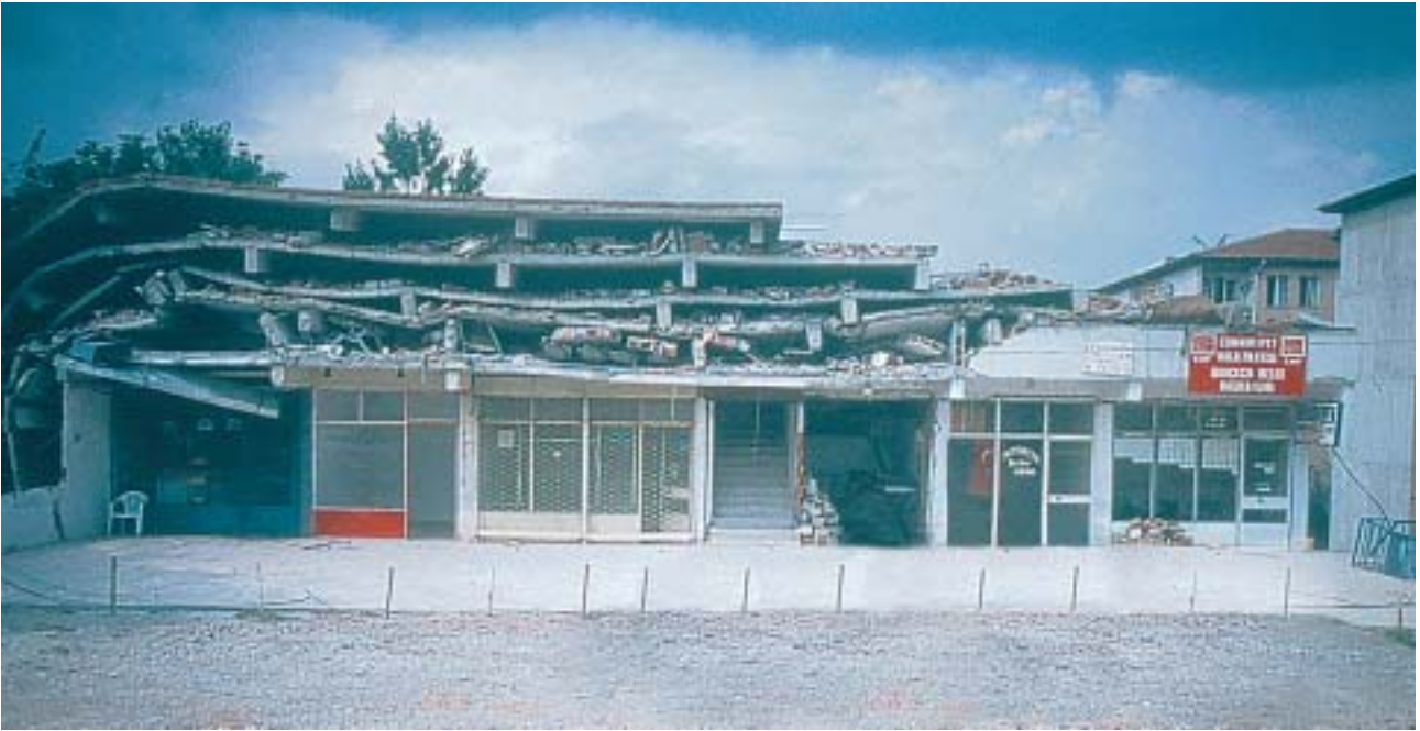
5/4 All the upper floors were too soft (Izmit, Turkey 1999).
