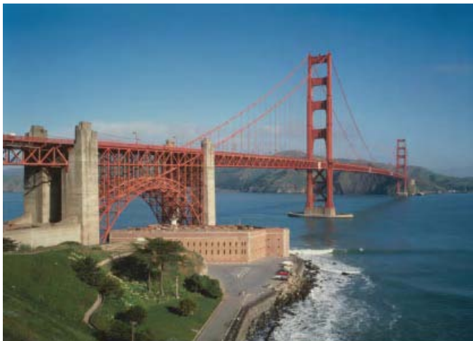
Exhibit 1.5 The Golden Gate Bridge was built across mouth of San Francisco Bay from 1933–1937 by design engineer Charles Ellis and chief engineer Joseph Strauss. Spanning one of the world’s most spectacular channels, the bridge is internationally renowned as a superb structural and aesthetic example of suspension bridge design. (Jet Lowe, 1984, HAER CA-31-43.)
