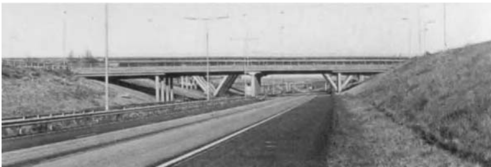
Fig. 3.14 Lack of harmony between adjacent bridges (Murray, 1991). (From Bridge Aesthetics around the World , copyright © 1991 by the Transportation Research Board, National Research Council, Washington, DC. Reprinted with permission.)
