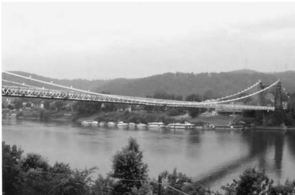
Fig. 1.11 Wheeling Suspension Bridge. (Photo by John Brunell, courtesy of West Virginia Department of Transportation.)
