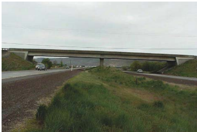
Exhibit 1.17 The I-82 Hinzerling Road undercrossing near Prosser, Washington, is a good example of the use of texture. The textured surfaces on the solid concrete barrier and the abutments have visually reduced the mass of these elements and made the bridge appear more slender than it actually is. (Photo courtesy Washington State DOT.)
