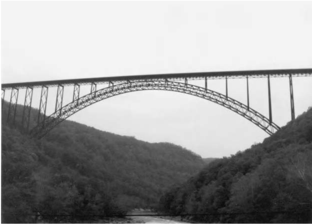
Fig. 4.1 New River Gorge Bridge. (Photo courtesy of Michelle Rambo-Roddenberry, 1996.)
