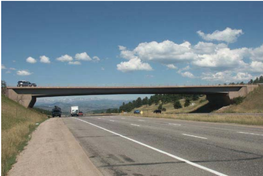
Exhibit 1.21 The Genesee Road (U.S. 40) Bridge over I-70 in Colorado is an elegant single span overcrossing with a slender appearance because the girder is in shadow and sloping lines on the abutment that invites the flow of traffic. It also provides a framework for an observer's first view of the Rocky Mountains. (Photo courtesy of Colorado DOT.)
