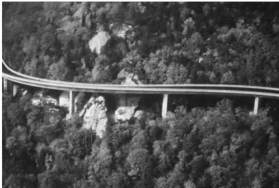
Fig. 3.16 Blue Ridge Parkway (Linn Cove) Viaduct, Grandfather Mountain, North Carolina (Gottemoeller, 1991). (From Bridge Aesthetics Around the World , copyright © 1991 by the Transportation Research Board, National Research Council, Washington, DC. Reprinted with permission.)
