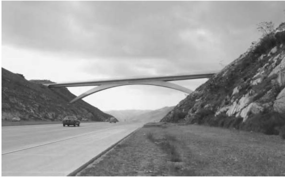
Fig. 3.15 Well-proportioned concrete arch, West Lilac Road overpass, I-15. (Permission granted by California DOT.)
