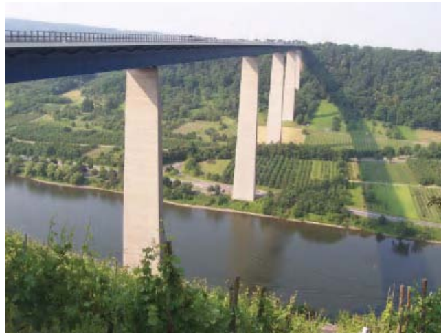
Exhibit 1.13 The bridge crossing the broad valley of the Mosel River (Moseltal-Brücke) in southern Germany is a good example of tall tapered piers with thin constant-depth girders that give a pleasing appearance when viewed obliquely.
