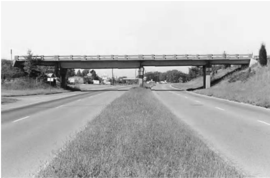
Fig. 3.9 Example of poor depth transitions and awkward configurations due to lack of superstructure continuity. (Photo courtesy of Tennessee DOT.)
