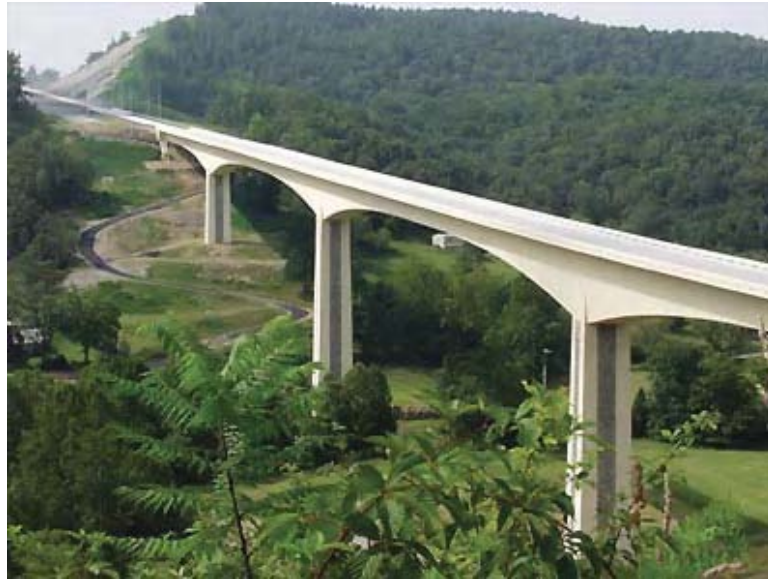
Exhibit 1.12 The Smart Road Bridge has pleasing proportions as the span lengths decrease going up the sides of the Ellett Valley near Blacksburg, Virginia. The bridge is 1985 feet long, 150 feet high, and serves the needs of researchers while protecting the scenic beauty of southwestern Virginia.
