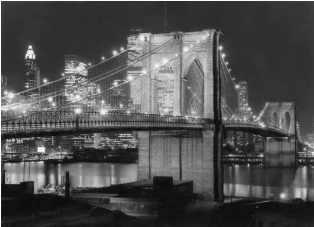
Fig. 3.19 Brooklyn Bridge, New York City. (Jet Lowe, HAER Collection, Historic American Engineering Record.)
