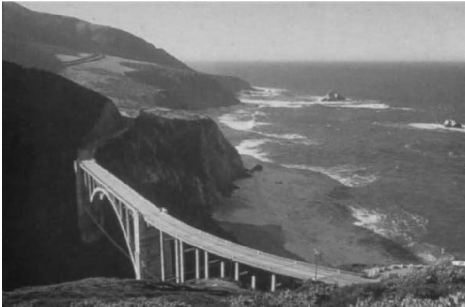
Fig. 1.14 Bixby Creek Bridge, south of Carmel, California. [From Roberts (1990). Used with permission of American Concrete Institute.]
