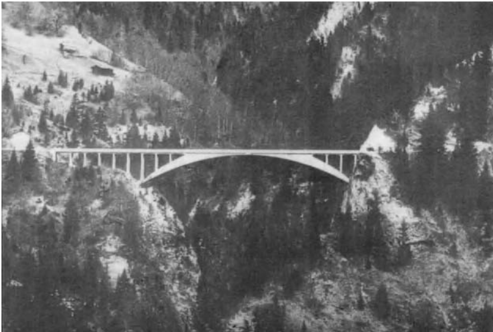
Fig. 4.2 General view of Salginatobel Bridge. [From Troitsky (1994). Reprinted with permission of John Wiley & Sons, Inc.]
