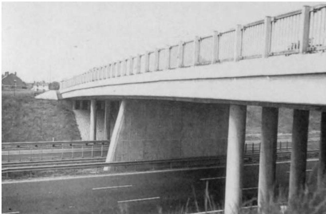
Fig. 3.37 Bridge with displeasing mixture of supports (Murray, 1991). (From Bridge Aesthetics around the World , copyright © 1991 by the Transportation Research Board, National Research Council, Washington, DC. Reprinted with permission.)
