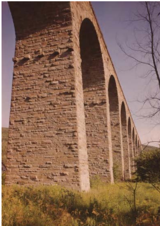
Exhibit 1.2 The Starrucca Viaduct near Lanesboro, Pennsylvania, was built in 1848 by the Erie Railway. At the time of its construction, it was the largest stone arch rail viaduct in the United States. The bridge has been in continual use for more than 160 years and still carries two tracks of the New York, Susquehanna and Western Railway. (HAER PA-6-17, photo by Jack E. Boucher, 1971.)
