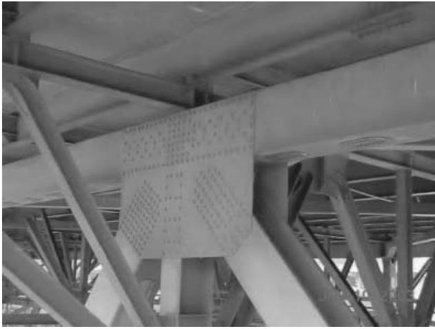
Fig. 2.15 Typical five-member node (two upper chord members, one vertical member, and two diagonal members) on I-35W Bridge (NTSB, 2008).
