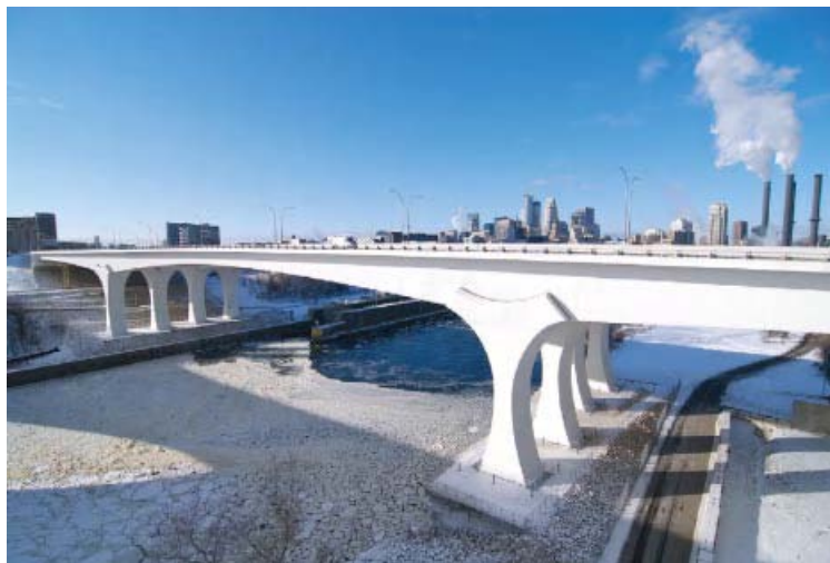
Exhibit 1.19 The I-35W St. Anthony Falls Bridge over the Mississippi River in Minneapolis, Minnesota, built in 2008 replaced the I-35W Bridge that collapsed in 2007 (see Section 2.2.7 and compare with Figure 2.14). The brightly lit girder face and sculpted piers contrast with the shadows cast by the deck overhang and the tops of the piers, accentuating the flow of the structure.
