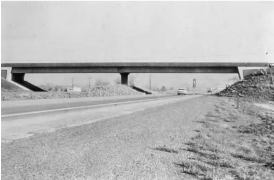
Fig. 3.20 Texture reduces visual mass, I-82 Hinzerling Road undercrossing, Prosser, Washington. (Photo courtesy of Washington State DOT.)
