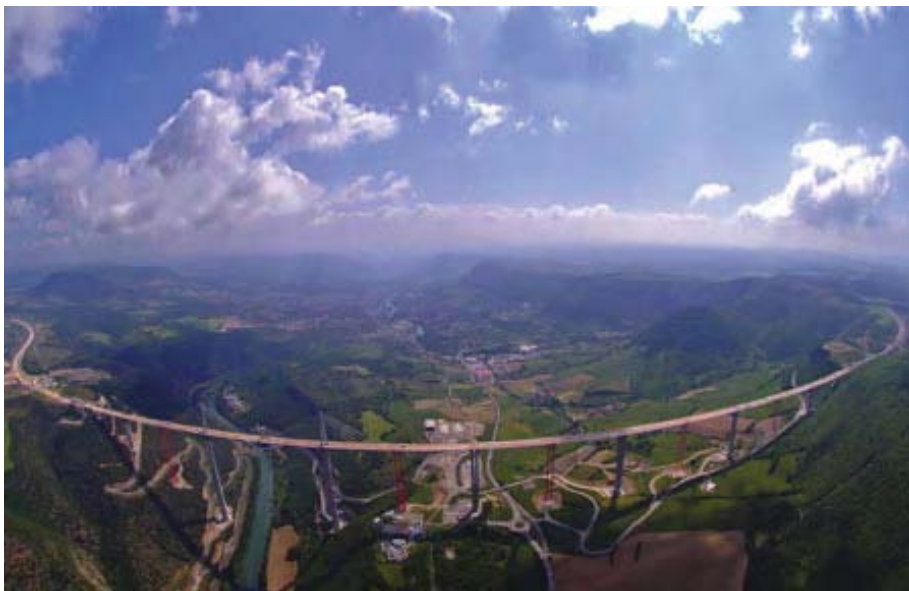
Exhibit 1.22 The Millau Viaduct spans the valley of the river Tarn near Millau in southern France. Completed in 2004, it has the tallest piers of any bridge in the world. The sweeping curve of the roadway provides stability as well as breathtaking views of the broad valley.
