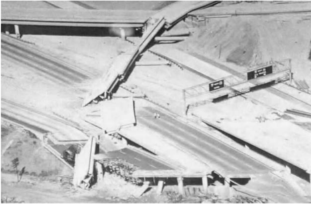
Fig. 2.4 View looking north at the I-5 and I-210 interchange after the quake showing the collapsed South Connector Overcrossing structure (bridge 2) in the center, the North Connector Overcrossing structure (bridge 3) at the top, and bridge group 4 at the bottom. (Photo courtesy E. V. Leyendecker, U.S. Geological Survey.)
