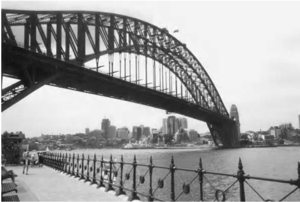
Fig. 4.9 Sydney Harbour Bridge.
