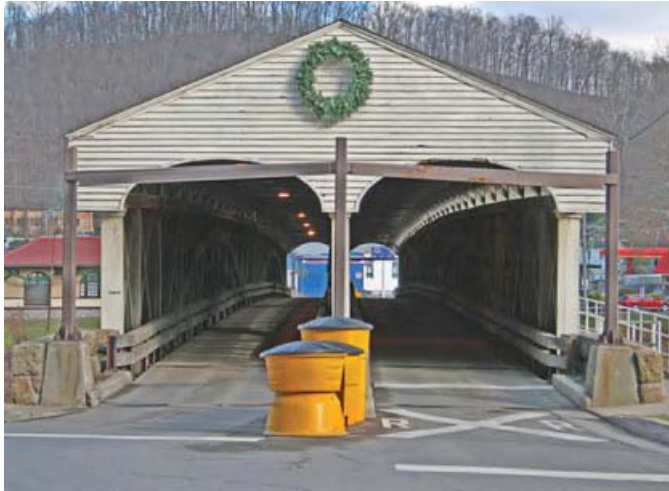
Exhibit 1.3 The Philippi Covered Bridge across the Tygart River Valley near Philippi, West Virginia, was built in 1852. It was used by armies of both the North and the South in the Civil War. In 1934 the bridge was strengthened and is today a part of U.S. 250. It is reportedly the only remaining two-lane “double barrel” covered bridge.
