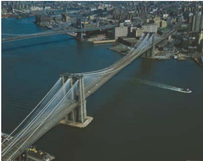
Exhibit 1.4 The Brooklyn Bridge was built 1869–1883 by John and Washington Roebling spanning the East River from Manhattan to Brooklyn, New York (photo looking east towards Brooklyn). When completed, it was the longest spanning bridge in the world and the Roebling system of suspension bridge construction became the standard throughout the world. (Jet Lowe, HAER NY-18-75.)
