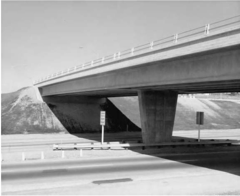
Fig. 3.32 Prestressed girders frame into the side of the supporting pier, eliminating from view the usual cap beam. (Permission granted by the California DOT.)
