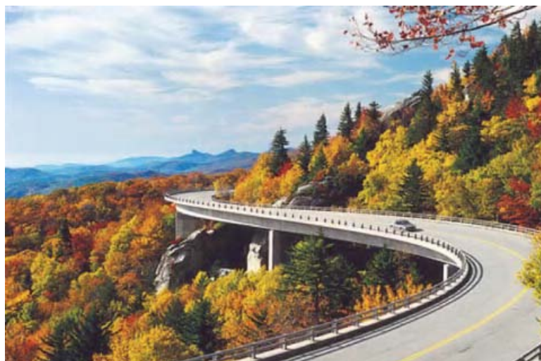
Exhibit 1.14 The Blue Ridge Parkway (Linn Cove) Viaduct, Grandfather Mountain, North Carolina, was built from the top down to protect the environment of Grandfather Mountain. This precast concrete segmental bridge was designed to blend in with the rugged environment.
