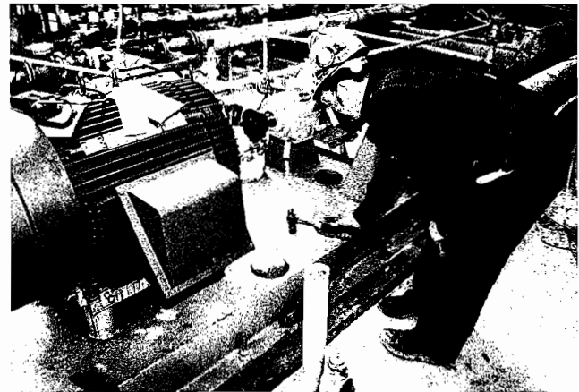
Figure 26. A Hammer Was Used to Test This Baseplate Grout Job for Voids.
