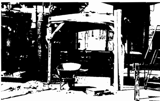
Figure 6. In Hot Weather, Shade the Baseplate for 24 Hours before and 48 Hours after Pouring the Grout.
