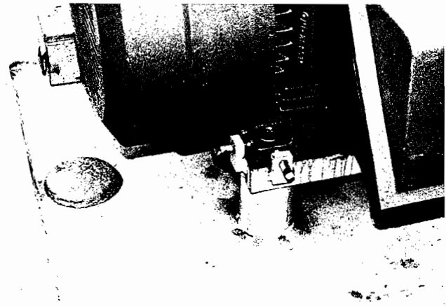
Figure 25. When the Epoxy Grout Begins to Stiffen, Mold a Dome over the Grout Hole to Prevent Forming a Pool for Water.
