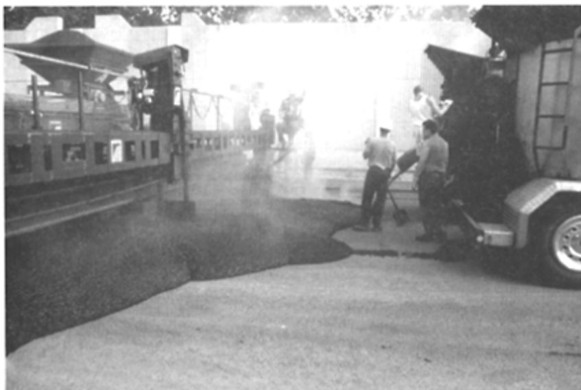
Fig. 8.5 Gussasphalt being fed by mobile stirrer/cookers in front of the screed bar with a feed paddle spreading the material evenly across the width
