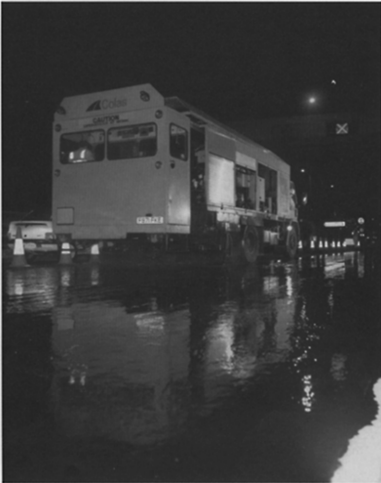
Fig. 11.9 Spraygrip application at Blackwall Tunnel
