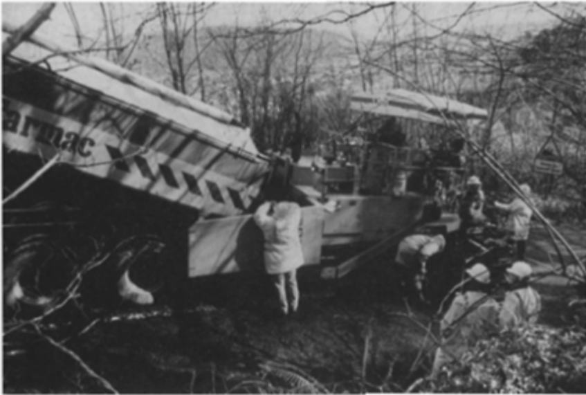
Fig. 9.12 Versatility of SMA—laying operations on the 1:4 gradient Porlock Hill, Somerset
