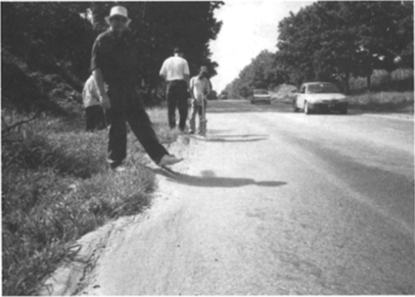
Fig. 6.14 Excessive binder and deformation
