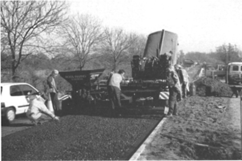
Fig. 5.8 Laying rolled asphalt surface course
