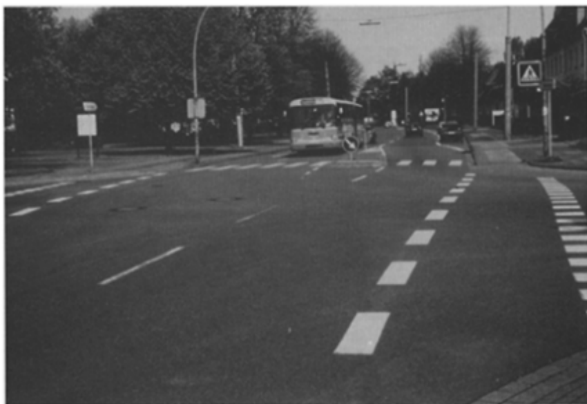
Fig. 9.1 Stone mastic asphalt in Wilhemshaven, Lower Saxony, 24 years old
