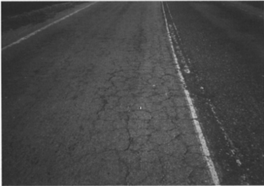
Fig. 6.13 Fatigue cracking
