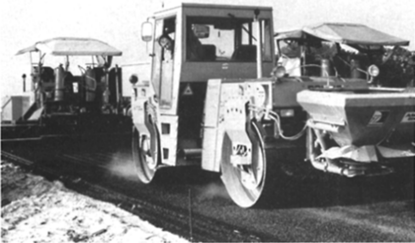
Fig. 9.7 Laying SMA in echelon on the A31 autobahn showing grit application from roller mounted spreader
