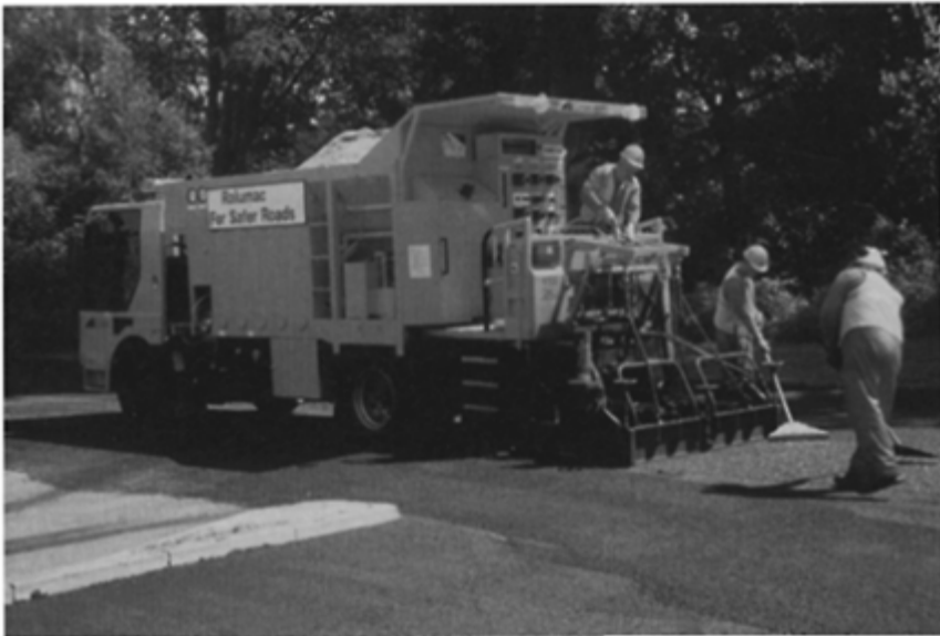
Fig. 11.8 Micro-asphalt applicator with articulated laying box
