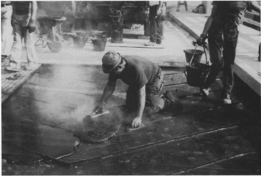
Fig. 8.4 Hand-laid mastic asphalt on a bascule lifting bridge deck, hence the chevron ribs and studs to enhance bond
