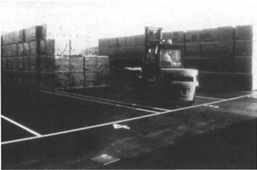
Fig. 9.10 SMA as a tough industrial paving—masterpave on a brick stockyard in Leicestershire
