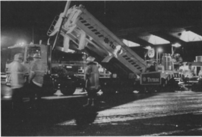
Fig. 9.6 Night laying of masterpave SMA at tool booths of Dartford river crossing to provide deformation-resistant surface
