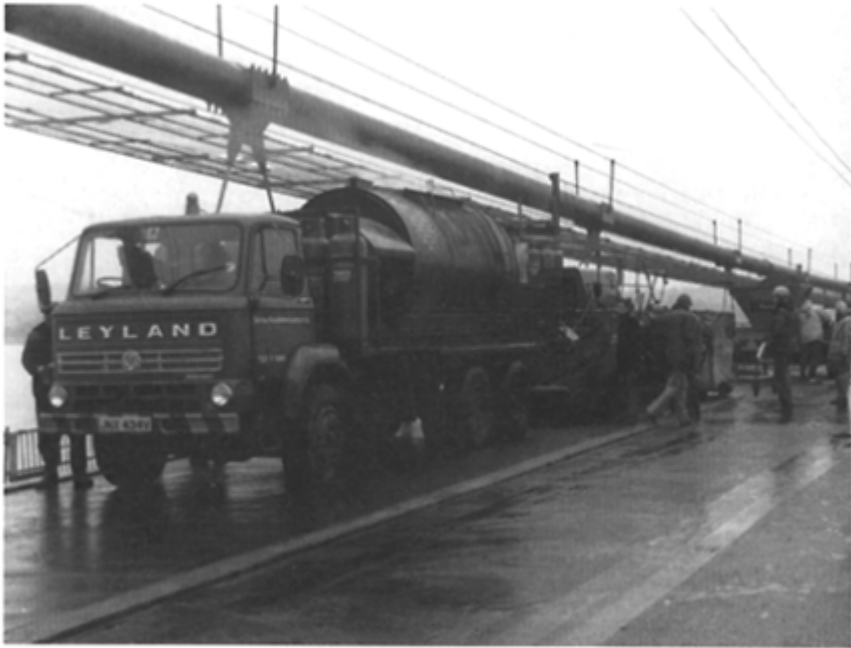
Fig. 8.1 Machine laid mastic asphalt with a stirrer/cooker backing up to the paver, which is heavily shrouded to retain the temperature
