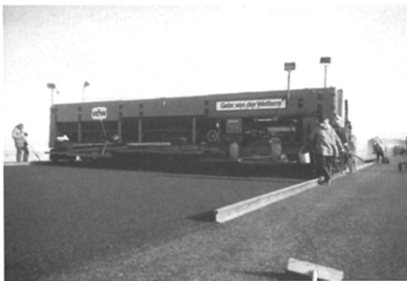
Fig. 8.6 11.5 m gussasphalt screed bar train
