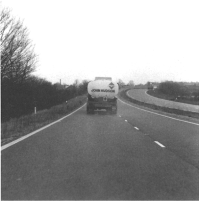
Fig. 7.9 Spray generated by a tanker travelling on porous asphalt
