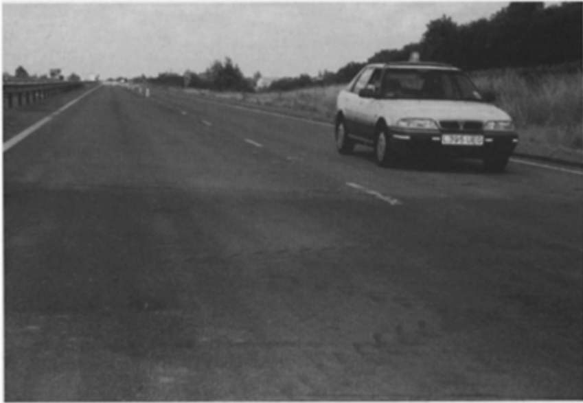
Fig. 10.4 10 mm Safepave after four years' trafficking (background) and 10 mm untrafficked UL-M (foreground)
