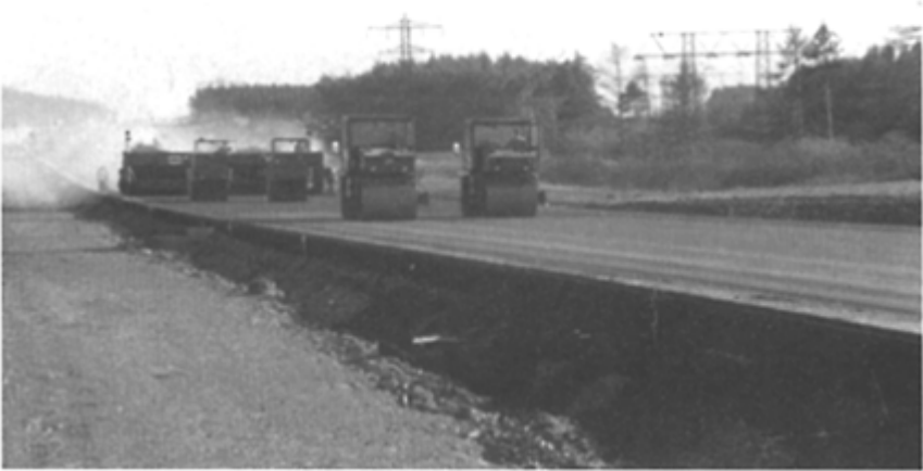
Fig. 8.7 Gussasphalt compaction with both rubber-tyred and steel-wheel rollers in action
