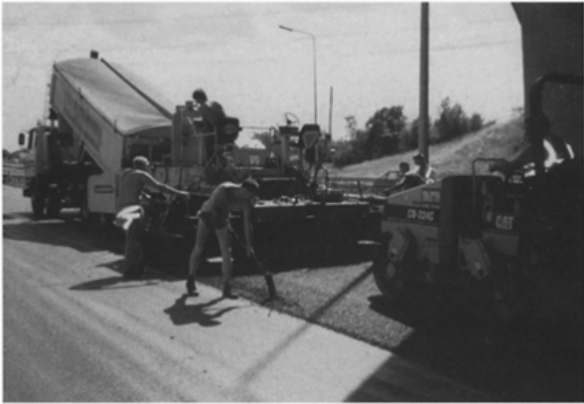
Fig. 10.3 Laying 14 mm SMA over pavement quality concrete
