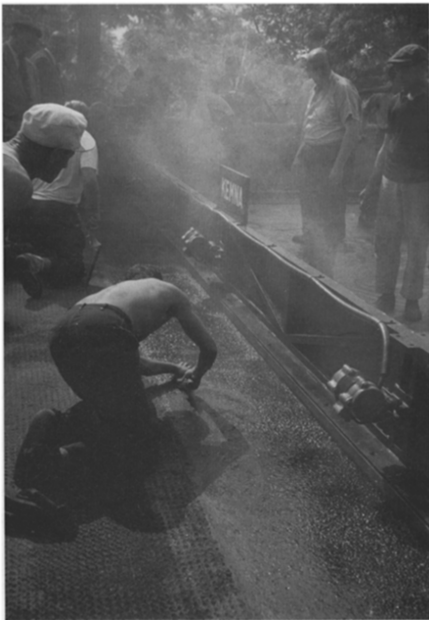
Fig. 8.8 An early application of gussasphalt on the Avus motor racing circuit in 1955 showing hand finishing and the effect of crimping rollers
