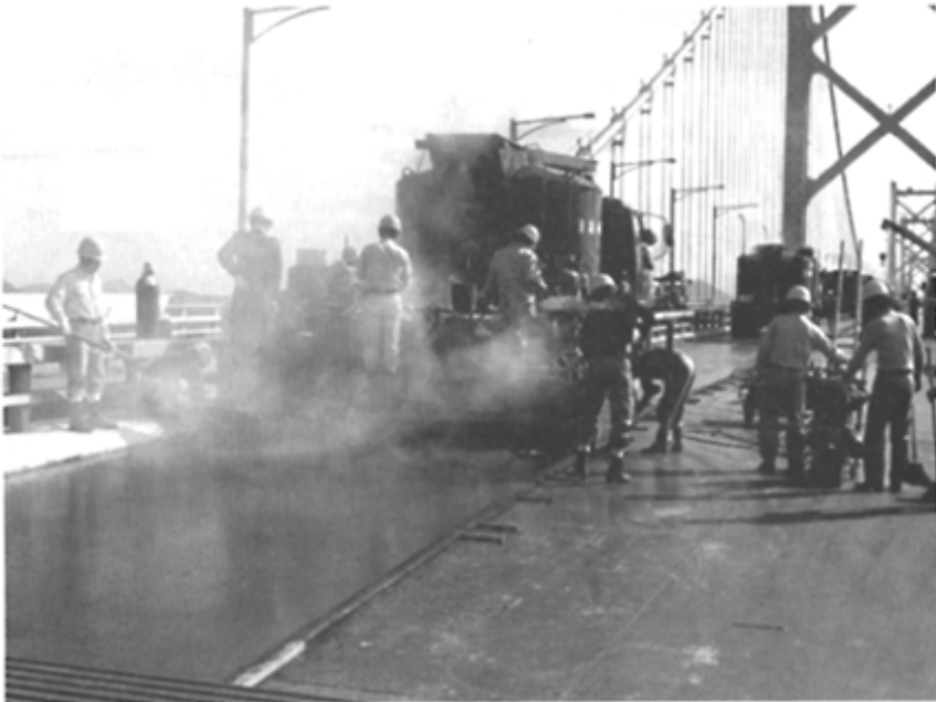
Fig. 8.9 Application of gussasphalt at Honshu-Shikoku, Japan
