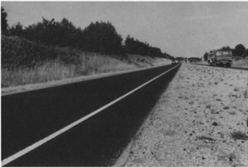
Fig. 9.9 SMA as a thin surfacing—25 mm thick masterpave on the A148 Holt Bypass, Norfolk
