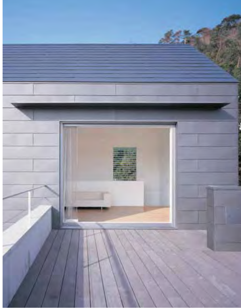
Above: The terrace in front of the living room, located above the bathroom wing, is covered with strips of water-resistant jarrah. A box-like structure on the terrace, part of the low wall that surrounds the terrace, houses a water faucet.
