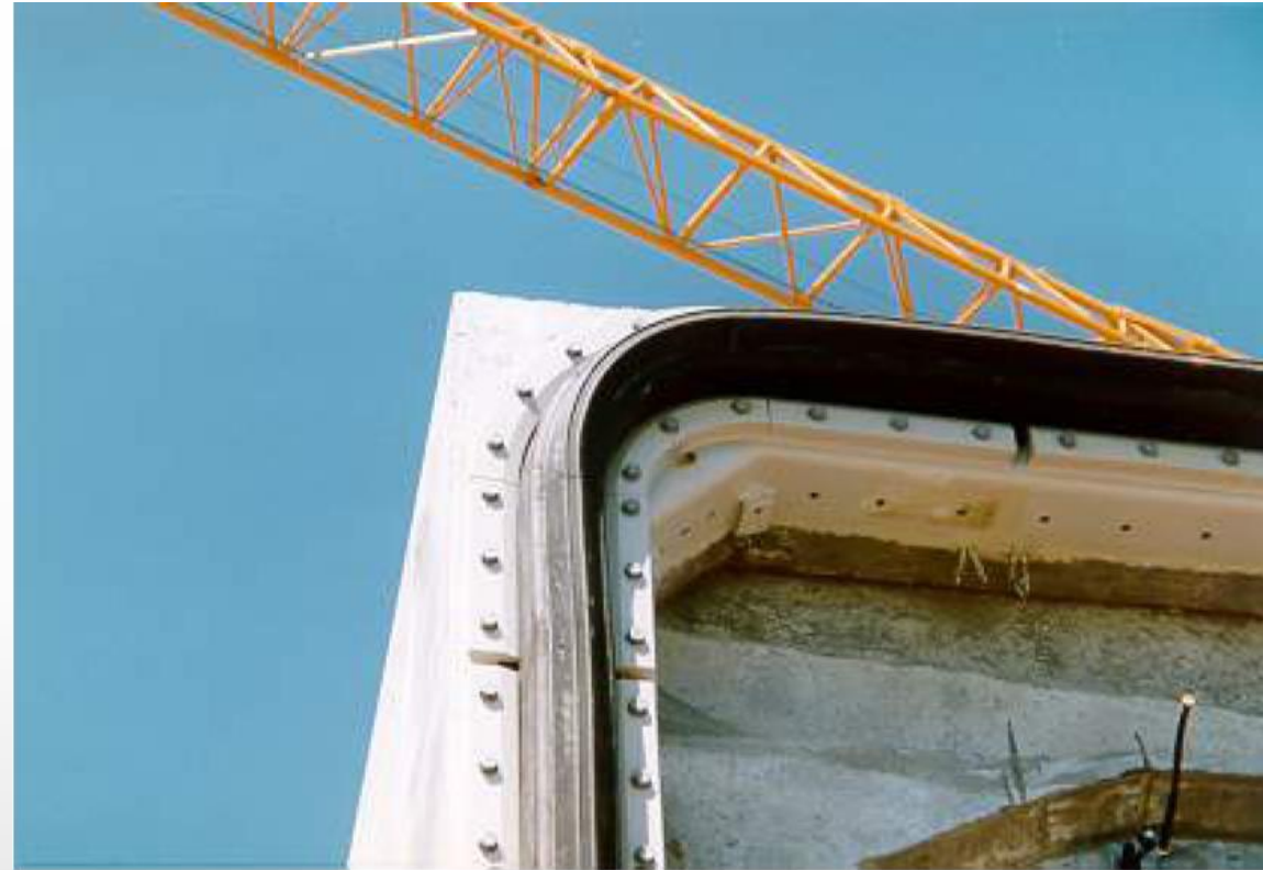
Photo: Top corner of mounted Gina frame – Øresund tunnel
