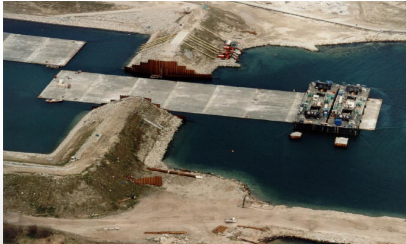
Figure 9 Completed tunnel element exiting the launch basin
