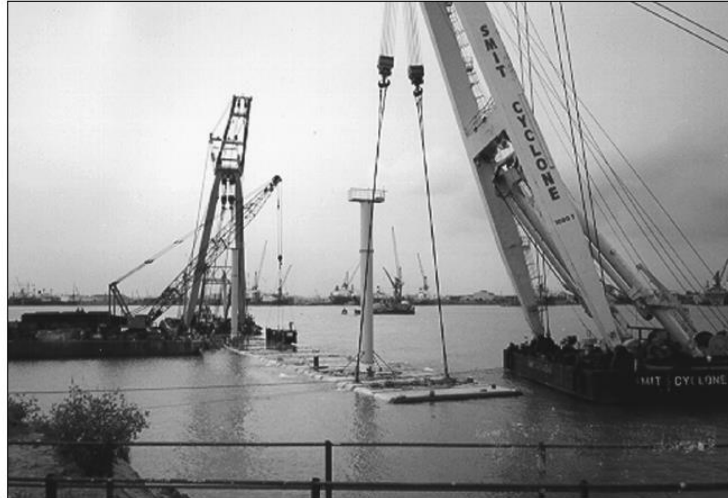
Figure 9. Immersion of immersed tube element using marine cranes
