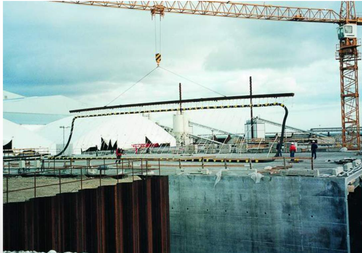
Photo: Hoisting of Gina frame – Øresund tunnel
