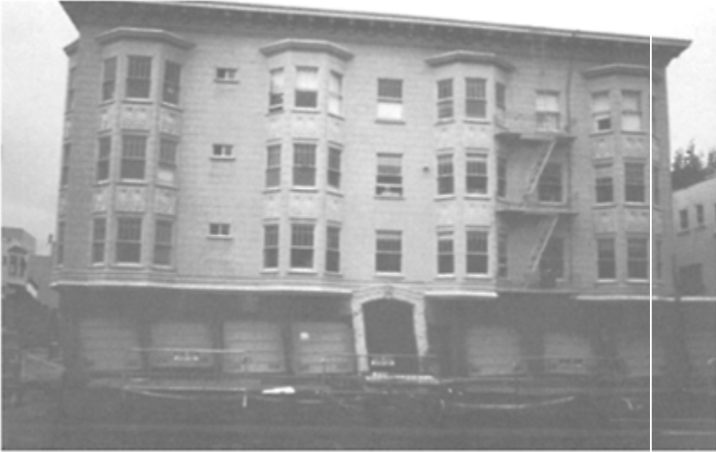
FIGURE 18.8 Typical soft-story apartment building in the Marina District of San Francisco following the 1989 Loma Prieta earthquake (courtesy of Y.Bozorgnia).
