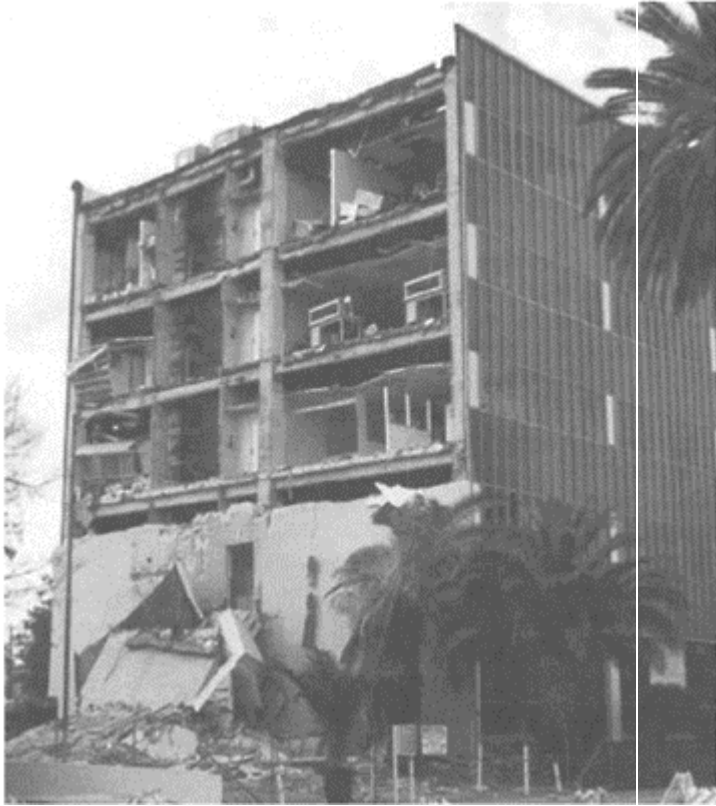
FIGURE 19.6 Collapse of building's exterior wall during the 1994 Northridge, CA, earthquake. (Photo courtesy of Yousef Bozorgnia.)
