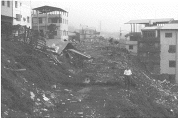
FIGURE 3.3 Damage from surface rupture on the Chelungpu reverse fault in Fengyuan City, Taiwan, accompanying the September 21, 1999, Chi-Chi earthquake of M 7.6. Photo taken 5 months after the earthquake. The cleared area on the upthrown side of the fault was formerly covered with buildings that were completely destroyed, with loss of life; the remains of these structures were subsequently removed. Damage to buildings on the downthrown side of the fault (far right) was severe, but the buildings were not totally destroyed. If an Alquist-Priolo setback had been in effect prior to development of this area, losses of life and property would have been greatly reduced. Photo by Robert Yeats, reproduced from Yeats
