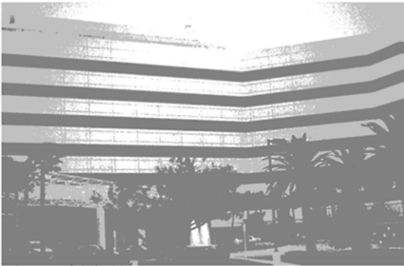
FIGURE 11.11 University of Southern California Teaching Hospital: base-isolated building affected by the 1994 Northridge, California, earthquake.
