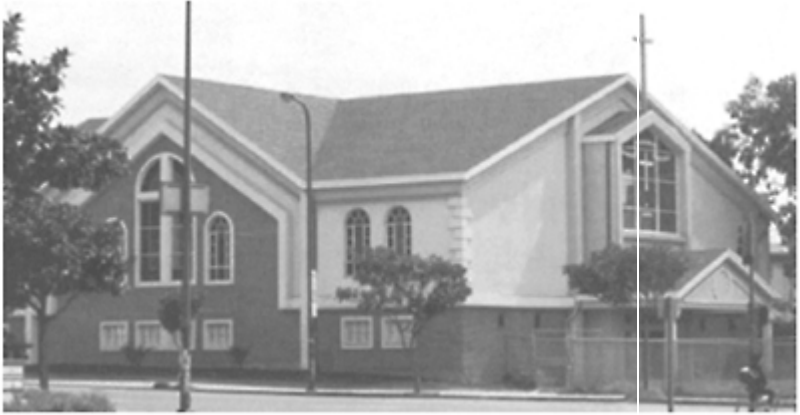
FIGURE 18.5 Existing wood frame building at the corner of Ashby and Adeline Streets in Berkeley, CA, public use.
