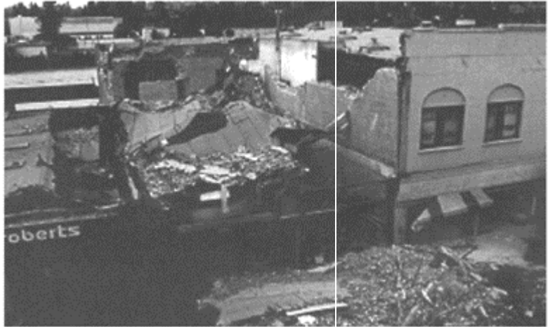
FIGURE 17.7 Collapsed unreinforced masonry buildings in Santa Cruz after the Loma Prieta earthquake. (Photo by the International Masonry Institute.)
