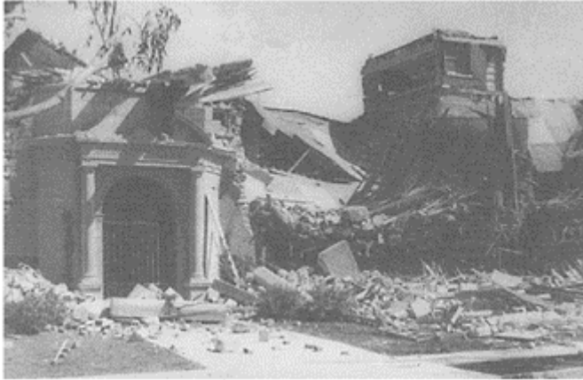
FIGURE 1.3 The 1933 Long Beach, California, earthquake—damaged Jefferson Junior High School. Photo from Steinbrugge Collection, National Information Service for Earthquake Engineering of the University of California, Berkeley.
