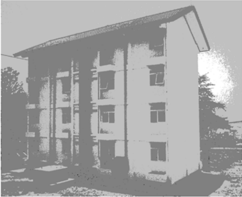
FIGURE 11.3 UNIDO demonstration base-isolated building in Indonesia.
