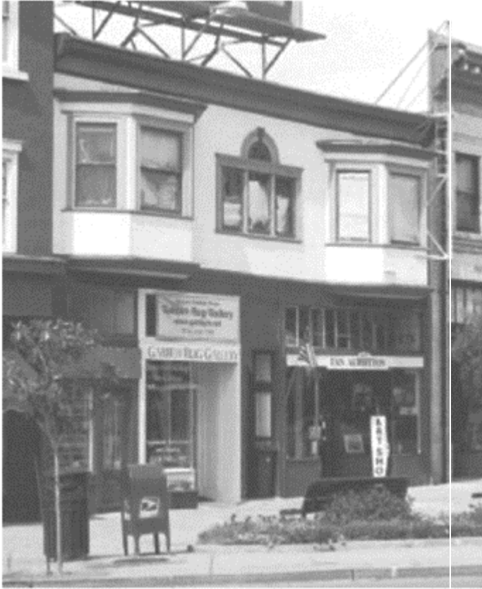
FIGURE 18.4 Existing wood frame building at the corner of Ashby and Adeline Streets in Berkeley, CA, mixed commercial and residential use.
