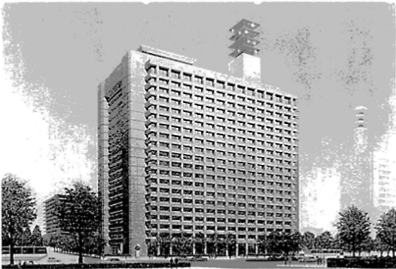
FIGURE 10.13 Central Government Building (courtesy of Kume Sekkei).
