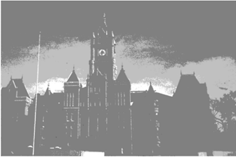
FIGURE 11.4 City and County Building, Salt Lake City, Utah: the first historic building retrofitted by base isolation.
