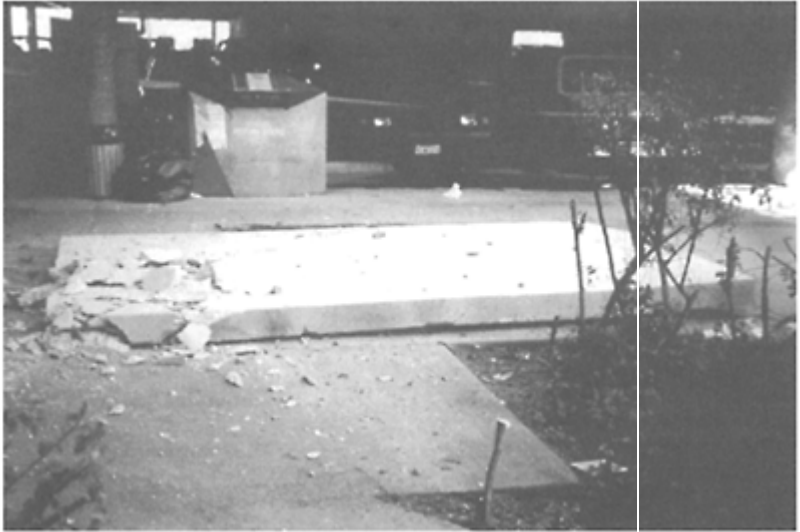
FIGURE 19.5 Fallen precast element from parking garage, responsible for death of a student during the 1987 Whittier Narrows earthquake in Los Angeles, CA, area. (Photo courtesy of Narendra Taly/California State University, Los Angeles; reproduced with permission of Earthquake Engineering Research Institute.)
