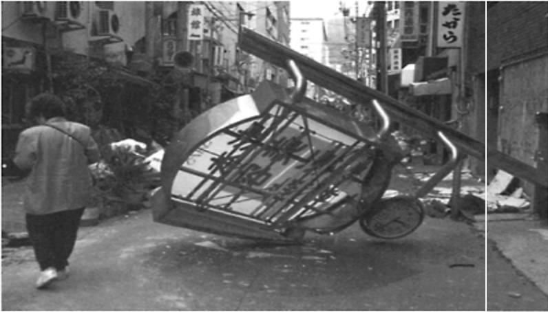
FIGURE 19.1 Collapse of signboard on street of Kobe, Japan, during the 1995 Great Hanshin earthquake. (Photo courtesy of Chris Arnold/Building Systems Development, Inc.)
