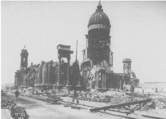
FIGURE 1.1 The 1906 San Francisco earthquake—damaged San Francisco City Hall, looking north from Larkin and Grove streets toward City Hall (behind Majestic Theatre). Photo from Steinbrugge Collection, National Information Service for Earthquake Engineering of the University of California, Berkeley.
