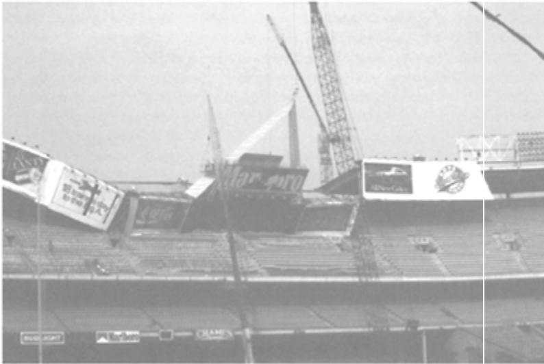
FIGURE 19.8 Collapse of 17-ton Scoreboard at Anaheim Stadium (black object below stadium's A logo and sur-rounded by billboards) during the 1994 Northridge, CA, earthquake.
