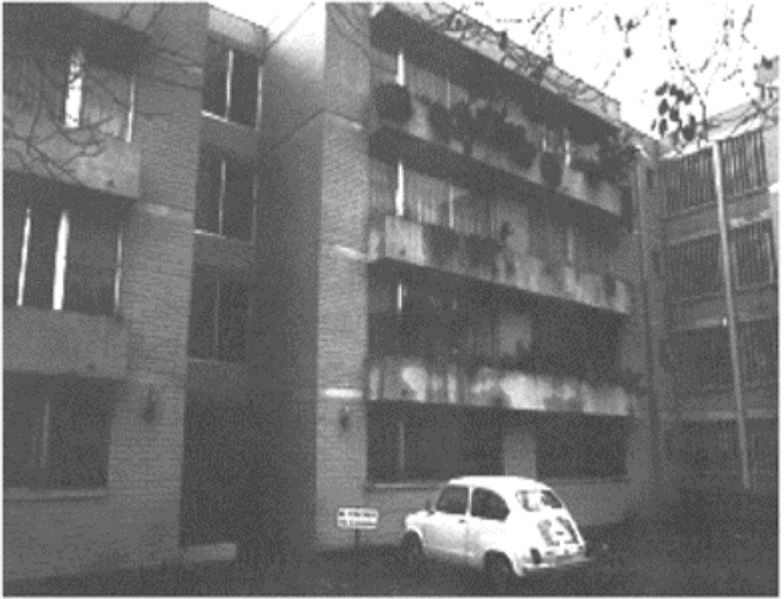
FIGURE 17.13 U.S.-type masonry building after Santiago, Chile, earthquake of 1985. (Photo by R.E.Klingner.)
