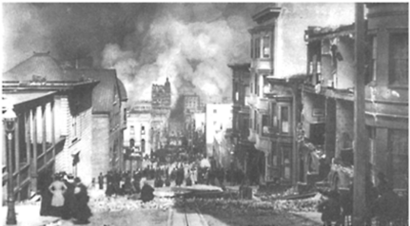
FIGURE 17.4 Damage from the San Francisco
