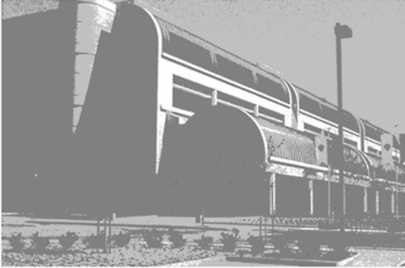
FIGURE 11.1 Foothills Community Law and Justice Center, Rancho Cucamonga, California: the first base-isolated building in the United States.
